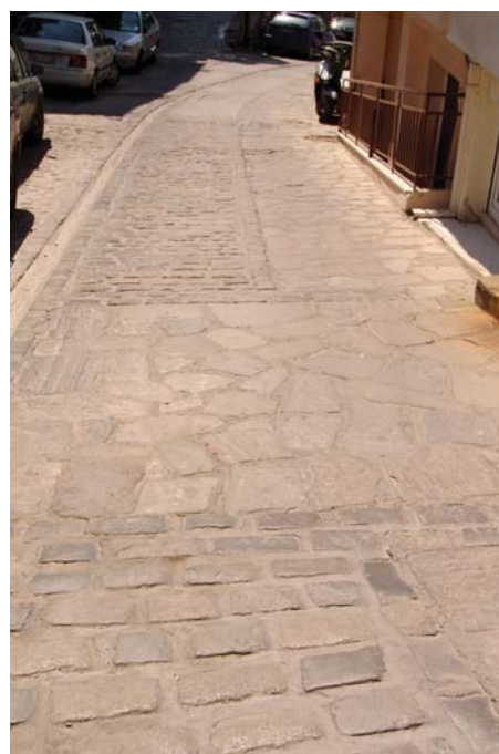
Picture 4: Street pavement in Ano Poli (city of Thessaloniki).
