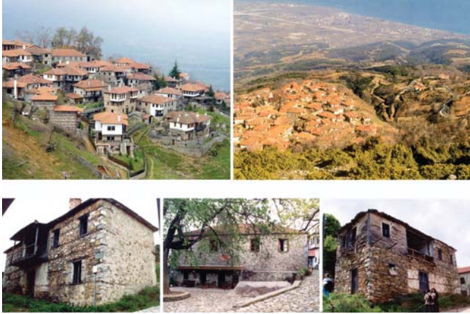
Actual views of the settlement.
