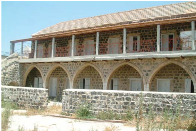
Beth Shami Looking West
