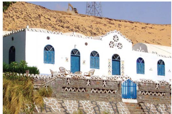
Fig(1) Samples of Traditional crafts used in buildings in Aswan.
