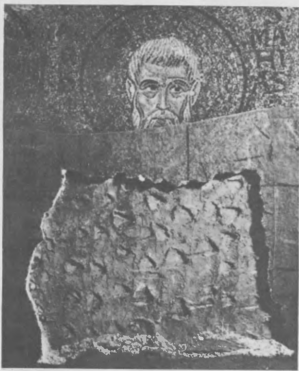
Fig. 3 - Removal of the mosaic and of the first layer of the support, revealing the second layer with its indentations for holding the mortar more securely
