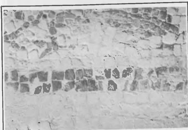
Fig. 10 - Mosaic from the east of France transferred to a slab of cement uninsulated from humid soil underneath. The efflorescence of salts, evident here, very rapidly brings about the destruction of the mosaic
