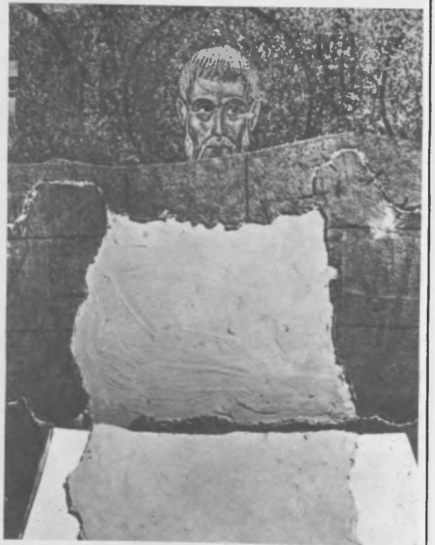
Fig. 5 - The new mortar bed is ready to receive the mosaic
