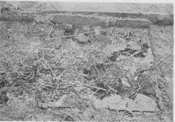
Fig. 14 - Saint-Paul-les-Romans, removing the cement slabs, we discover a network of roots and tunnels dug by field mice
