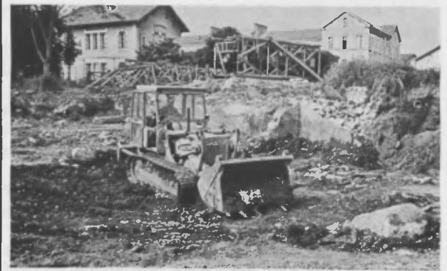
Fig. 4 - Perigueux, the destruction of the remains of an antique polychrome mosaic, 1977
