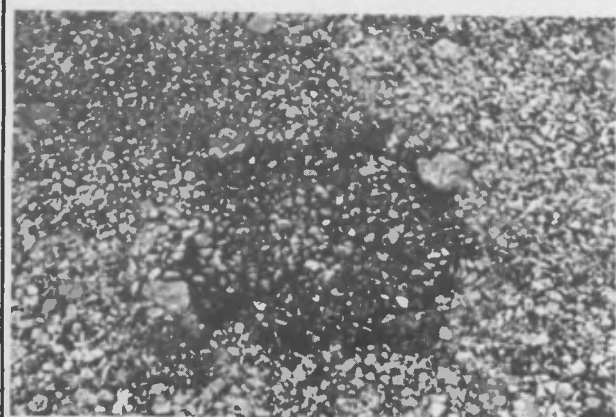
Fig. 2 - Section of pavement in the process of treatment
