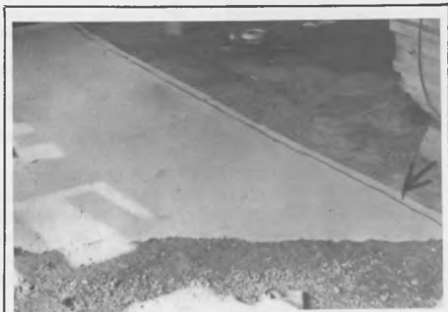
Fig. 4 - A glued piece of mosaic, ready to be separated. At the end, a glued strip of cotton at the edges of adjacent sections
