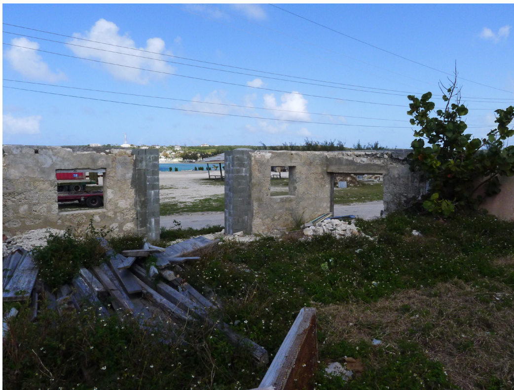
Figures 104 to 108 (from top left clockwise): concrete cistern on the south facade of the jail building; upper and lower terraces of the jail complex; arrow-headed strap hinge on discarded right hand cell door; interior view of left hand cell; view of the northern portion of the jail yard showing the surrounding stucco and concrete and rubble walls surrounding the yard.
