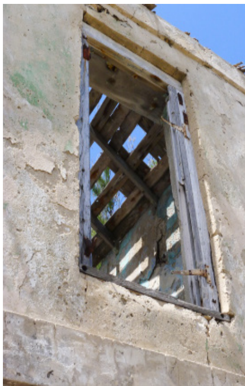
Figures 62 to 67 (upper left, clockwise): First floor showing support structures; detail of the support members; detail of iron strap hinge fastened to wooden window casing on second floor window; window with full wooden shutter on southeast facade; window opening on second floor with shutter strap hinges in place and full wooden window casing; northeast facade from second floor stair landing showing double wooden window casings and remnants of strap hinge fasteners.
