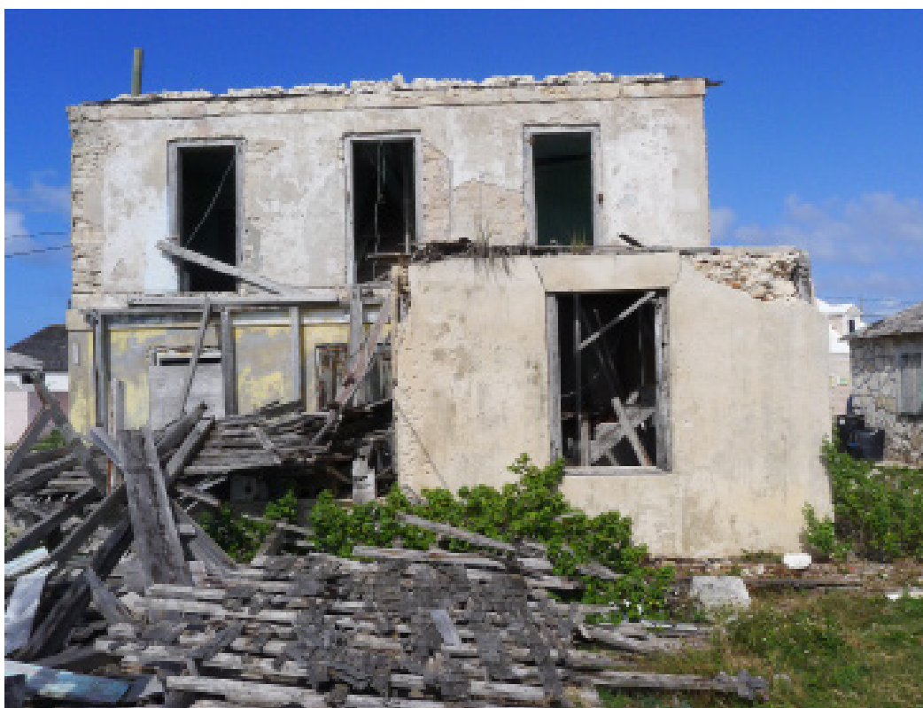
Figures 73 to 77 (from top left clockwise): west facade; detail of mortise and tenon and peg construction of the rear addition; detail of the balcony and openings to the second floor: stairs to the third floor are visible through the central opening; east facade; southern facade showing wooden rubble from the collapsed roof and addition.
