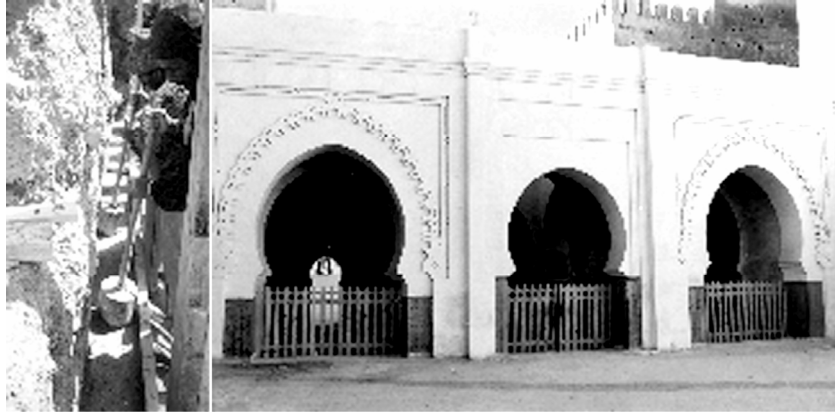
Figure 23.4 Restoration of historic walls
