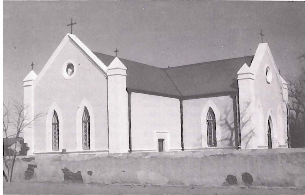
Fig. 1. The church at Bethany after restoration. (Photo: H. Gous)
