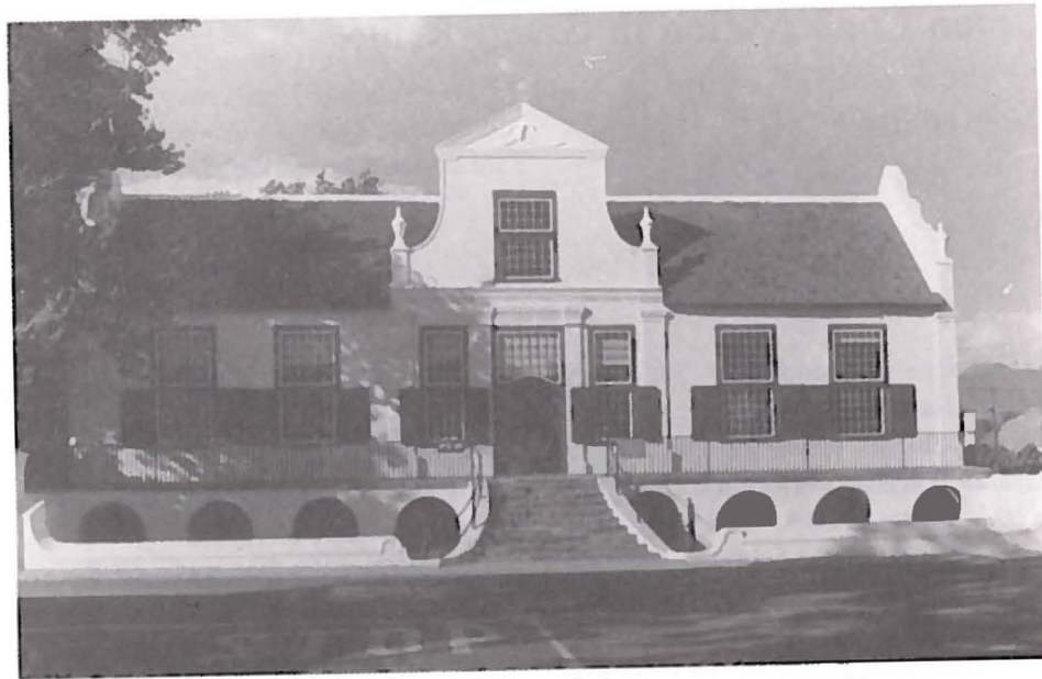
Fig. 1. The Old Dutch Reformed Church Parsonage (Reinet House), Graaff-Reinet, completed in 1812. (Photo: Peter Whitlock)
