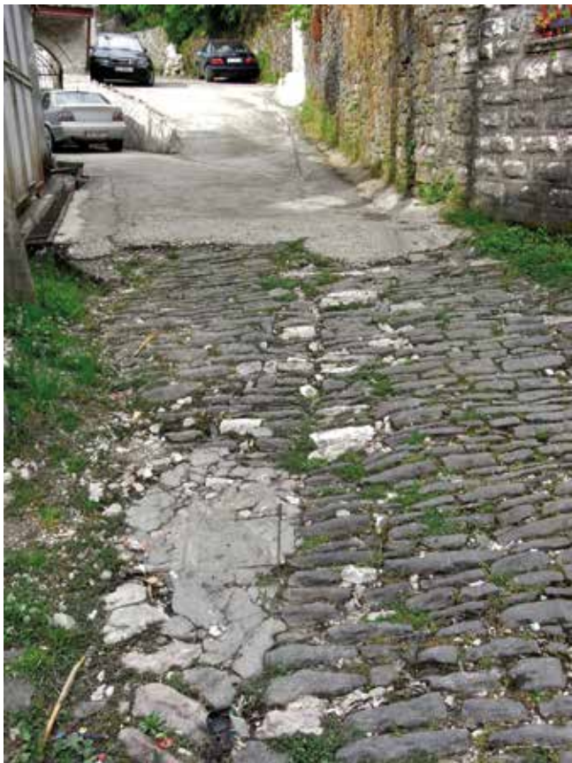
Fig. 8: While the ICOMOS Mission Report states, “A substantial financing of 85.000.000 lekë has also been allocated for the reconstruction of roads in the historic centre”, these funds have actually been used to cover historic cobblestone pavements with concrete. Photo: Stephan Doempke
