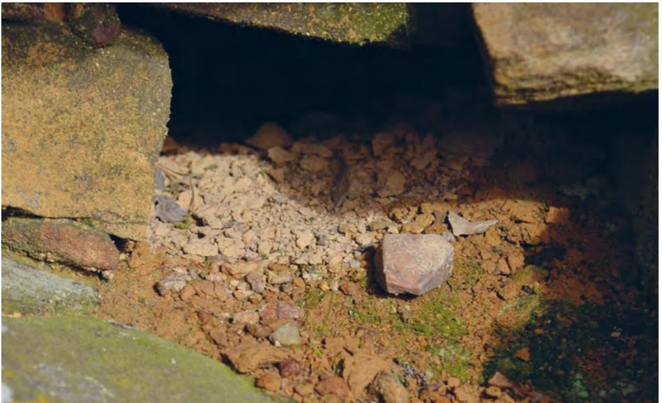
*Fig. 4 The remains of clay mortar visible in the wall core at Mervinslaw.*
