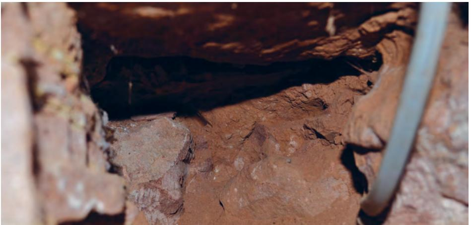
*Fig. 5 This opening in a wall has revealed the clay-bonded wall core.*
