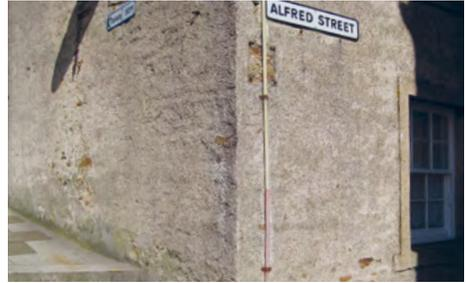
*Fig. 2 A clay-bonded wall in Stromness retaining the original lime harl that protects the underlying clay mortar. Masonry walls built using clay often do not differ in external appearance from lime-bonded walls.*
