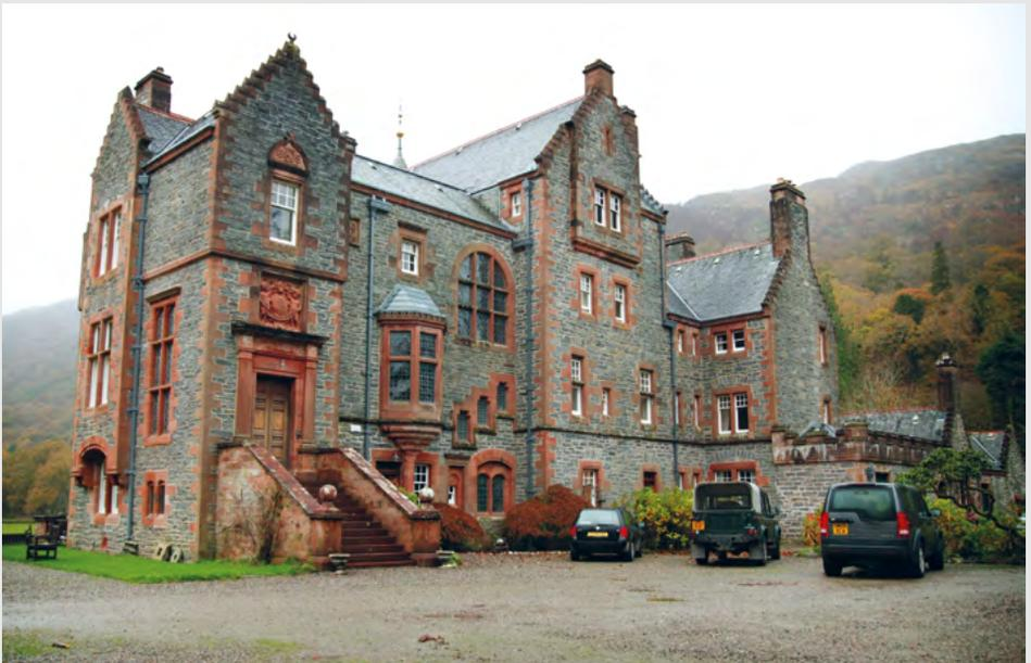
*Fig. 1 This 19th century mansion was constructed using clay in the wall core and pointed with lime externally.*
