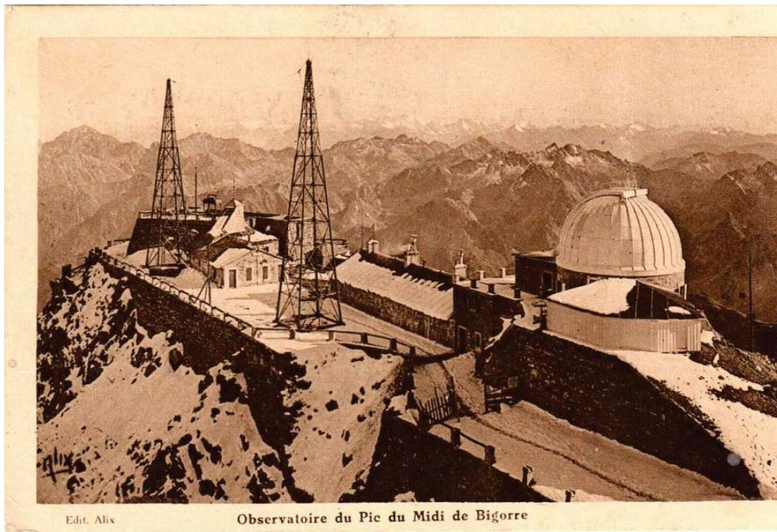
**Fig. 9.30** The Pic du Midi Observatory in 1925. The two TSF aerials have been placed on the summit. The crumbling northern ravine started to be reinforced. Photo © Alix, Fond Eyssalet
