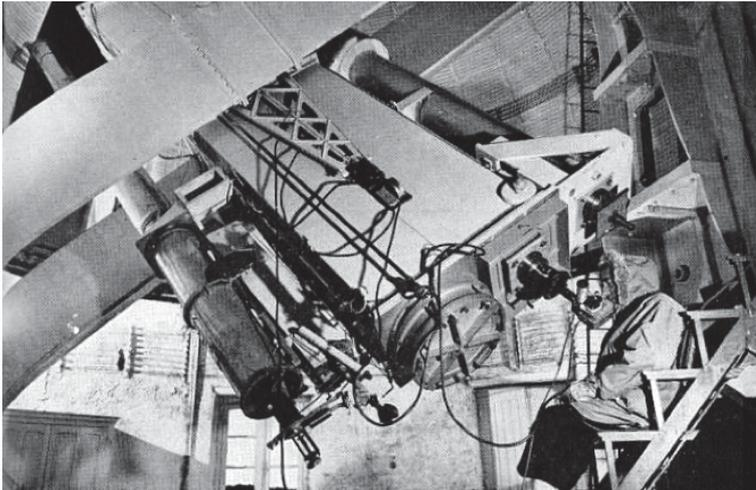
**Fig. 9.31** The refracto-reflector, named the Baillaud Telescope, under the Baillaud dome in 1947. It was with this instrument that the main planetary and solar observations from 1950–60 were made. The instrument was dismantled in 1970 and replaced by a coronagraph. Photo © Régie du Pic du Midi and Observatoire Midi Pyrénées
