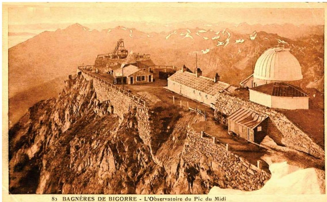
**Fig. 9.29** The Pic du Midi Observatory just after the First World War. We can see the Baillaud dome and observatory building on the right, built between 1906 and 1908. The north terrace crumbled following several years without maintenance (1920). Photo © Régie du Pic du Midi and Observatoire Midi Pyrénées
