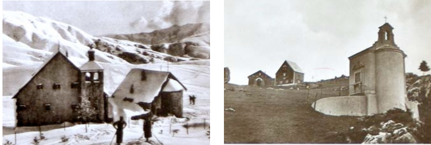
Figure 3-4. Mino Fiocchi – Nino Castelli Lodge; Valsassina, 1928-1931. View of the the lodge and the Bettini Chapel. Photo taken in those years. Fiocchi archives.
