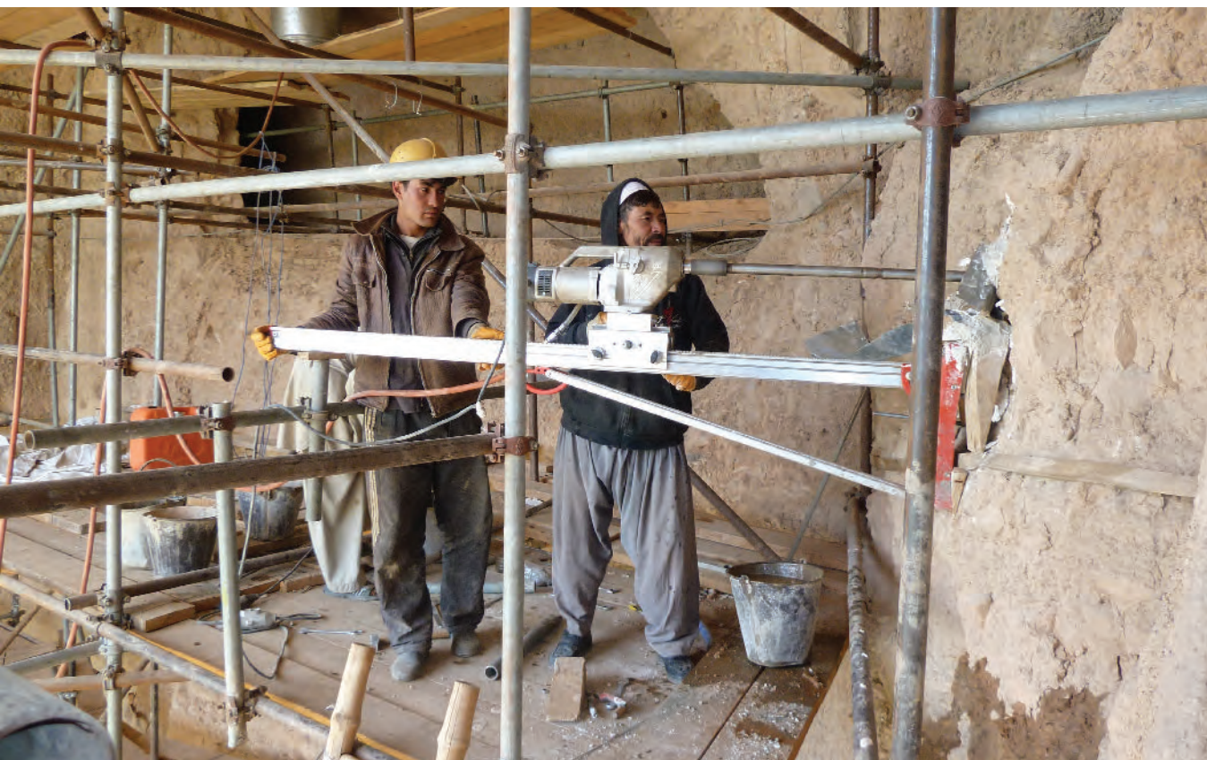
Conservation work at the eastern Buddha, 2009/10, drilling the holes for the anchors © UNESCO/Bert Praxenthaler
