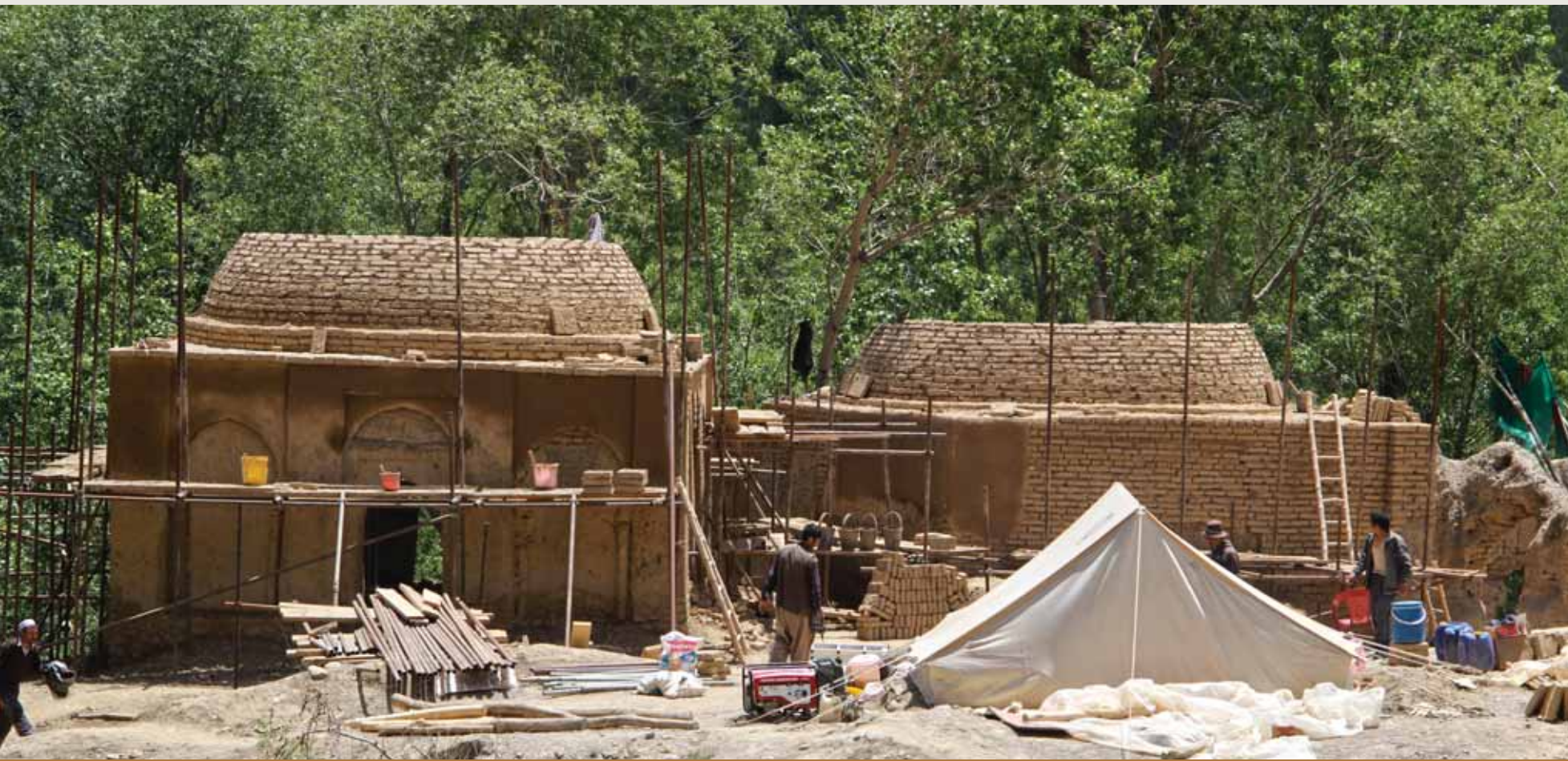
Mausoleums A & B, rebuilding of the cupolas © UNESCO/Mujtabah Mirzai
