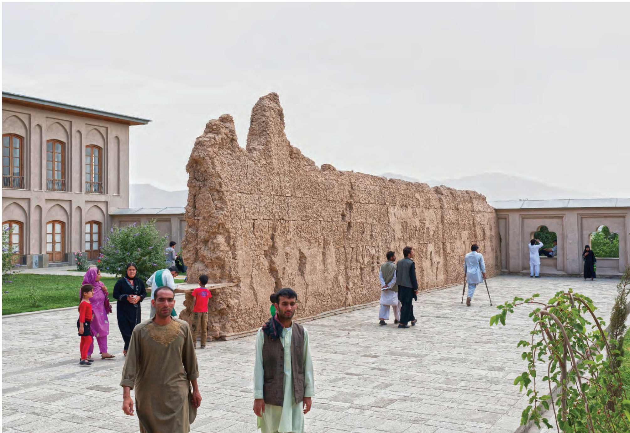
One of the installations that formed part of dOCUMENTA (13) presence in Kabul was represented by the erection of a pakhsa (compressed mud and straw) wall in the courtyard of the Queen's Palace at Baghe Babur. This traditional building technique is used throughout Kabul and the provinces, especially in the construction of traditional Qala's (fortified walled homes) although is becoming less common in the city. This example was built and left to naturally degrade over the course of the event-100 days © dOCUMENTA (13)
