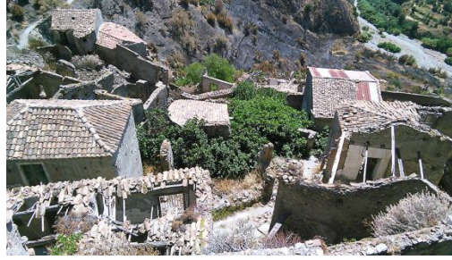
Fig.2- Partially collapsed houses in Pentedattilo.
