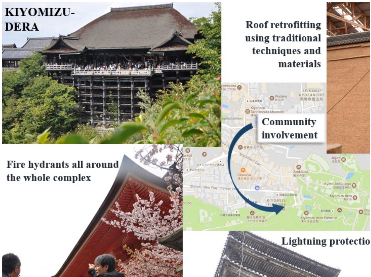
Fig.1- Scheme of Kiyomizu-dera main good practices highlighted during the TDD: earthquake-resistant architecture, fire fighting system and lighting protection, landslide stabilization and monitoring, and community engagement. Some teams requested further information, such as slope stabilization measures or activities to engage the local community, to share with their project partners once back in their respective countries. (Photos: Barbara Minguez Garcia)
