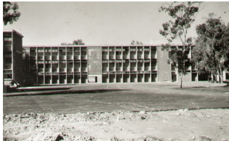
Fig.4– Lefkoshia Turkish Boarding School for Girls (Nicosia, Cyprus) 1962, architect: Ahmet Bahaeddin (Docomomo Cyprus, 2014)
