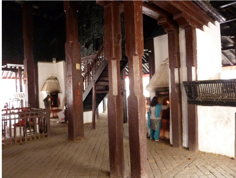
Fig.2– Local Kathmandu residents making offerings at the shrines in Kasthamandap prior to its collapse. The large central posts are reputed to have been cut from a single tree (Forbes, 2014).
