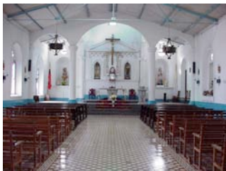
Figure 3. Internal view of the temple
