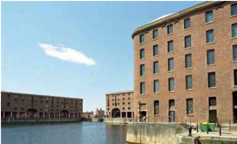
Fig. 8: Albert Dock Warehouses (Liverpool) opened for storage of imported goods brought by ships in 1846. It was the first structure in the UK to be built entirely of cast iron, brick and stone. By the turn of the twentieth century only 7% of ships using the Liverpool port were sailing ships and Albert Dock was eventually closed in 1972. The dock's silted up and the warehouses fell derelict. Planning for the dock's regeneration began in 1982 and was completed by 1988. The complex forms part of the Liverpool Maritime Mercantile City world heritage property and the UNESCO inscription details identify the skilful adaptation of the warehouses to new uses, including the Tate Liverpool Art Gallery, Maritime Museum, International Slavery Museum, Beatles Story Museum and bars, restaurants, shops, offices and hotels. Repairs and alterations required to convert the warehouses to the new uses were kept to a minimum and have not significantly affected their authenticity and integrity. It is the largest group of Grade I (highest quality) listed buildings in the UK and is the most visited multi-use attraction in the UK outside of London.
