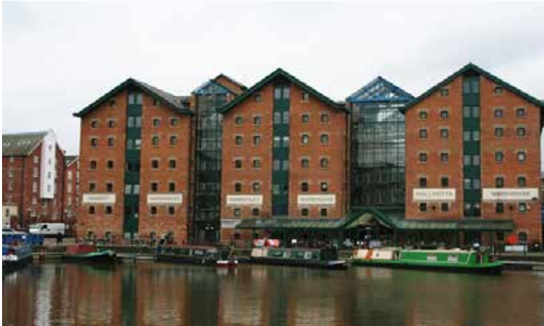
Fig. 3: Gloucester Docks Warehouses and Mills. The warehouses and mills at Gloucester were mainly built in the period 1840 – 1870 for the storage and processing of imported grain. After a long period of stagnation, in which many of the buildings were threatened with demolition, a period of rehabilitation and regeneration of the warehouses and dock area commenced about 12 years ago and continues today. Many of the former warehouses and mills have now been converted to other uses, including residential apartments and a mix of waterside museums, bars, cafes, restaurants and shopping plus new communal squares, walkways and public art.
