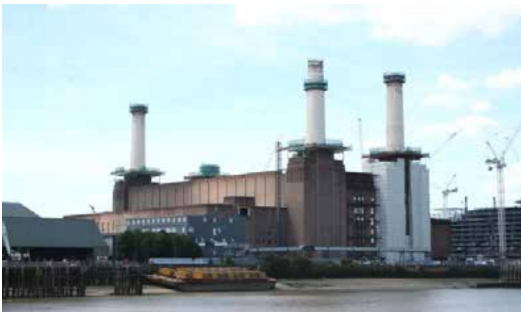
Fig. 2: Battersea Power Station (London) is a decommissioned coal-fired power station located on the south bank of the River Thames in London comprising two individual power stations (built in the 1930s and 1950s to an identical design, providing the well known four-chimney iconic structure, in the brick-cathedral style of power station design like Bankside). The station ceased generating electricity in 1983, but has become one of the best known landmarks in the UK and was listed as a heritage site in 1980 and to a higher II* grade in 2007. There have been numerous proposals and attempts to redevelop the site since, and eventually one is now in progress (since 2012), using the Power Station as the central focus of the regenerated 40-acre site, which will include shops, cafes, restaurants, art and leisure facilities, office space and residential accommodation (over 800 homes). The plan includes the restoration of the historic Power Station itself, the creation of a new riverside park and walk and the creation of a new High Street to link to new underground stations. Work commenced on the power station itself in 2013 including the restoration of the art deco structure internally and externally, reconstruction of the chimneys, and refurbishment of the historic cranes and jetty as a new river taxi stop.
