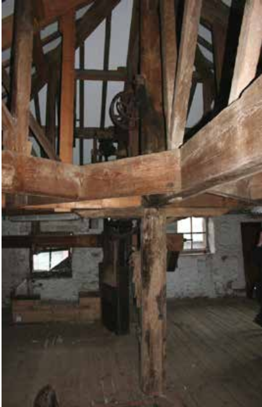
Fig. 13: Warwick Bridge Corn Mill (Cumbria) an early 19th C water powered corn mill, significant for its intact machinery and waterwheel (dated 1843) remained in operation until 1989, but has been on the Heritage at Risk Register since 1999 (15 years). The roof has been repaired by the owner but the overall condition is poor. Options for a more comprehensive restoration to secure a sustainable use by the North of England Civic Trust (NECT) are under discussion at the present time. NECT was awarded a grant of £1,379,300 (GBP) from the Heritage Lottery Fund (HLF) in June 2015 towards its ambitious £2 million (GBP) project to bring the building back into operation as a working mill and artisan bakery providing specialist courses in bread-making with associated crafts, and as a resource for learning in connection with the national school curriculum and accredited conservation courses. The building has been bought by NECT for this working project with the assistance of a low interest loan from the Architectural Heritage Fund (set up as part of the UK's contribution to the European Architectural Heritage Year campaign 1975 to assist such rescue projects). Work should commence in late 2015. Had this option not been realised the property has had the benefit of planning permission to convert the building to residential use, but this would have resulted in the loss of the machinery.
