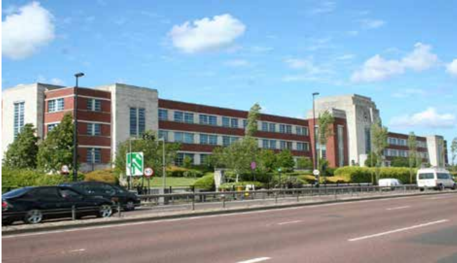
Fig. 6: The Wills Building (Newcastle upon Tyne) was a former cigarette factory built in the Art Deco style in the late 1940s for WD & OH Wills. After the factory closed in 1986 it was listed, but stood empty for a number of years and was in a semi-derelict state at the time of purchase. Various schemes were put forward after many people had called for its reuse, including conversion into a hotel, but its 10 minute location from the city centre meant there was scope for residential use. The rear section of the factory complex was demolished as the buildings were too impregnated with nicotine to be cost-effectively restored. The main building was converted into luxury residential apartments with its exterior carefully restored, it re-opened in 1999. Modern housing was built on the “brownfield” land to the rear, which helped fund the works.
