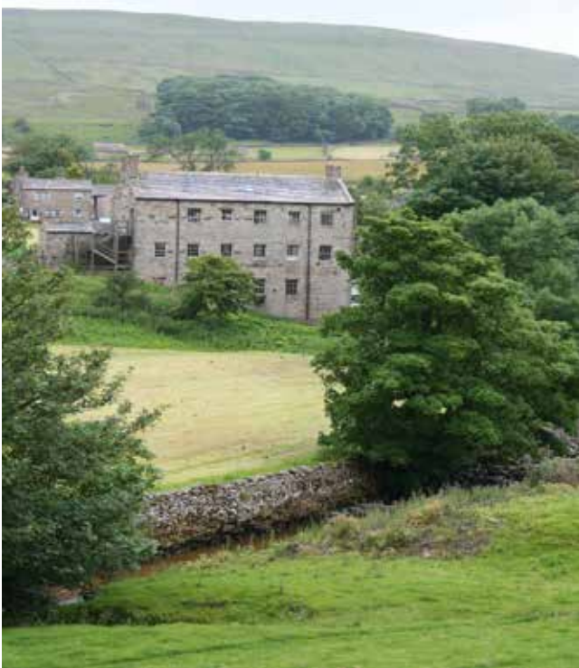
Fig. 12: Gayle Mill (North Yorkshire - rural location) is a 19th century sawmill which has been restored by the North of England Civic Trust and is now open to the public. Gayle Mill, in the Yorkshire Dales National Park, was successively used as a water-powered cotton mill, woollen mill, sawmill and hydroelectric power station. It was eventually rescued and restored by the North of England Civic Trust (NECT) with funding from Heritage Lottery Fund, English Heritage and the Yorkshire Dales National Park Authority. In 2004 the mill won second place in the UK BBC2 television series 'Restoration' and is now managed by the volunteer-led Gayle Mill Trust, but its ownership is retained by NECT.
