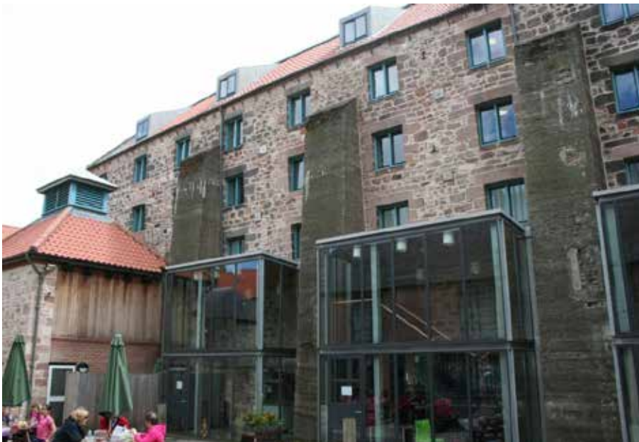
Fig. 11: Dewars Lane Granary (Berwick upon Tweed) an 18th century (1769) granary in use for storing and conditioning grain and, more recently, linseed and grass seed, until 1985. Berwick-upon-Tweed Preservation Trust led a £5 million (GBP) project to restore the building and secure its future as a multi-use facility incorporating exhibition space, a heritage interpretation centre, a bistro, youth hostel and meeting rooms. It opened in 2011. This scheme was cited in the English Heritage Publication entitled “Constructive Conservation”.
