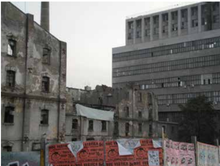
Fig. 8: The First Steam Mill, 1902, before reconstruction (Photo: M.Roter-Blagojević).
