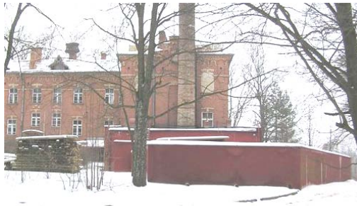
Figure 4. An oil heater was added onto the Marsza_kowski House without sensitivity to architectural integrity (photo: Moroz-Keczynska)
