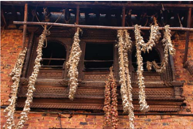
The three bay window, in the second floor has rectangular opening in the centre flanked by openings with cusped arches. The lower plank apron has floral patterns.
