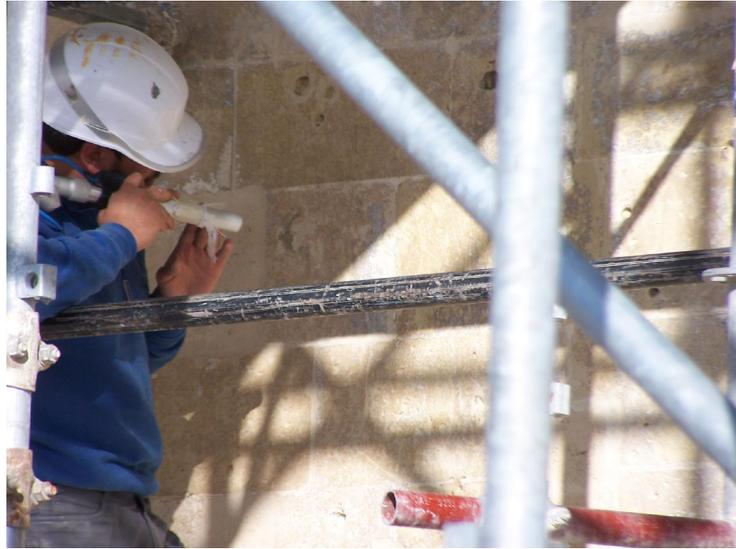
Fig. 6. Laser cleaning of a limited area on the tufa stone surface of the Matera Cathedral.
