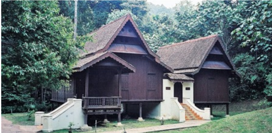
Melaka-style house with a typical Rumah Ibu main house on left and a separate Rumah Dapur kitchen annex behind it at right, with an optional Selang connector space in between
