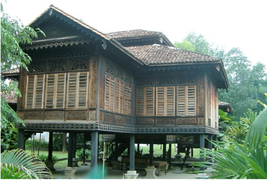
Rumah Penghulu Abu Seman , a traditional Malay house from Kedah state that, as part of the building tradition, was able to be dismantled piece by piece and reassembled on the grounds of Badan Warisan Malaysia, the Malaysian Heritage Foundation in Kuala Lumpur
