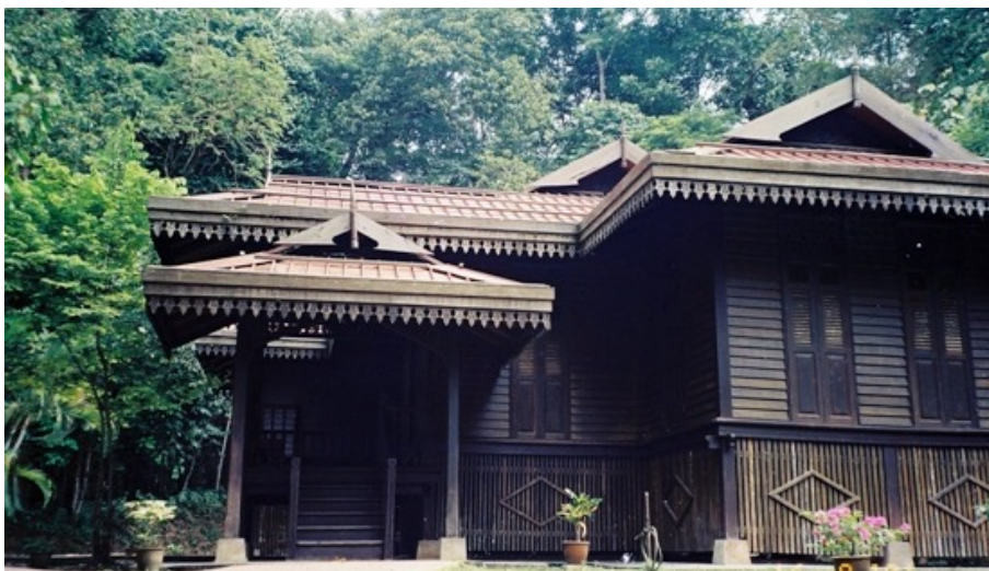
A well-shaded bumbung limas roof type Malay kampung house in the Johor style, designed by Nadge. Note the lines of carved cucur atap or papan lawa roof eaves, and also the buah butung roof pointers that were once reserved for chief's houses.
