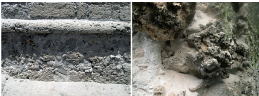
Figure 7. Left: consolidation tests on the Fortim de São José gate. Right: detail of the limestone disintegration in the ruins observed on the Rua Maria Pia.
