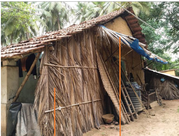
Palm-leaf barrier along walls ('dollois').
