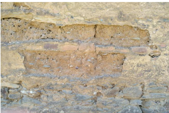
Damages incurred / problems faced: Mason-bee holes.
