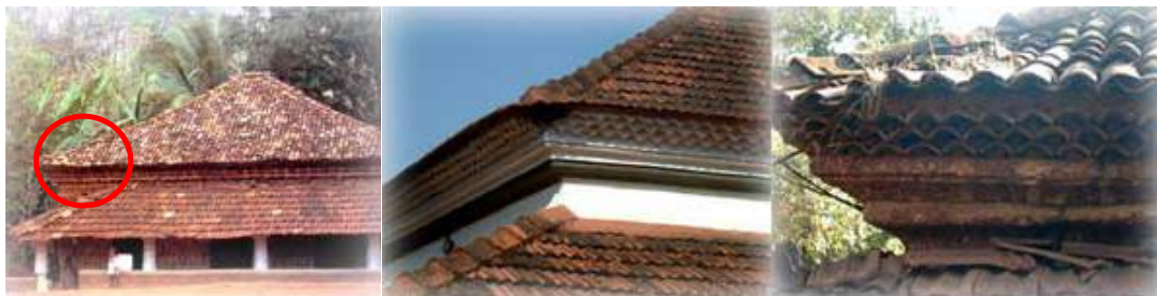
Image 55, Image 56 and Image 57: Corbelling made with 'Country-tiles'.
