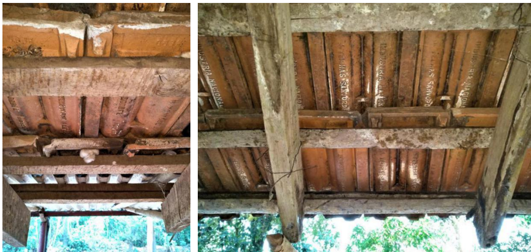
Image 127: Two, instead of one baton was fixed along the ends of the roof's framework (Survey no. 13).
