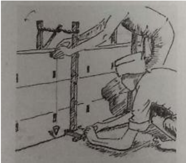
Checking levels with the plumb. [Source: Lobo, Earth in Architecture , p.43]
