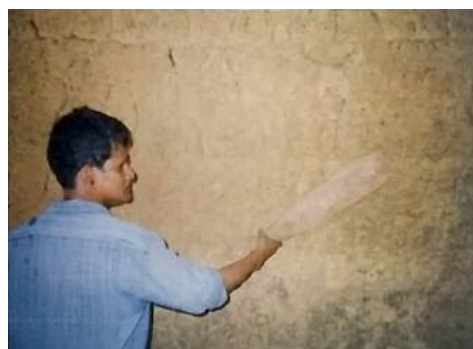
Image 31, Image 32 and Image 33: Cob construction process in Goa.
