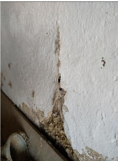
Damages incurred / problems faced: Warping, cracking and fallen plaster.
