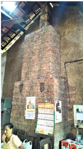
Maintenance and repairs: A laterite block was built to cover the major crack and window opening, and thereby stabilise the wall. The block turned out to be more voluminous than needed.
