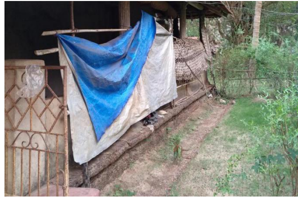
Distinct architectural details: Decorative laterite masonry base-course on front facade. Maintenance and repairs: Tarpaulins, coconut palms and woven coconut-palms protect the veranda from rainwater.
