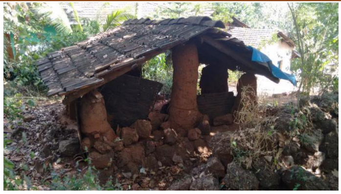
Outhouses, roof supported on earthen pillars.
