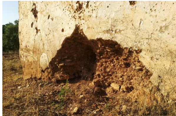
Damages incurred / problems faced: Holes in walls especially where there is lime-based plaster.
