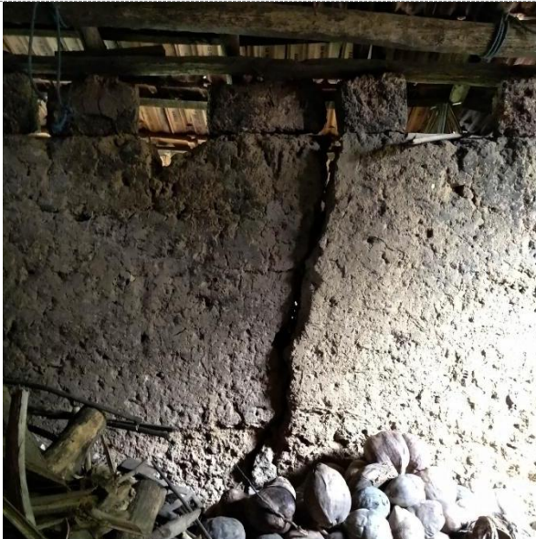
Damages incurred / problems faced: Structural cracks.
