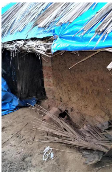
Image 73: Corners; earth with laterite-stones at intervals (Survey no. 11).
