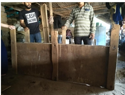
Parts of a recent rammed-earth form-work used in Goa (4 images). [Drawing by Lionel Afonso]
