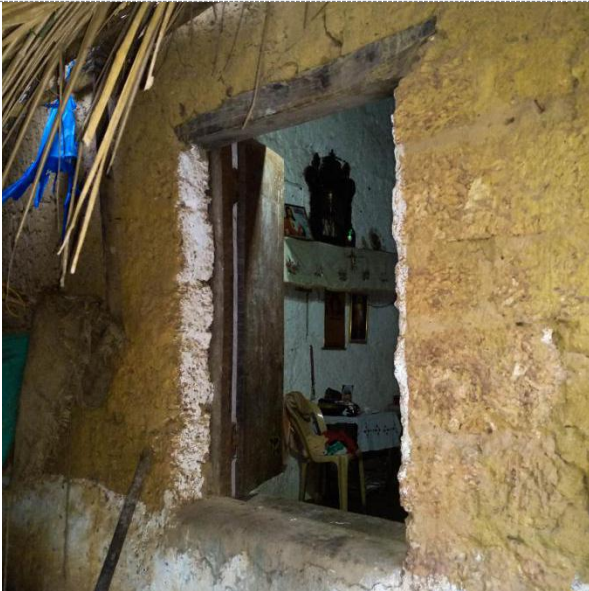
Plasters: Thin coat of lime on earthen walls (interior), including window jambs.
