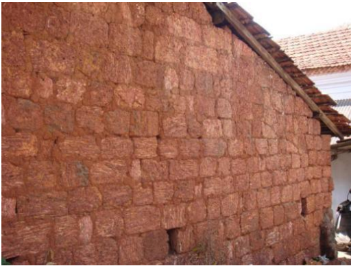
Image 49: Earthen mortars in laterite masonry. [Photo credit: Jose Lourenco]
