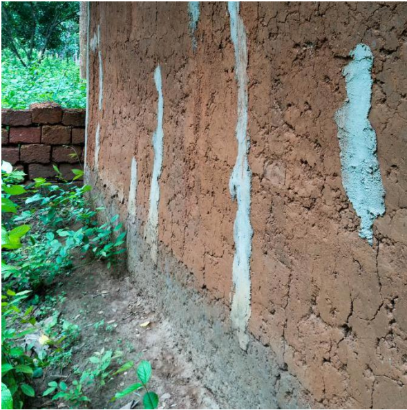
Observations: Base-course is greyish along the one facade. Repairs: Cracks and and other repairs done in cement.
