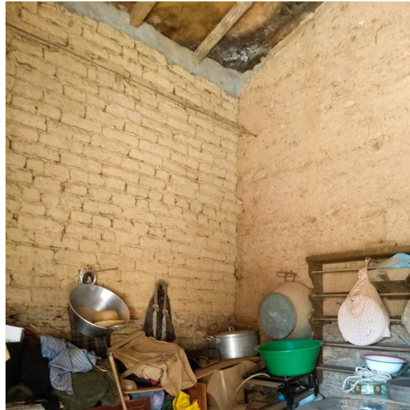
Distinct characteristics: Interior walls are in adobe-bricks.
