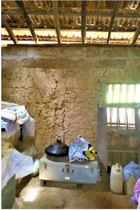
Image 110: Wall heights were extended using laterite-stones (Survey no. 7).
