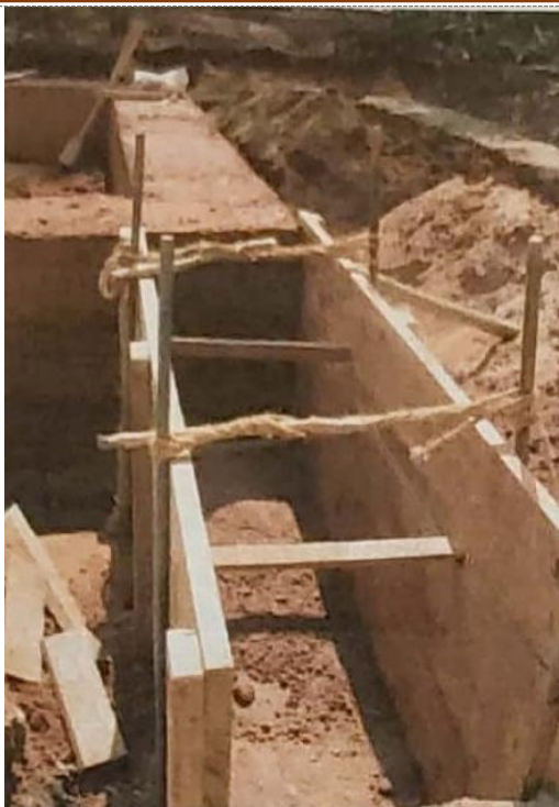
Banche traditionnelle et entretoise ('kani' in Konkani) [Source: Lobo, Earth in Architecture , 2006, p.42]
