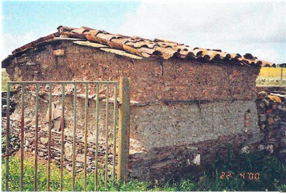
Description of earth used: The second 'lift' is more red and has more schist.
