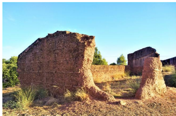
Damages incurred / problems faced: Wall damages got worse with time as the building has not had a roof for many years, some parts of the walls have fallen, vegetation in and around the structure.
