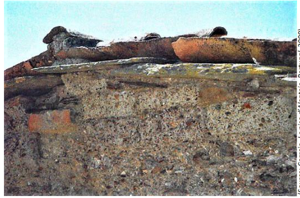
Distinct characteristics: There are adobe-bricks in the gable walls.
