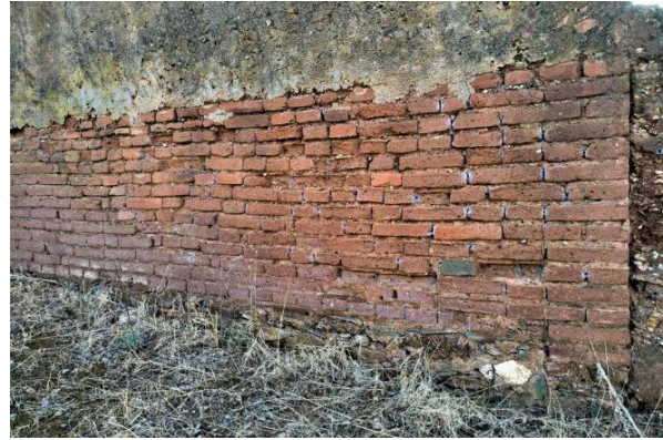
Base-course: In the second division, there is fired-brick masonry on the top of the stone base-course.
