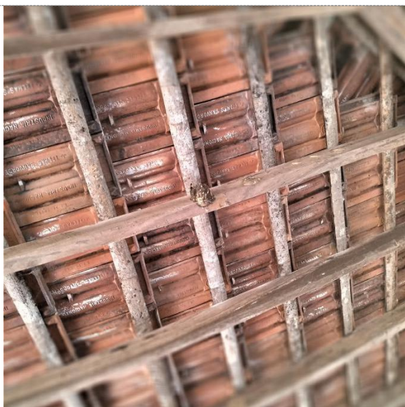
Damages incurred / problems faced: Insects called 'bateen' make nests out of mud on roofs.
