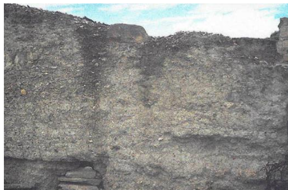
Use of stone in rammed-earth construction.
