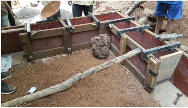
Recent rammed-earth form-works used in Goa.
