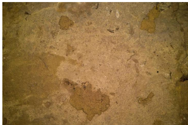
Damages incurred / problems faced: Insects have built earthen-nests on interior walls.
