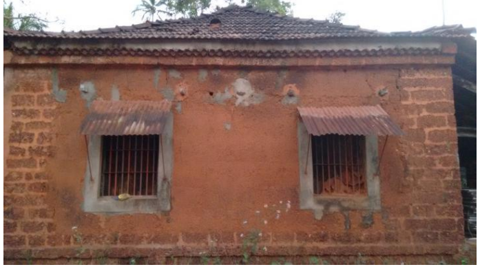
Image 49: Earthen mortars in laterite masonry. [Photo credit: Jose Lourenco]
