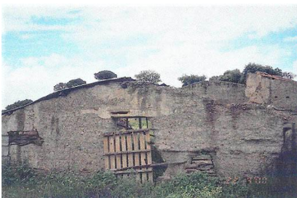
Use of stone in rammed-earth construction.
