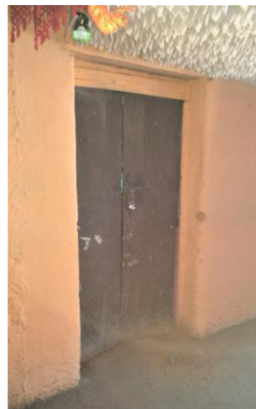
Image 92: Lintels of doors and windows were mostly slanted, and opened up to the interior of the house (Survey no. 3a).
