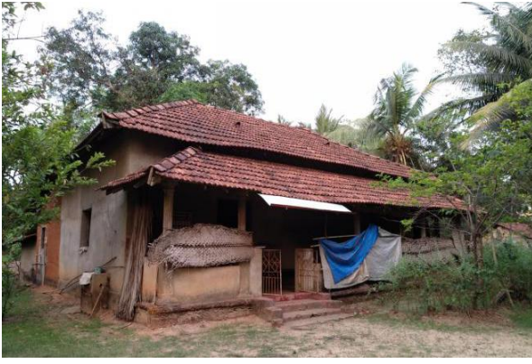
Distinct architectural details: Decorative laterite masonry base-course on front facade. Maintenance and repairs: Tarpaulins, coconut palms and woven coconut-palms protect the veranda from rainwater.
