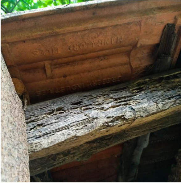
Damages incurred / problems faced: Roof-frame is rotting.
