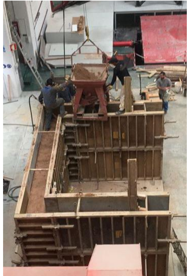
Modern rammed-earth form-work in Portugal.
