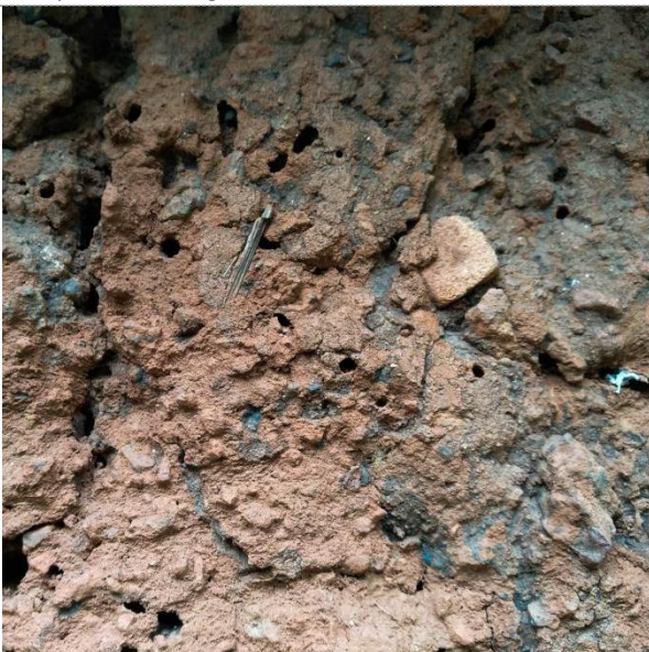
Damages incurred / problems faced: Mason-bee holes
