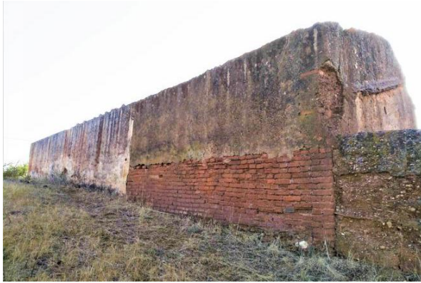
Base-course: In the second division, there is fired-brick masonry on the top of the stone base-course.
