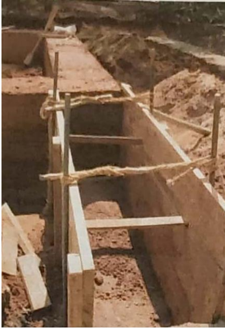
Form-work with ribs and spacers ('kani' in Konkani) [Source: Lobo, Earth in Architecture , 2006, p.42]
