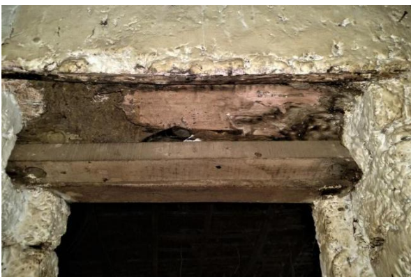
Damages incurred / problems faced: Rotting of lintels.
