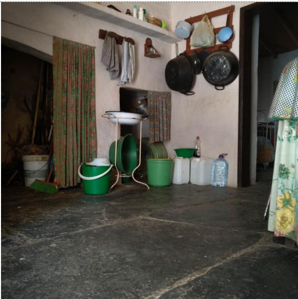
Flooring: Stones were commonly used as floor tiles in the kitchen because they are easy to clean.
