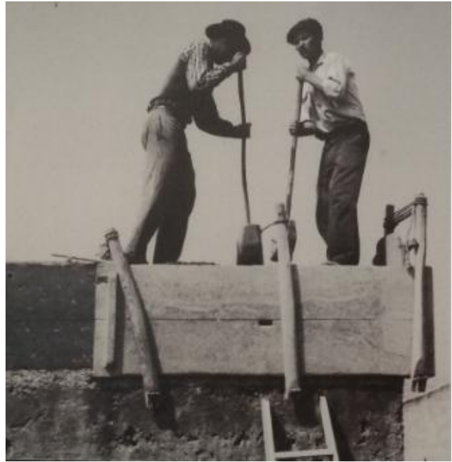
Traditional rammed-earth form-work used Aldeia da Luz in Évora before the 1950's.
