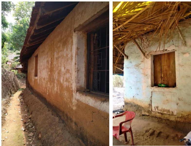
Image 87: A small, earthen gradient covered the foot of external walls (Survey no. 12).
