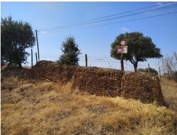
Image 150 and Image 151: Rammed-earth compound wall. Beja, Alentejo, 2018.
