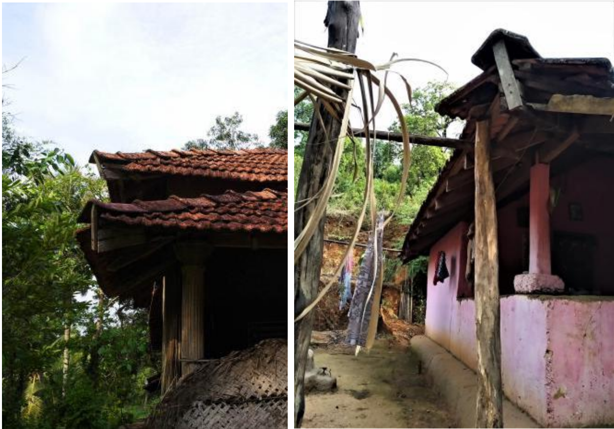
Image 129 and Image 130: Small, wooden batons were fixed on roof corners (Survey nos. 11, 13).
