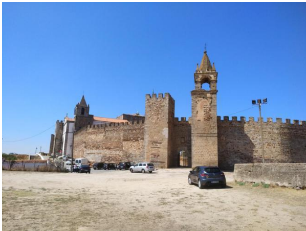
Image 148 and Image 149: Rammed-earth fortification walls. Castelo de Mourão, Évora, Alentejo, 2018.
