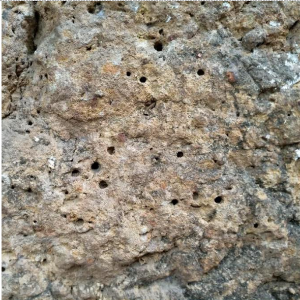
Damages incurred / problems faced: Mason-bee holes.
