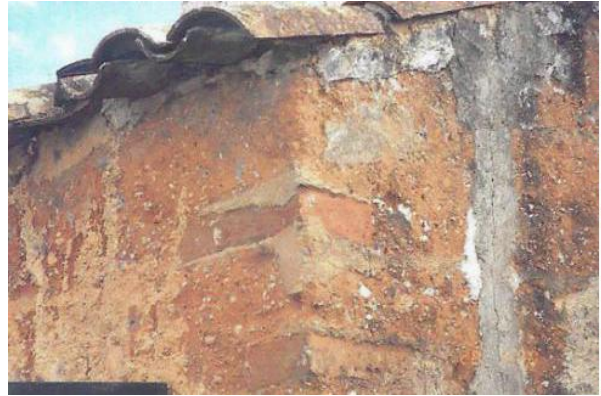
Corners: In rammed-earth and brick.
