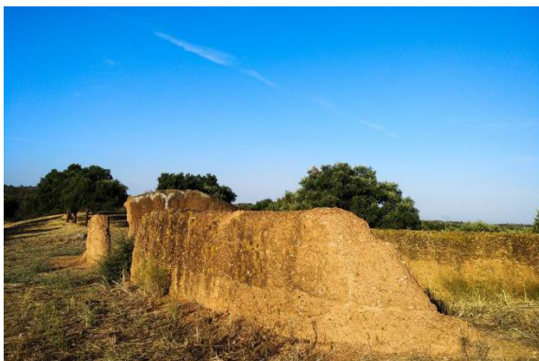
Damages incurred / problems faced: Wall damages got worse with time as the building has not had a roof for many years, some parts of the walls have fallen, vegetation in and around the structure.
