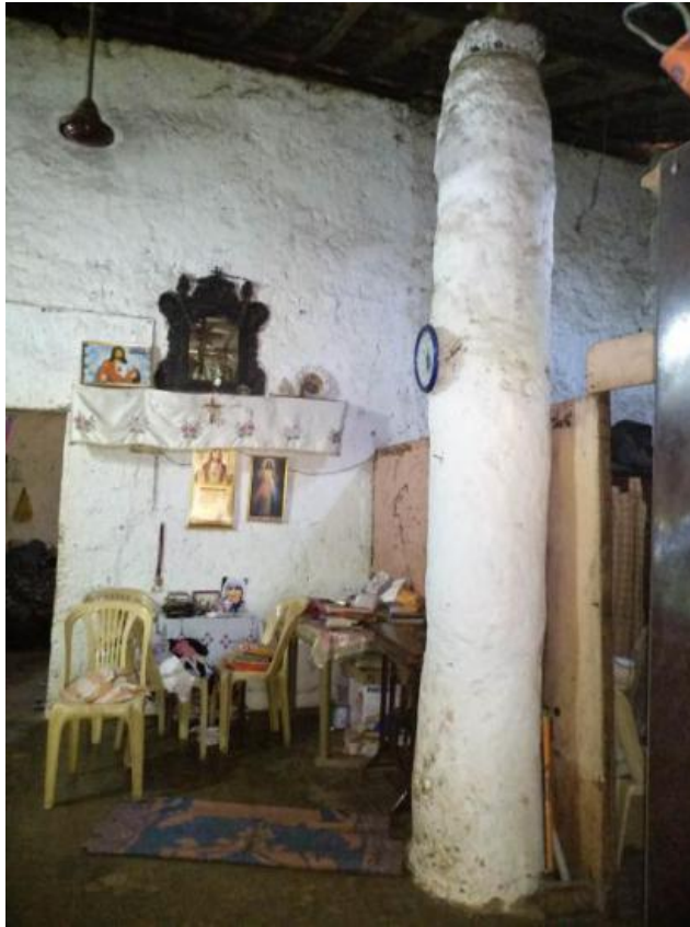
Image 100: Earthen pillar (Survey no. 8).
