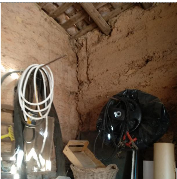
Damages incurred / problems faced: Cracks in corners.
