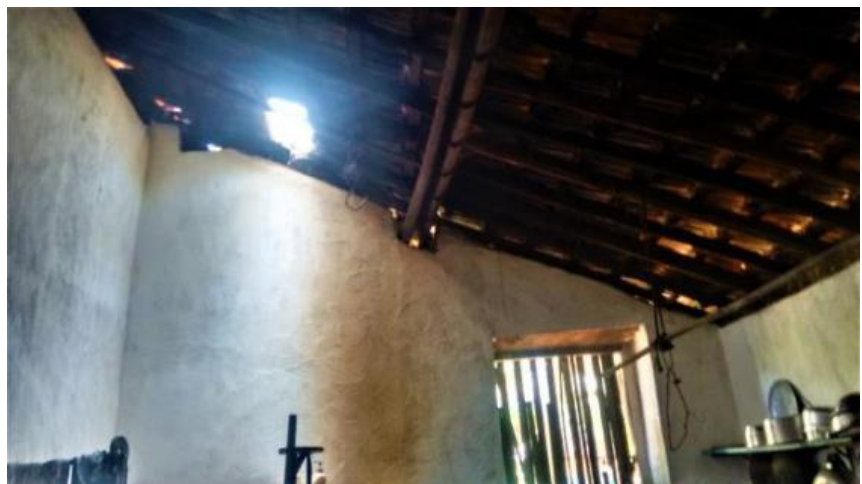
Image 118: Sample of a ventilating roof-tile.
