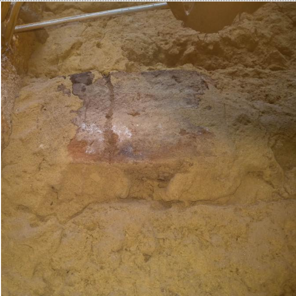
Observations: There is a (piece of) fired brick in the adobe-brick gable.
