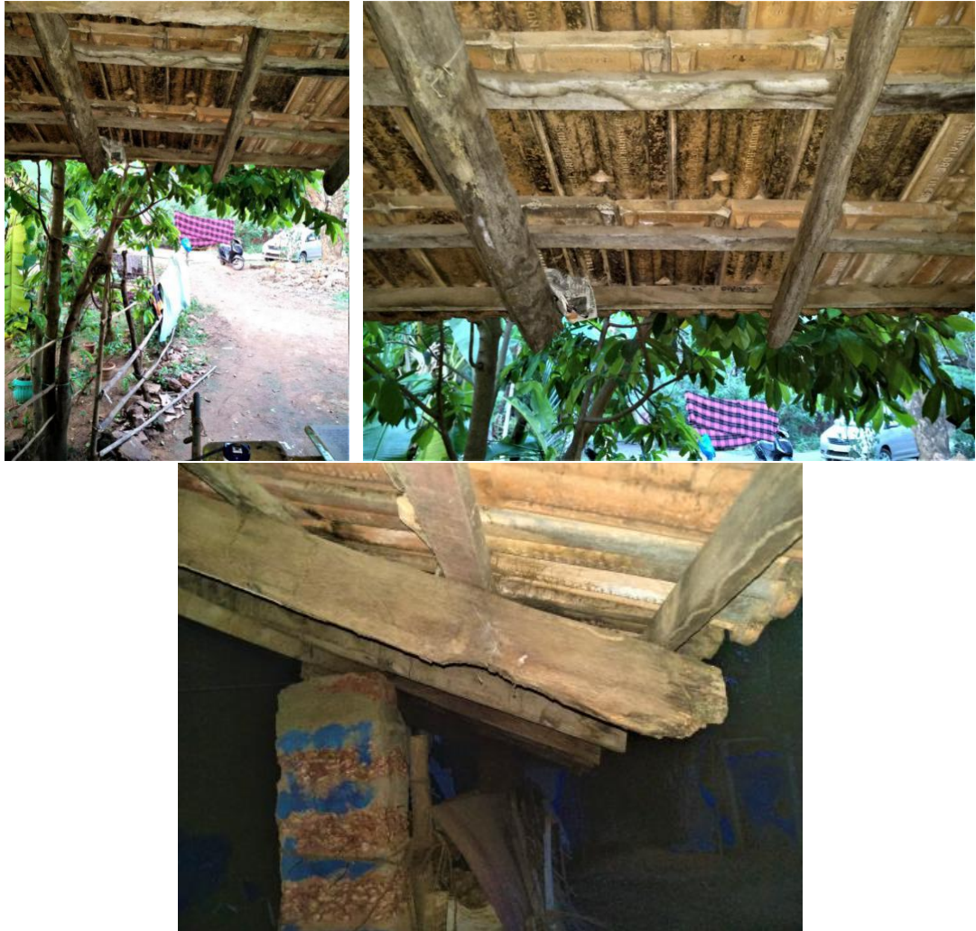
The last baton along the edge of the roof is placed with the smaller side resting on the rafters.
