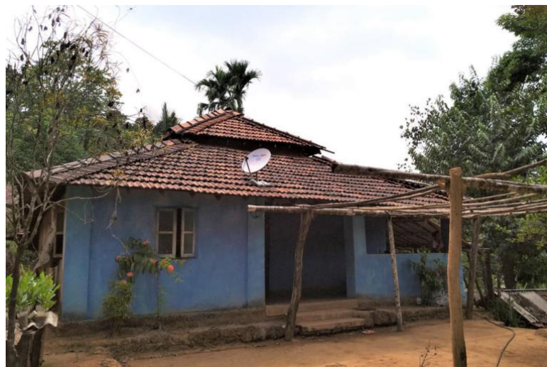
Image 109: The upper part of the roof thrusts upwards, and is separate from the lower part (Survey no. 12).
