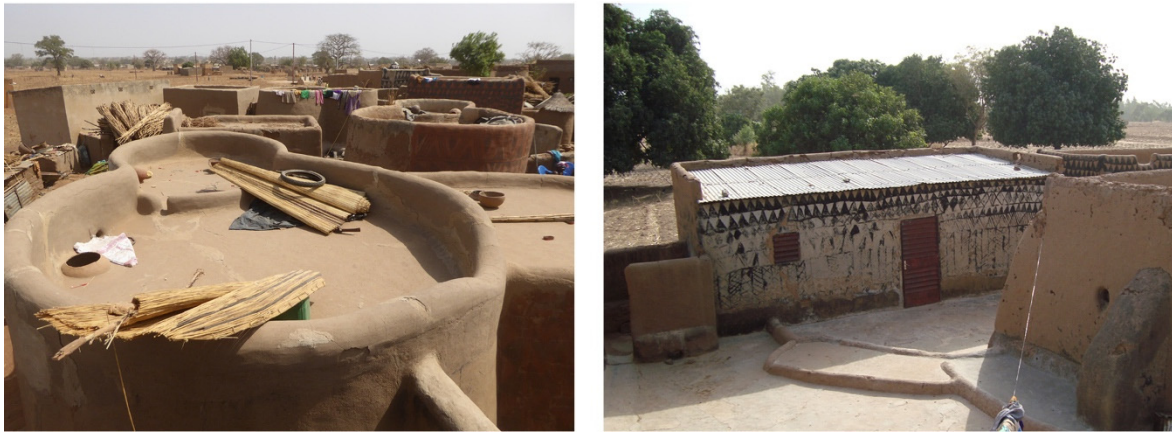
Figure 11. Transformations of the traditional earth roofs in Tiébélé, with the consequent change in the form of the construction.
