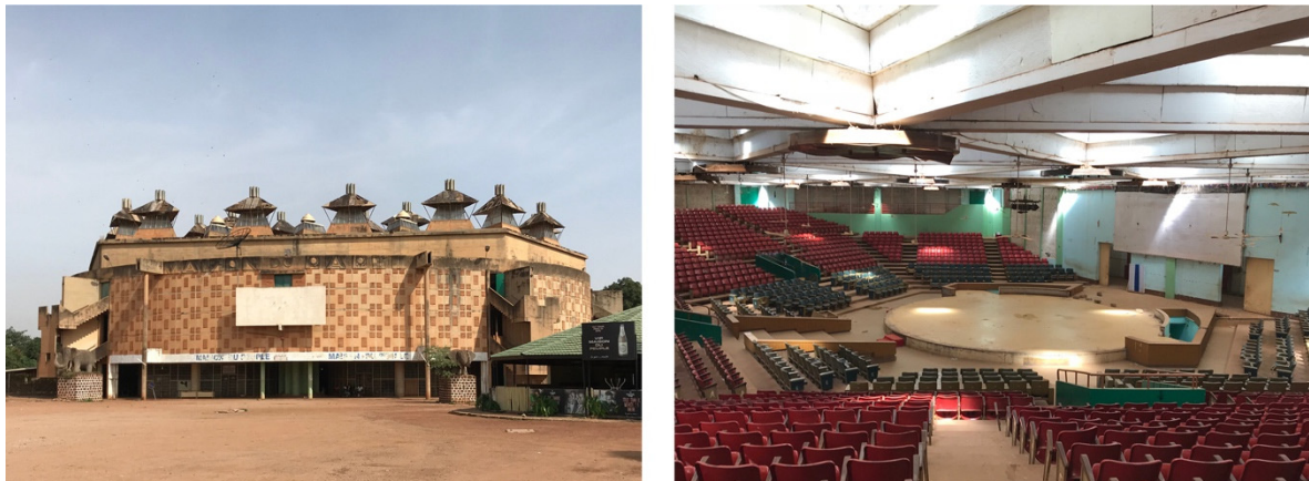
Figure 8. Current condition of the Maison du Peuple in the city of Ouagadougou.
