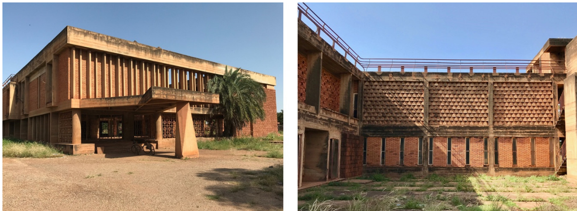
Figure 7. Current condition of the Palais Yameogo in the city of Koudougou.
