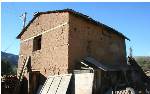
Figure 3. Adobe furnace in Chuchiñf, in which both continuous and corner horizontal wooden reinforcements can be identified.
