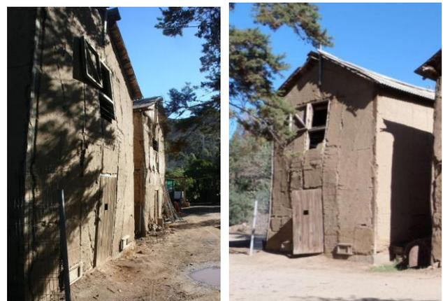
Figure 10. Severe deformation of a tabique wall associated with an inappropriate choice of wooden joints in pillars - Furnace in El Boldo.
