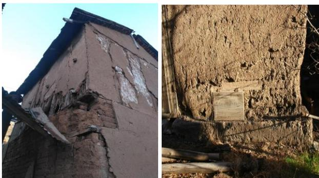
Figure 9a. Erosion in a. upper area of an adobe wall in Chalinga b. lower area of an adobe wall in Chuchiñi.
