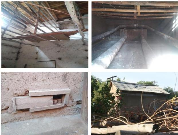
Figure 2. Mechanical features designed to enhance tobacco drying. a. Poplar logs were used to hang tobacco leaves b. Iron tubes conducted hot air through the furnace c. Wooden portholes controlled air intake in the furnaces d. Ridges could be lifted mechanically to allow for better ventilation.
