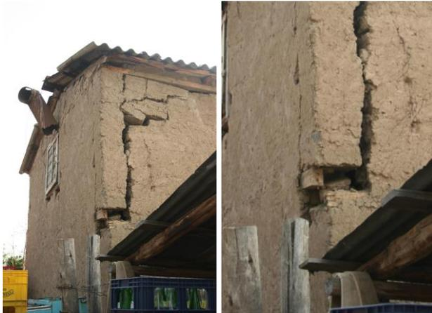
Figure 8. Crack in a furnace in Panguessillo, associated to poor links within its horizontal wooden reinforcement.
