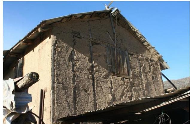
Figure 4. 'Tabique' furnace in El Queñe with one horizontal block between the sawn wooden elements and horizontal wires.
