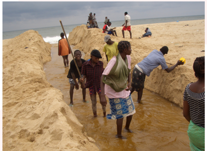
Example of beels created by locals to drain flood water © I. Adelekan
