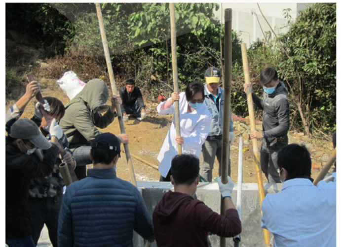
Traditional slaking and preparation of lime with straw fibres © K. Hong Ip
