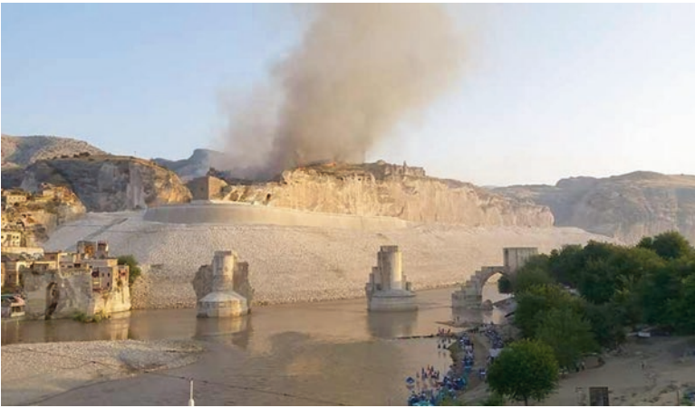
Fig. 24.2 Hasankeyf during dam construction. ( Note. Photograph by B. Gün, 2018)
