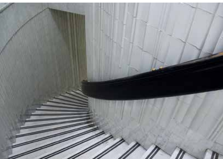
Fig. 11: Stairway leading to the hotel rooms and originally designed ceramic tiling (photo Petr Vorlík)
