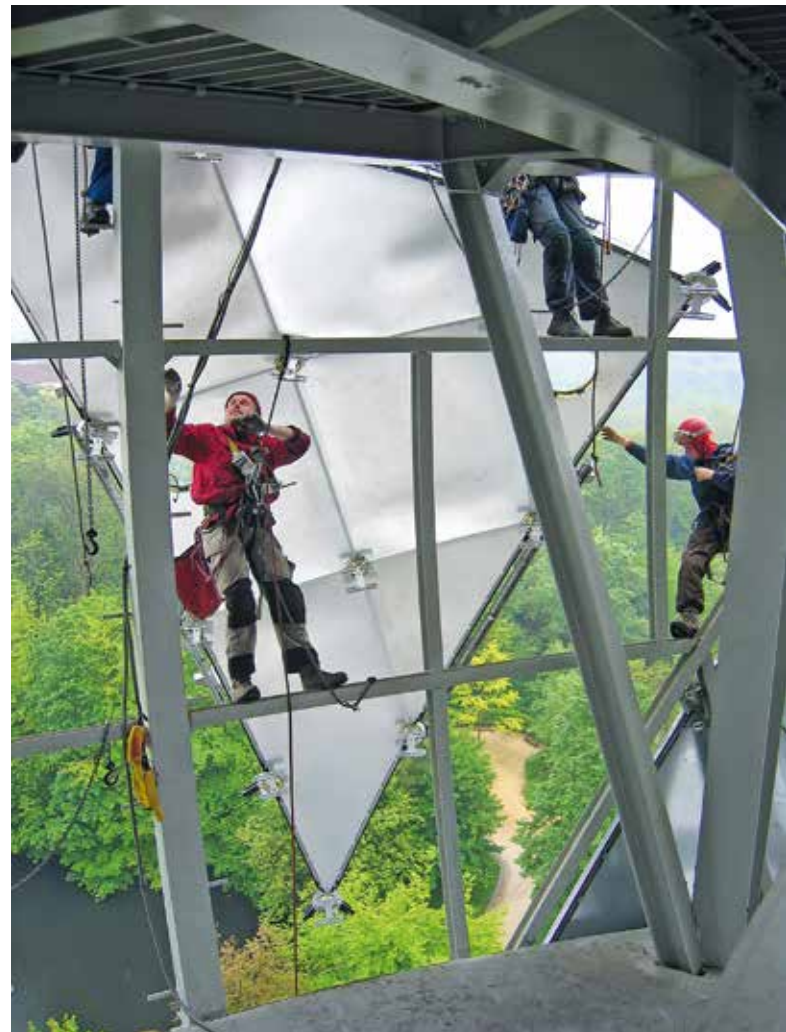
Fig. 5: Installing a panel of pre-assembled triangles (photo Origin 2005)
