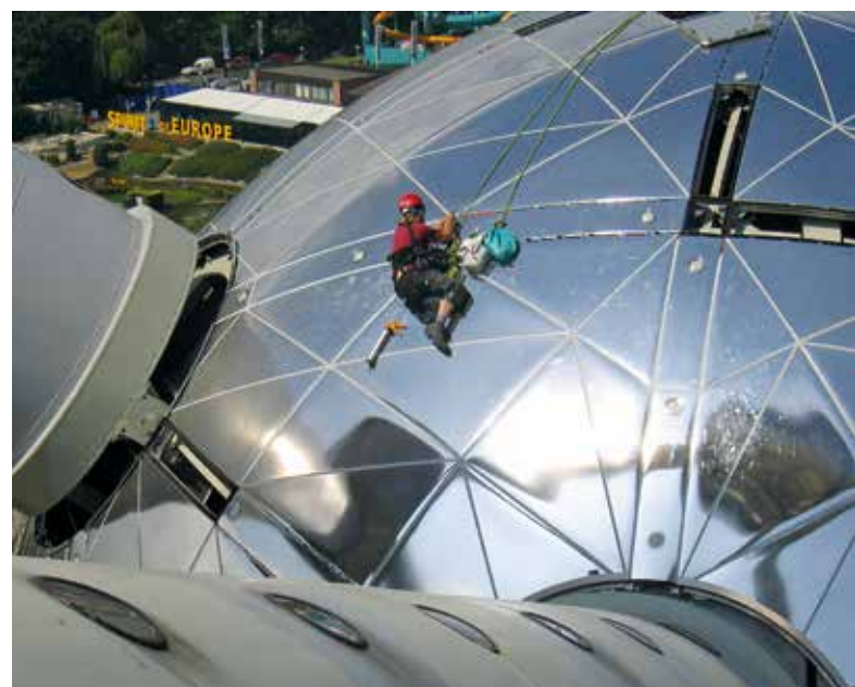
Fig. 6: Installing the meridian plates (photo Origin 2005)
