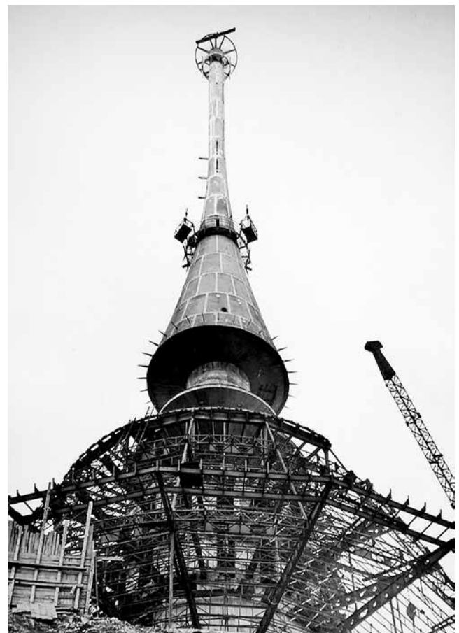
Fig. 1: Photograph of the construction process (© archive of Vítkovice a. s.)
