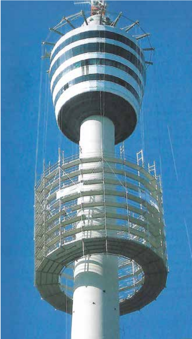
Fig. 9: Elevator on ropes for external repairs
