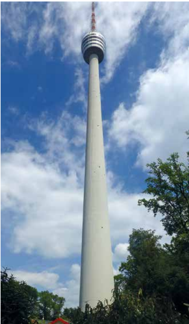
Fig. 1: The first reinforced concrete television tower in Stuttgart, 1953–56
