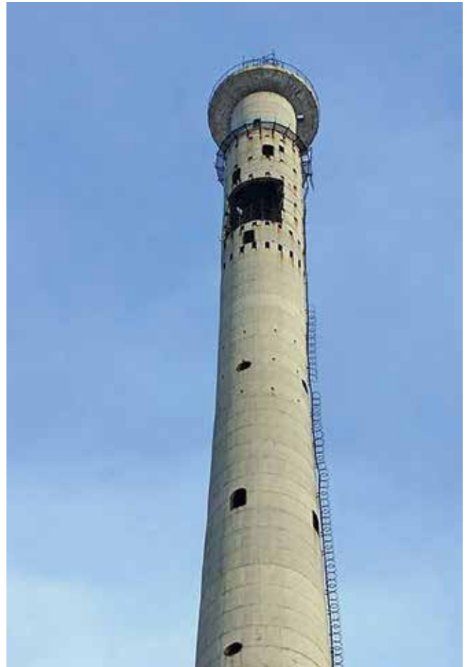
Fig. 3: The TV tower before demolition ( https://neferjournal.livejournal.com/4710982.html )
