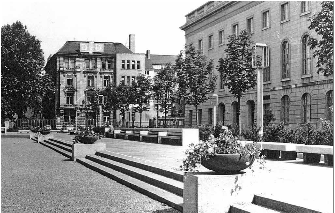
Fig. 4: Humboldt University garden courtyard, view 1962 (Archive of the Humboldt University Berlin/Dokumentation Büro Topos)
