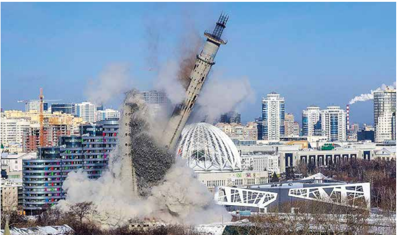
Fig. 4: The demolition ( http://www.brodyaga.com/pages/viewlarge.php?id=51040&cty=Ekaterinburg&place=Russia%20Sverdlovsk&region=Sverdlovsk )
