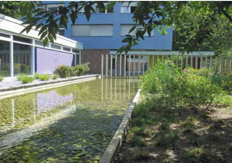
Fig. 12: Akademie der Künste, restored theatre garden with repaired water basin and stele wall (photo Klaus Lingenauber, 2016)
