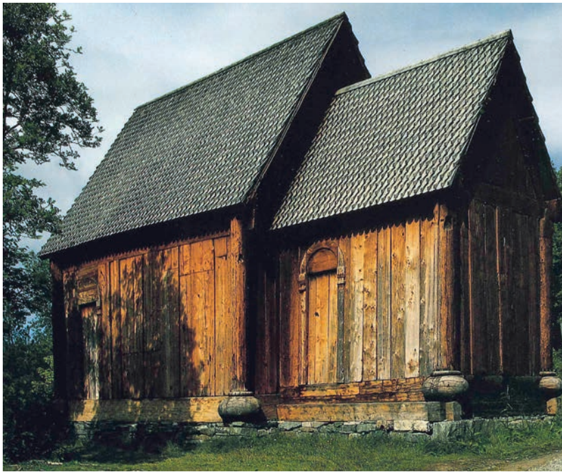
Fig. 8 Stave church without internal vertical central room: Haltdalen, 1150–1200 (drawing by Håkon Christie; from Anker 2005, p. 338)
