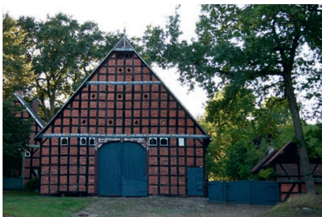
Fig. 1.12 Jabel (Lüchow), hall houses of the predominantly traditional timber-framed construction type (photo by Kerstin Duncker)
