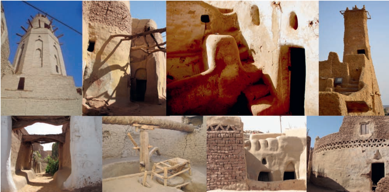
Fig. 2 An overview of earthen building typologies in the Western Desert
