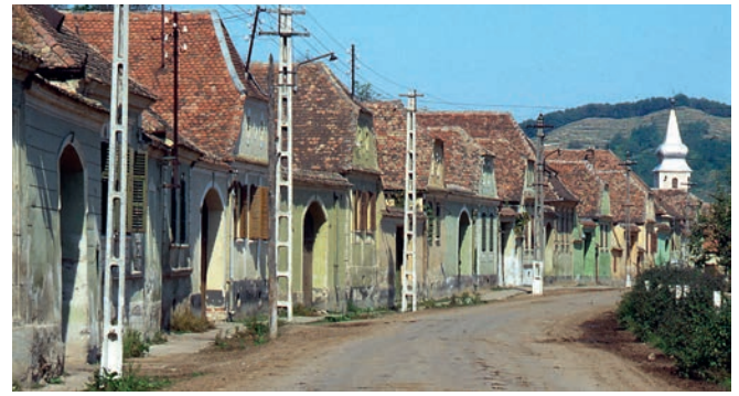
Fig. 16 Richiş (Reichsdorf), main street, row of houses of the Romanian peasants [C. Machat]
