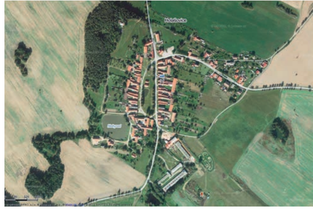
Fig. 4 Holašovice, Czech Republic, World Heritage site, aerial view of the settlement [mapy.cz]
