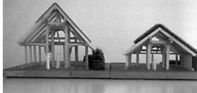
Fig. 14 Borg, high and low models, steep pitch with wood shingles, low pitch with turf
