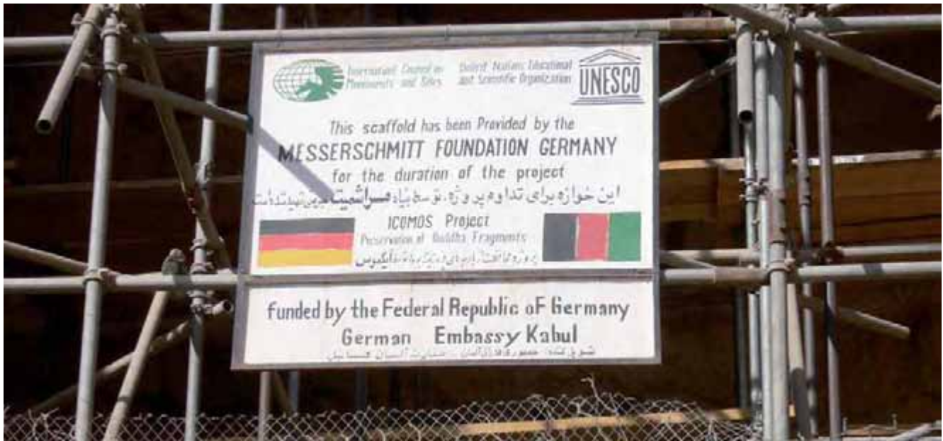
The scaffold provided by the Messerschmitt Foundation
