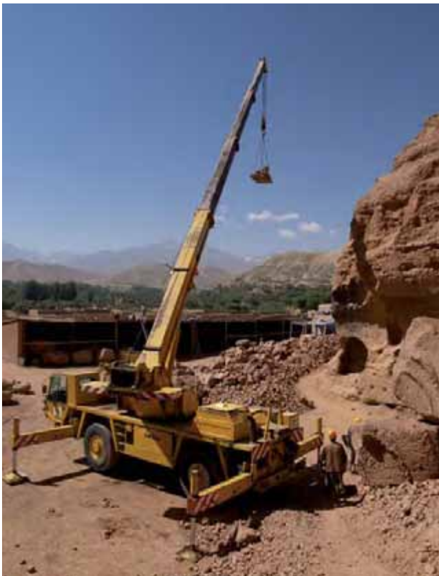
Recovery of rocks by means of a 35 t heavy-duty-crane at the Western Buddha
