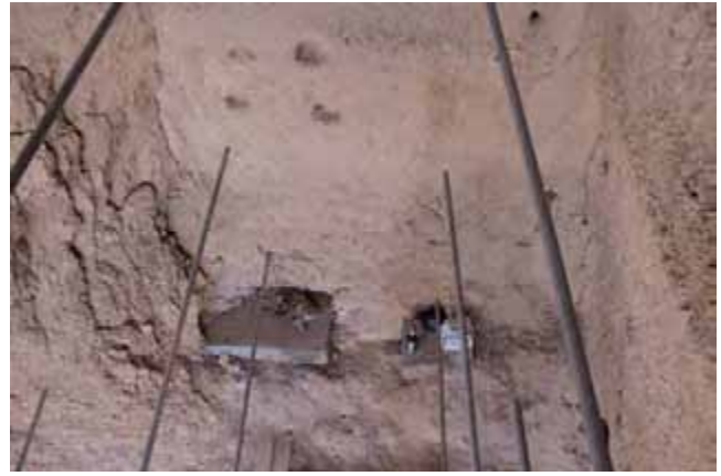
△ Fig. 1b. Left shoulder after removal of the loose rock fragments
