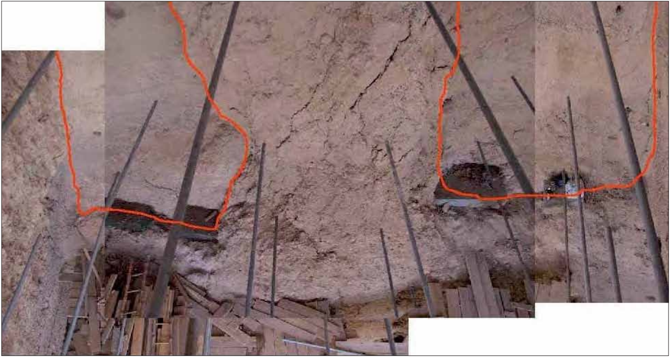
Fig. 9. Trace of an open joint parallel to the back wall (red line)
