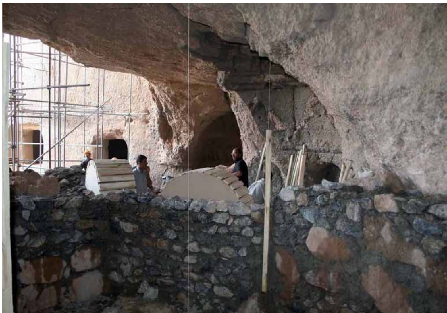
Figs. 8a,b. Reconstruction of the partition wall between caverns no. I and II
