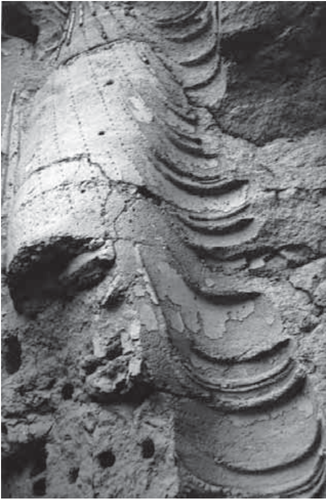
Fig. 6. Western Buddha, detail of right leg in 1965 [ASI] and sketch demonstrating the system with wooden pegs and ropes [Tarzi 1977, vol. 2. p. 117]
