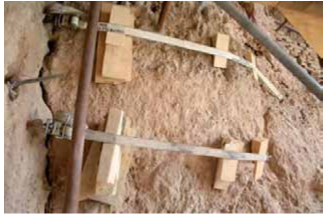
△ Fig. 5b. Provisional stabilisation of the loose wedge
