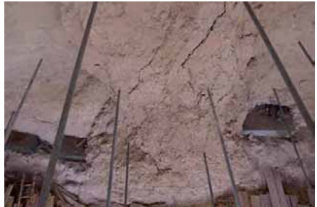
△ Fig. 2b. Head of the Eastern Buddha after removing the loose rock fragments
