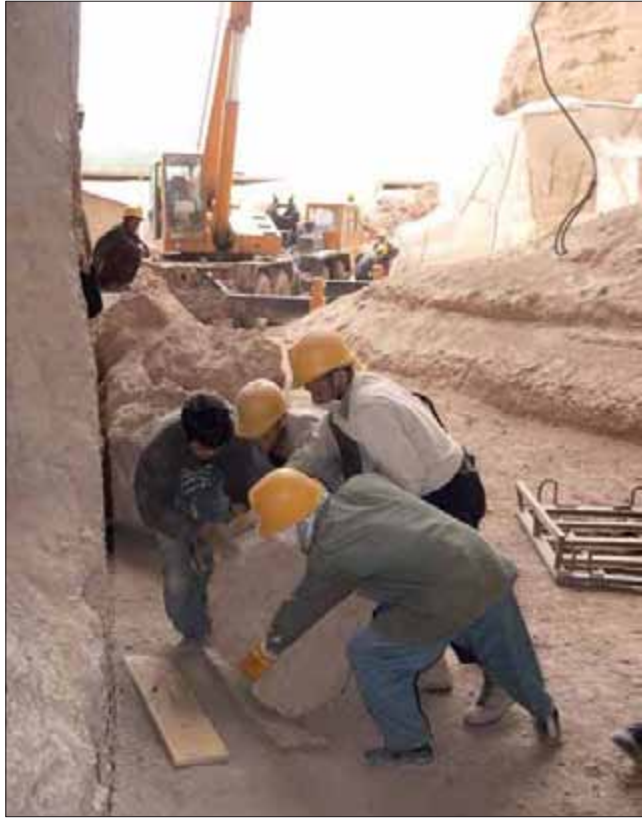
Removal of rock fragments with a heavy-duty crane (left). The steps near the Buddha's shoulder are cleared of rubble so that a temporary base for the upper zone of the scaffold can be added (right).
