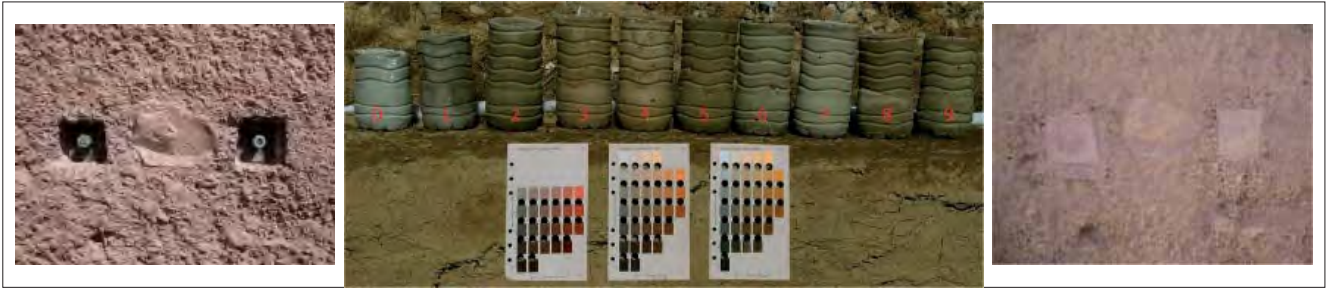
Fig. 22. Covering anchor heads with proper mortar (test site)
