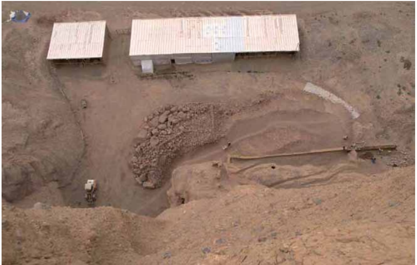
△ Depot for sand, small boulders and rocks without sculpted surface
