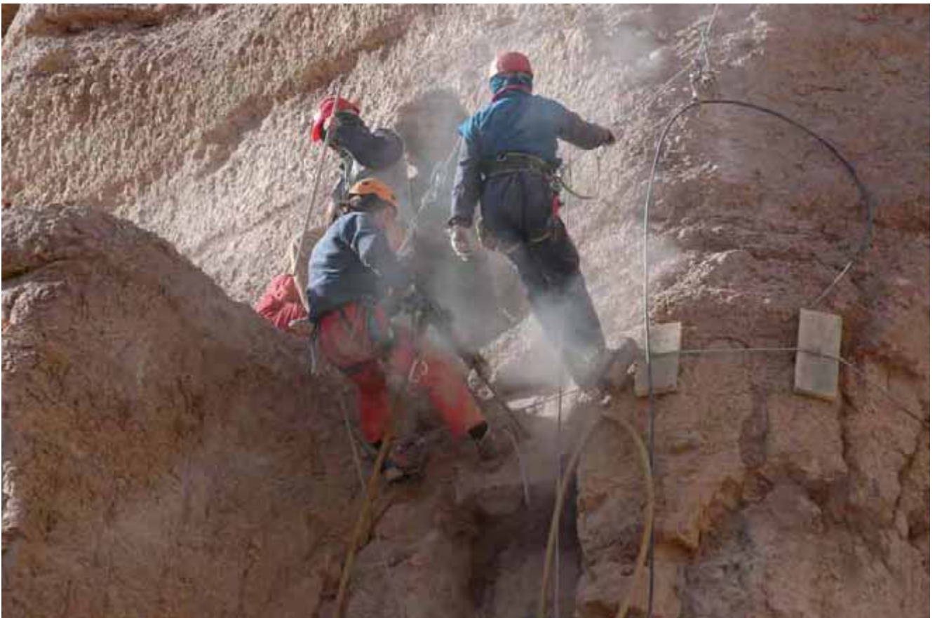
Fig. 36. Drilling the lower part of the niche
