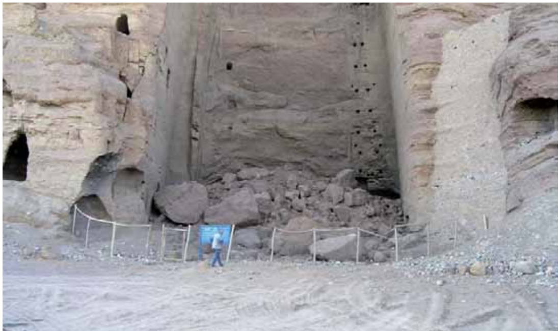
Niche of the Western Buddha with rubble heap before beginning of the salvage work in July 2004
