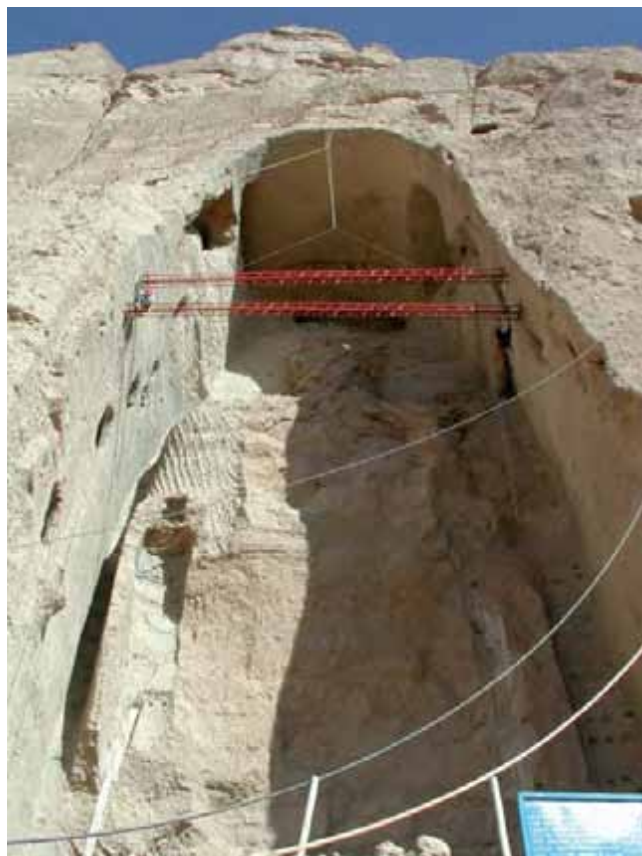
Fig. 13. The temporary beam (left) and steel rope (right) for the temporary support of the upper eastern part of the Eastern Buddha
