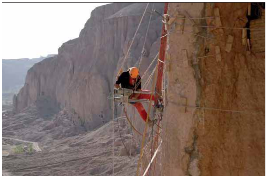
Fig. 29. Drilling for the setting of nails ▷
