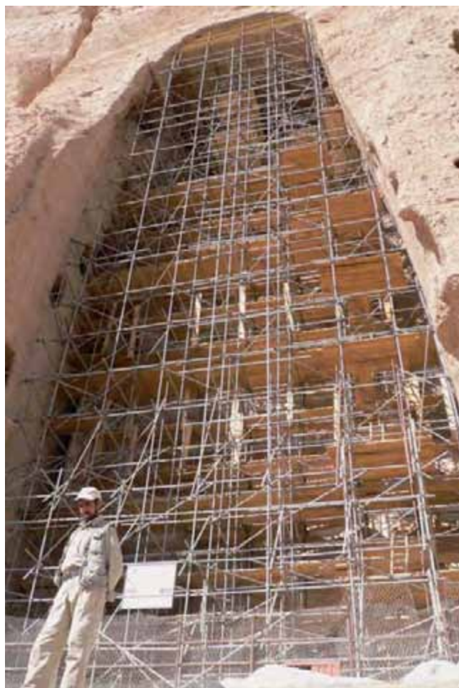
The completely scaffolded Eastern Buddha niche
