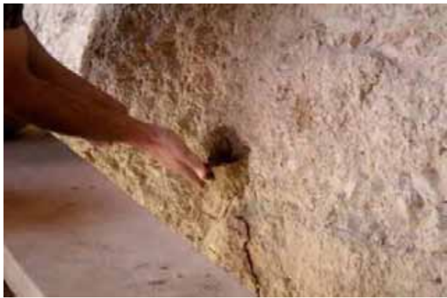
△ Fig. 7a. Preparations for refilling the borehole
