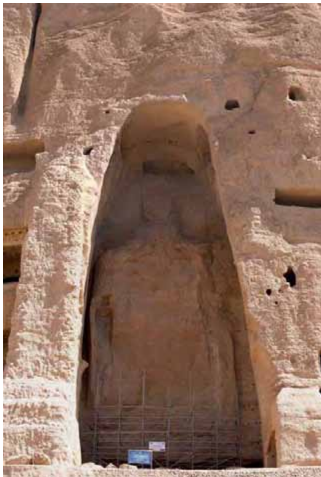
Continuation of erecting a scaffold in the Eastern Buddha niche
