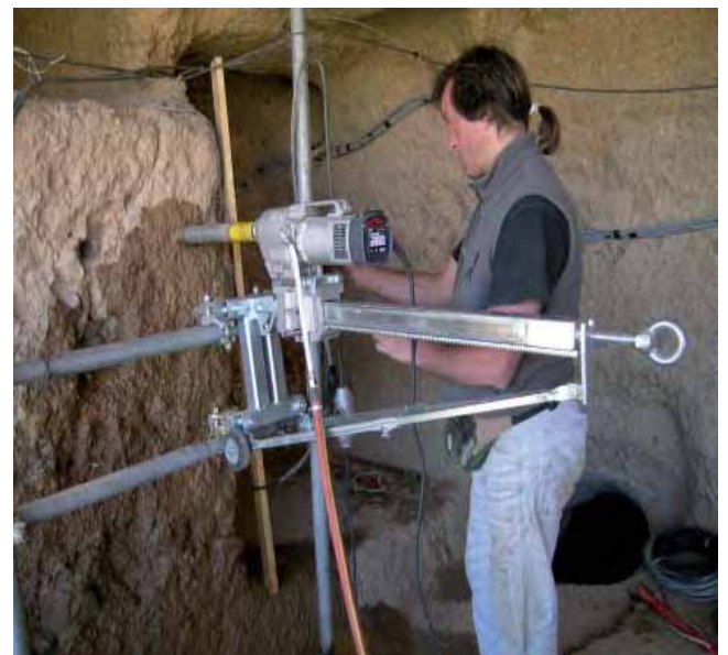
Fig. 21 ▽ Detail of execution of nails from inside the caves by means of a small rotary machine and a diamond head
