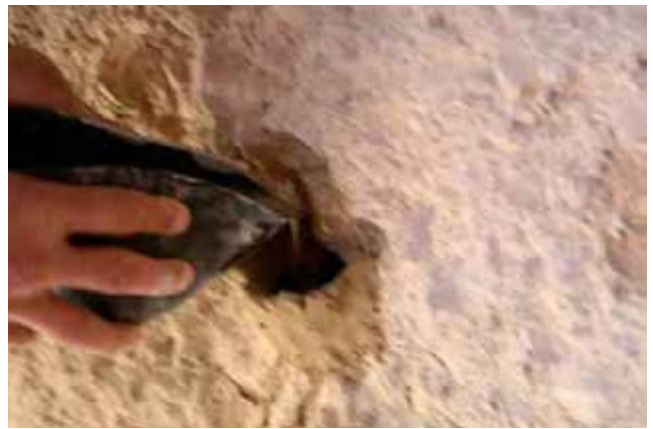
△ Fig. 7b. Filling Ledan into the borehole
