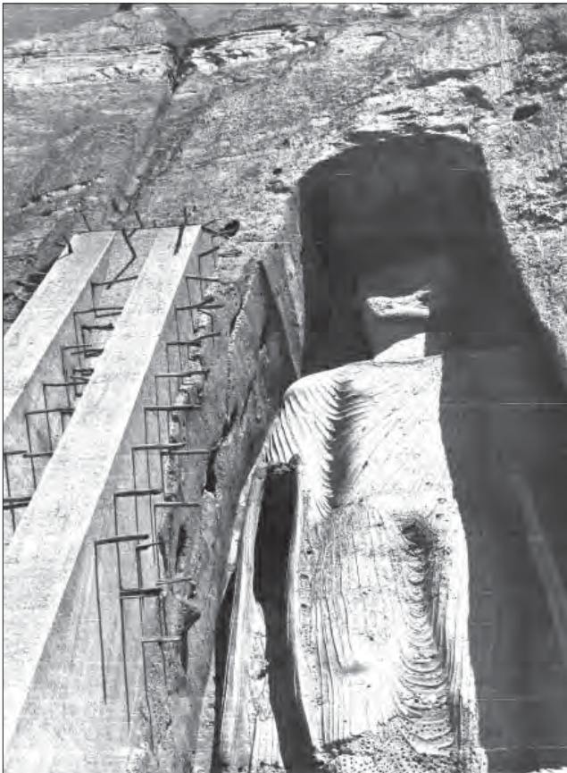
▽ Fig. 20. E. Melzl, Eastern Buddha with brick-faced buttress, 1958
