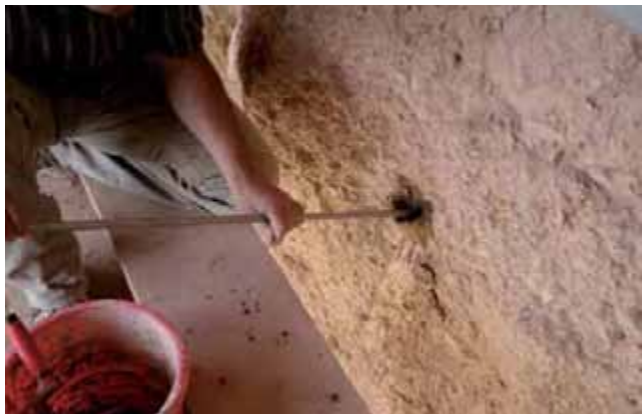
▽ Fig. 8a. Pushing anchor as far as possible into the borehole
