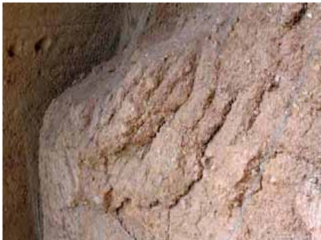
Fig. 19. Right shoulder of the Small Buddha (new discontinuities parallel to the back wall)
