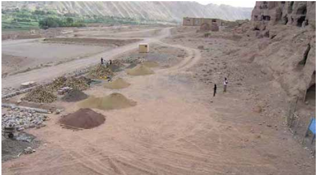
The construction of the shelters begins.
