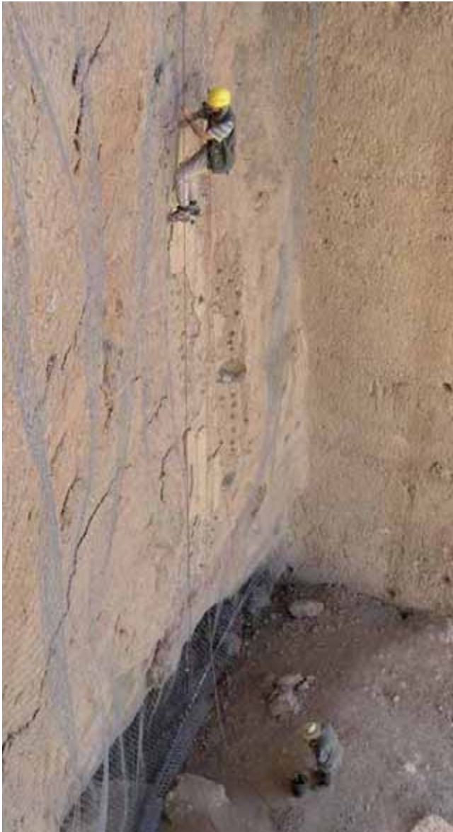
△ △ Emergency measure, alpine style, spot-bonding of clay plaster fragments in situ
