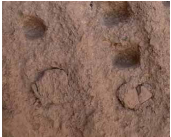
▽▽ Clay lumps pressed into the holes with stones
