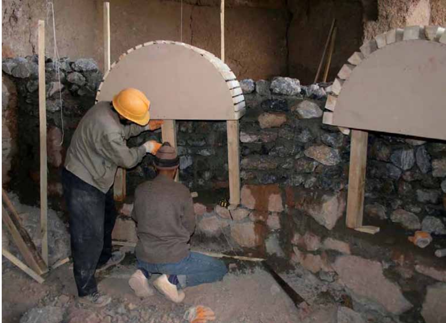
Figs. 8a,b. Reconstruction of the partition wall between caverns no. I and II
