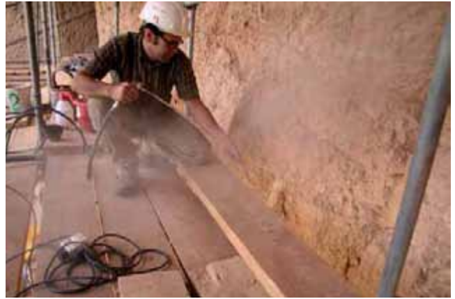
△ Fig. 6b. Removal of dust from the borehole
