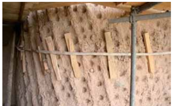
▽ Fig. 4b. Provisional stabilisation of right shoulder
