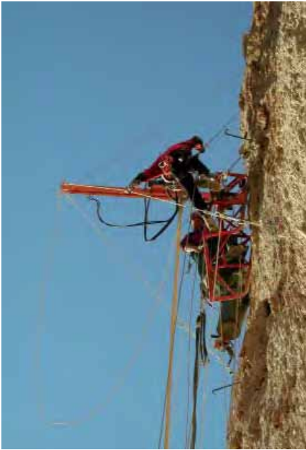
△ Fig. 16 Installation of temporary struts. During the installation the strut is fixed at the top of the cliff, in the safe zone
