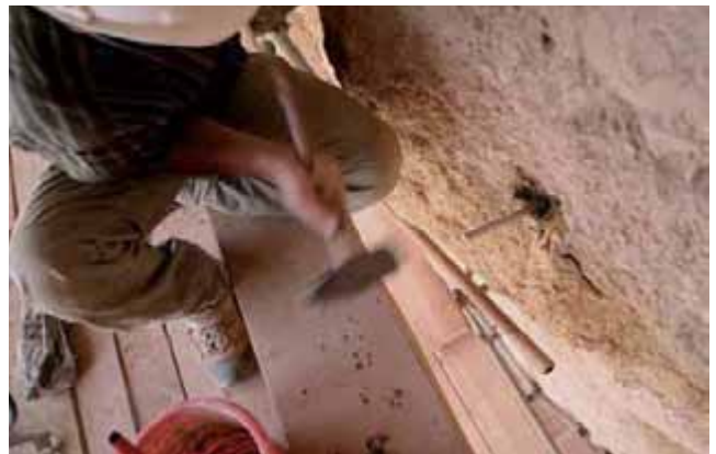
▽ Fig. 8b. Driving anchor into the borehole with a hammer
