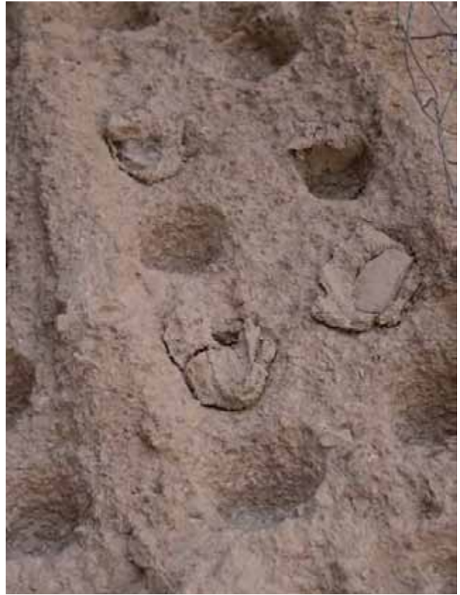
▽▽ Clay lumps pressed into the holes with stones
