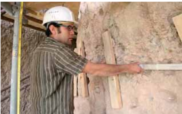
▽ Fig. 4a. Provisional stabilisation of right shoulder
