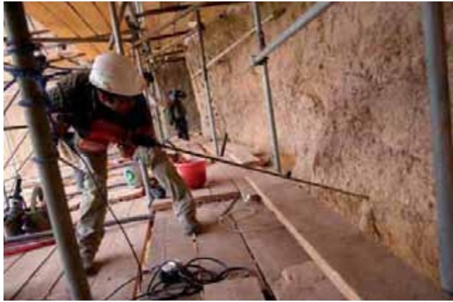
△ Fig. 6a. Drilling of anchor borehole
