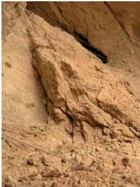
Fig. 18. Remains of the head of the Eastern Buddha (detail with new discontinuities)
