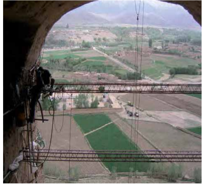
△ Fig. 16 Installation of temporary struts. During the installation the strut is fixed at the top of the cliff, in the safe zone
