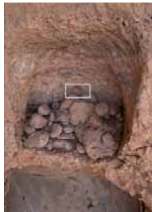
△△ Eastern Buddha, rock cavity with hole in the back wall where the relic was found. The hole is the remains of the beam hole for inserting the Buddha's right arm beam
