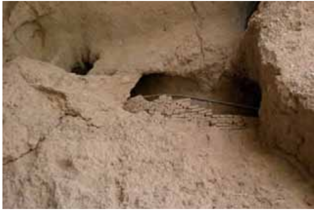
△ Fig. 5a. Loose wedge under the Eastern gallery
