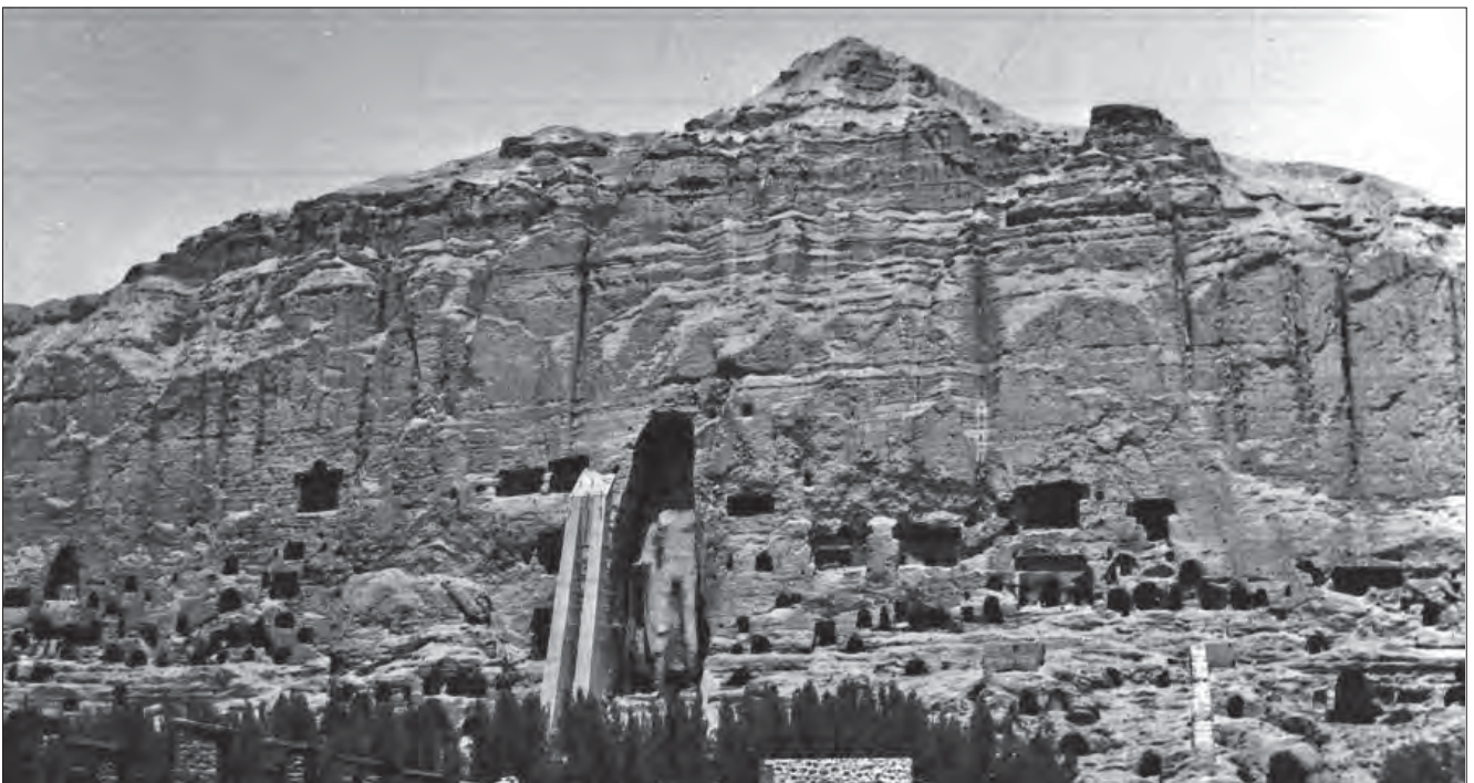
Fig. 24. E. Melzl, view of the Eastern Buddha with new buttress, 1958
