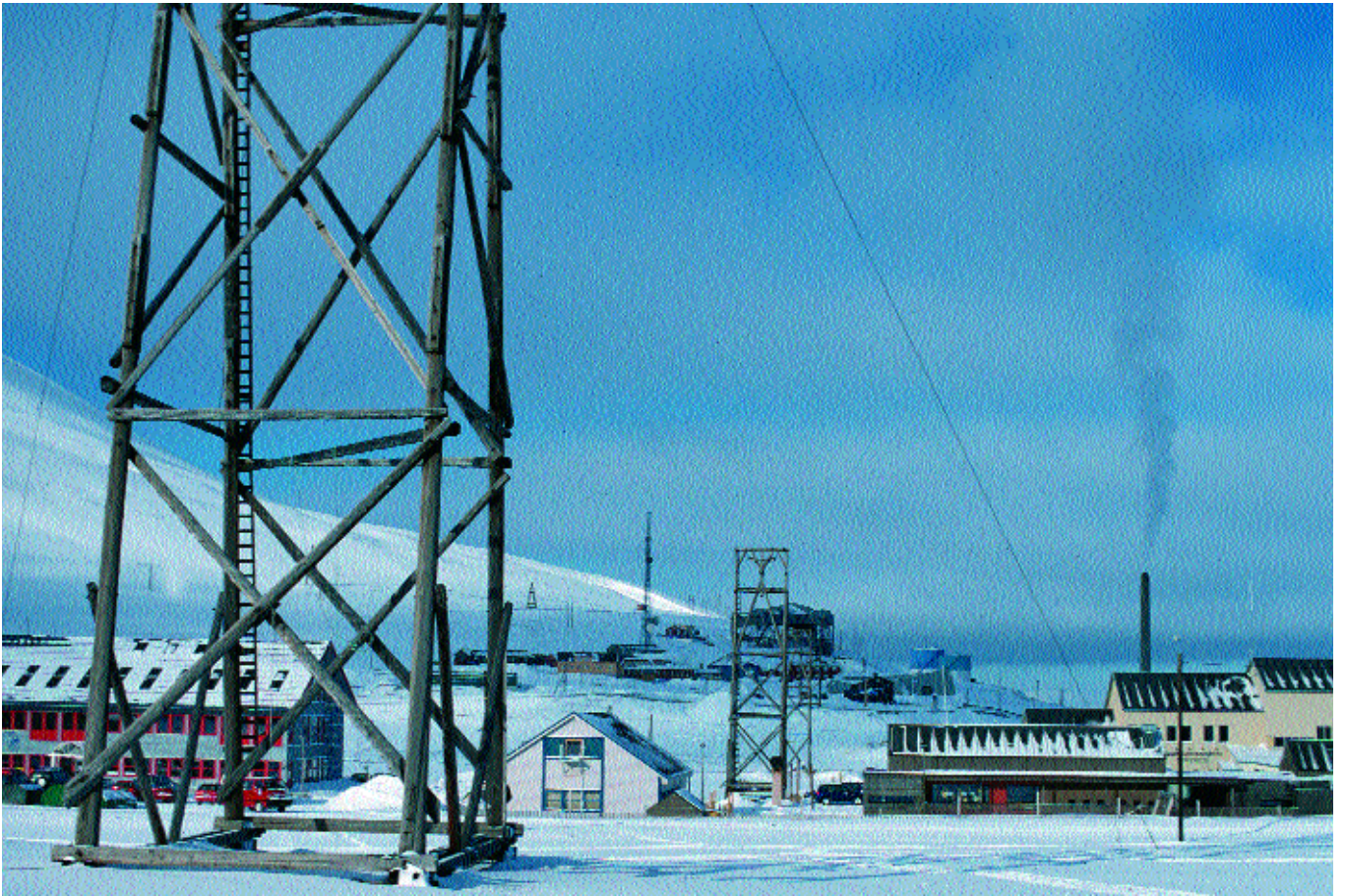
The aerial transport system for coal that goes through the middle of the present settlement of Longyearbyen, Svalbard. Although the cables were taken down when the transport system went out of use in 1986, it is still easy to see how the system worked. The entire system was protected by law in 2003. (Susan Barr)
