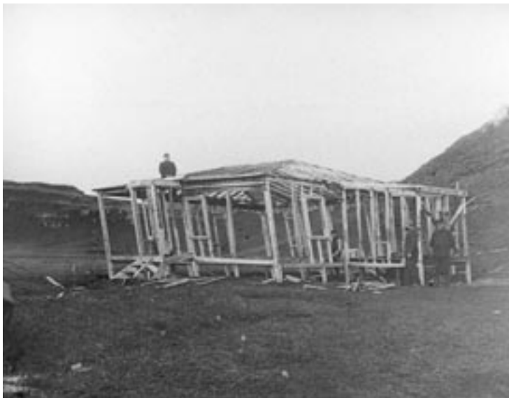
Fig. 1 Remaining upright timbers of the British Volage sta- tion at Observatory Bay in Royal Sound, Kerguelen in 1901, before they were used for the German accom- modation hut. (Geographical Institute, Technical University, Munich)
