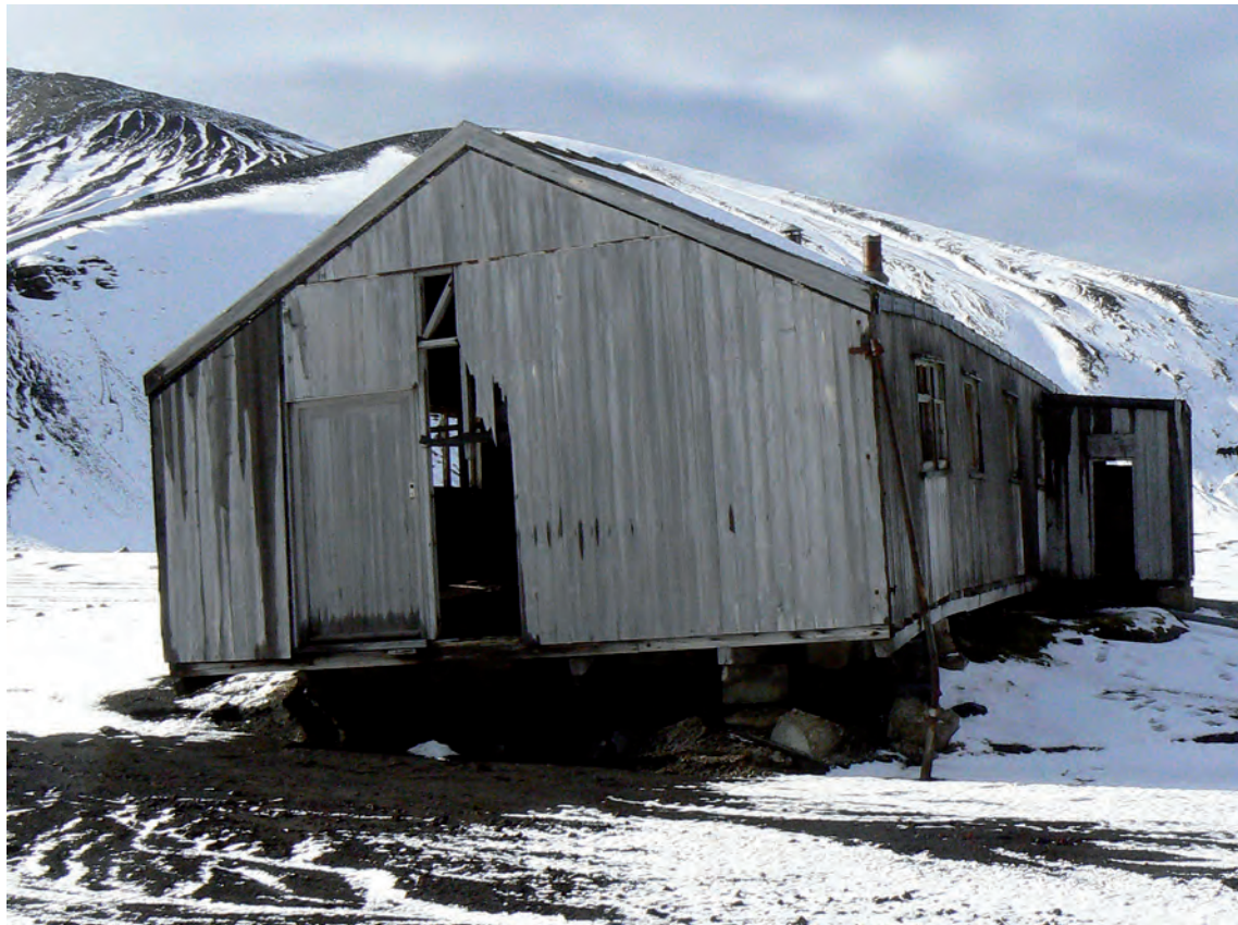
Figure 9. The Hunting Lodge has significantly less deterioration than other structures at the site partly due to a high foundation keeping the wood well above the soil. However the left corner shows erosion of the foundation that is in danger of collapse. Photo: Benjamin Held
