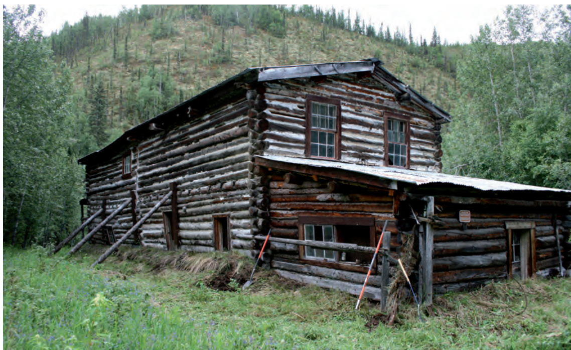
Figure 4. The Steele Creek roadhouse in 2009, prior to beginning of the work of replacing the rotten lower wall logs. Western shed in foreground. Note the thick earth berms piled up along the north, long axis wall, and the external braces placed against the north wall in 2003. View from the northwest. (Photo: Robin Mills, BLM Alaska)
