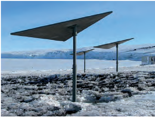
Fig. 3. With snow and ice build-up threatening Captain Scott's base at Cape Evans, 5 Vortex generators have been installed behind the base. The generators disturb the wind flow which creates turbulence and the effect is intended to minimise the snow accumulation against the southern and eastern aspects. Although we are in the early stages of the snow and ice mitigation measures, we are already seeing positive results. (Photo: AHT)
