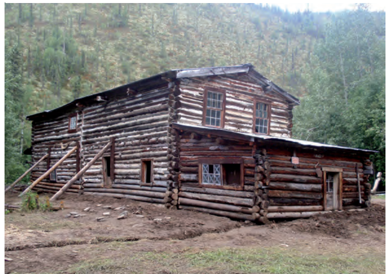
Figure 11. The roadhouse with replacement lower wall logs atop (hidden) pits full of river cobbles. Note the external braces installed in 2003 on the north side of the building have been re-set and left in place, as a backup against unforeseen shifting of the building. View from the northwest. (Photo: Robin Mills, BLM Alaska)
