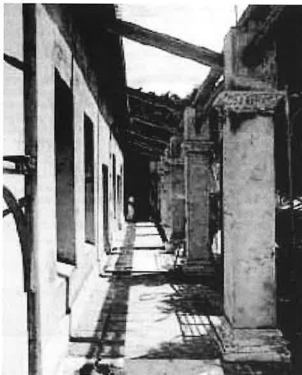
Fig. 4. Exhibition hall under preservation. Photo taken by Kuo An Tsung Architecture Association preservation
