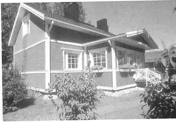
Nowadays it is typical to change the outward appearance of these houses by adding typical features of 1800s architecture, like moldings and small paned windows (Photo: Anu Soikkeli)
