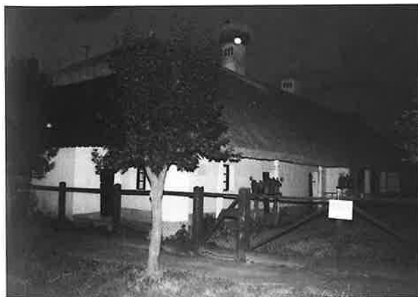
Balatonszentgyörgy, street façade entryway (Photo by Géza Kulcsár)
