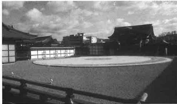
Underground Auditorium at Higashi-Hogan, Kyoto, Japan Auditorium souterrain à Higashi-Hogan, Kyoto, Japon
