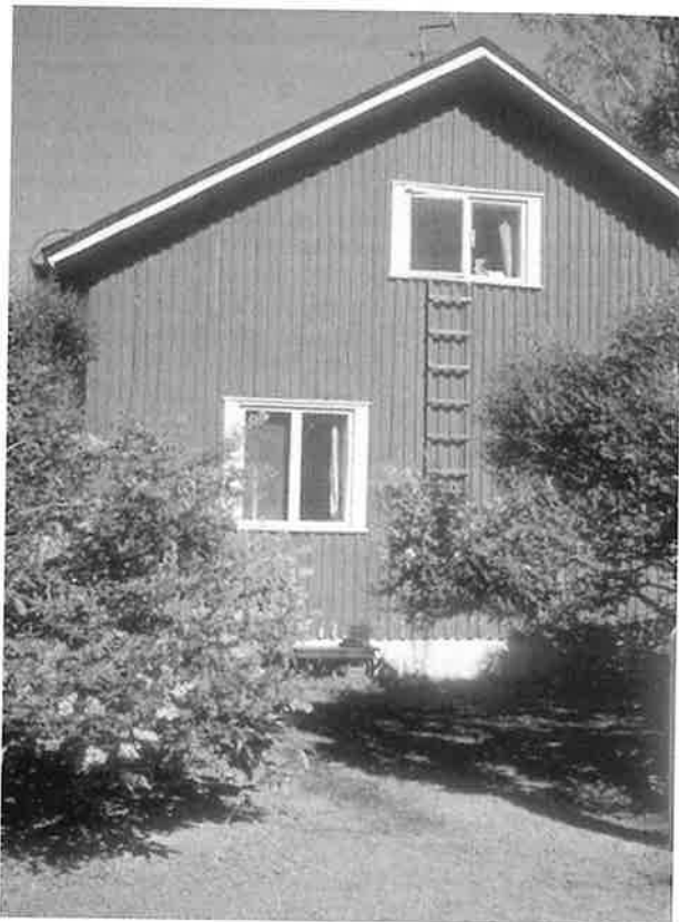
Originally the simple houses were covered with horizontal or vertical boarding – both types of boarding were never used together in the same building (Photo: Anu Soikkeli)
