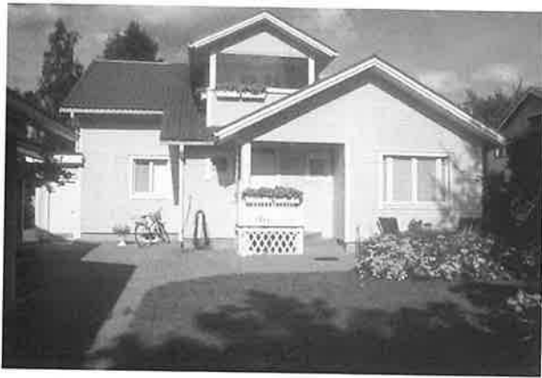
Some of the buildings has been refurbished and modernized completely from the outside (Photos: Anu Soikkeli)
