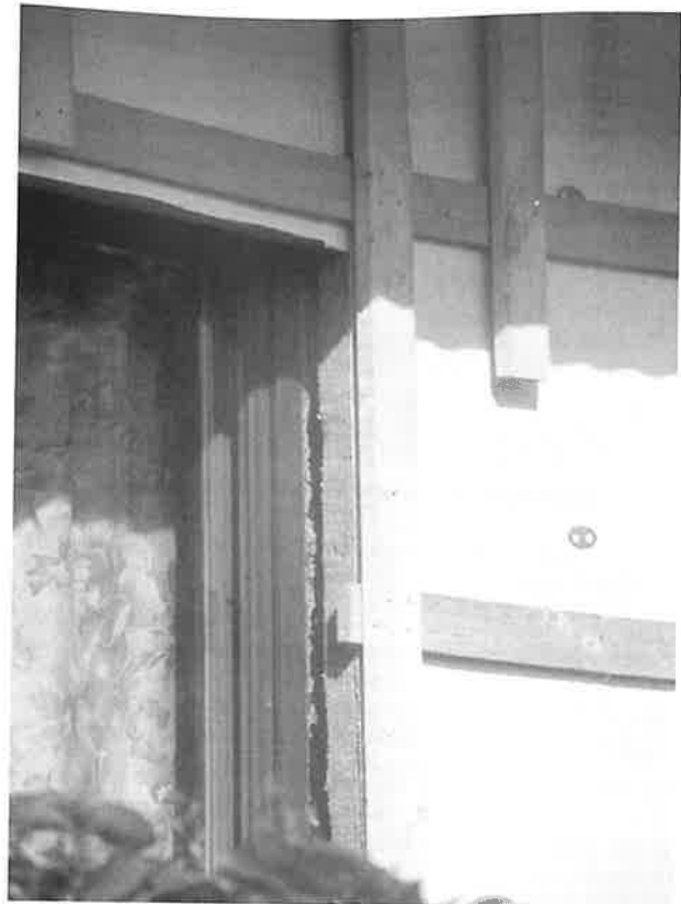
It is common to add insulation to old buildings in Finland - windows are often left deep in the facade (Photo: Anu Soikkeli)
