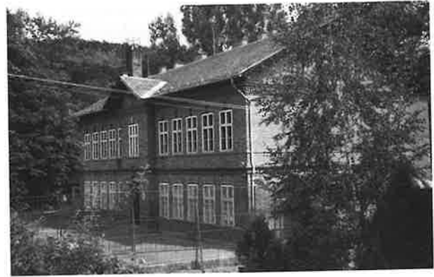
School building in the miners' settlement of Pereces. École de l'exploitation minière de Pereces
