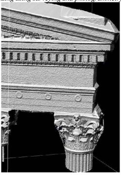
Figure 3 – Complex surface of historic building using laser scanning.
