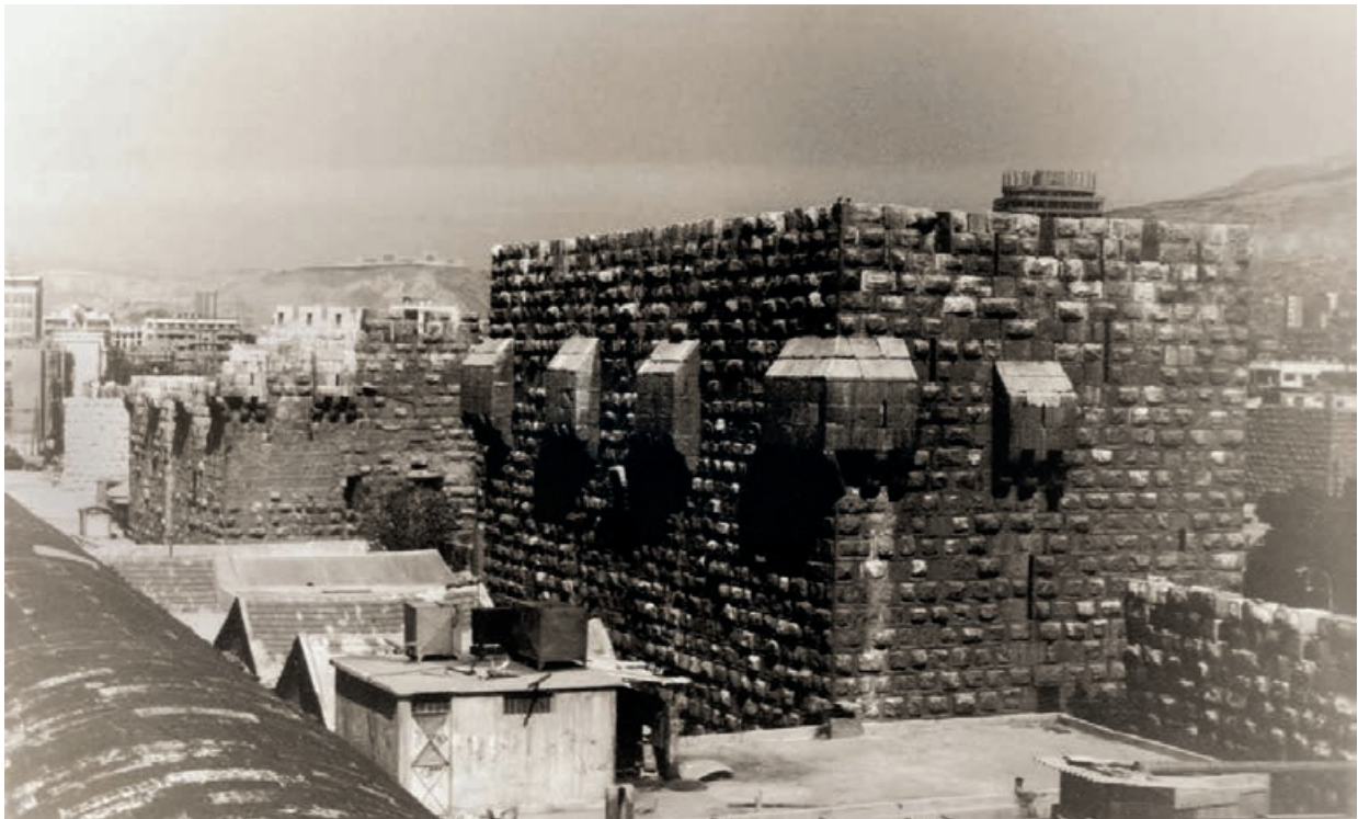
Fig. 7 The citadel of Damascus (courtesy of H. Hanisch, D-DAI-DAM-HP-f-K13-U53-011_SYRHER).
