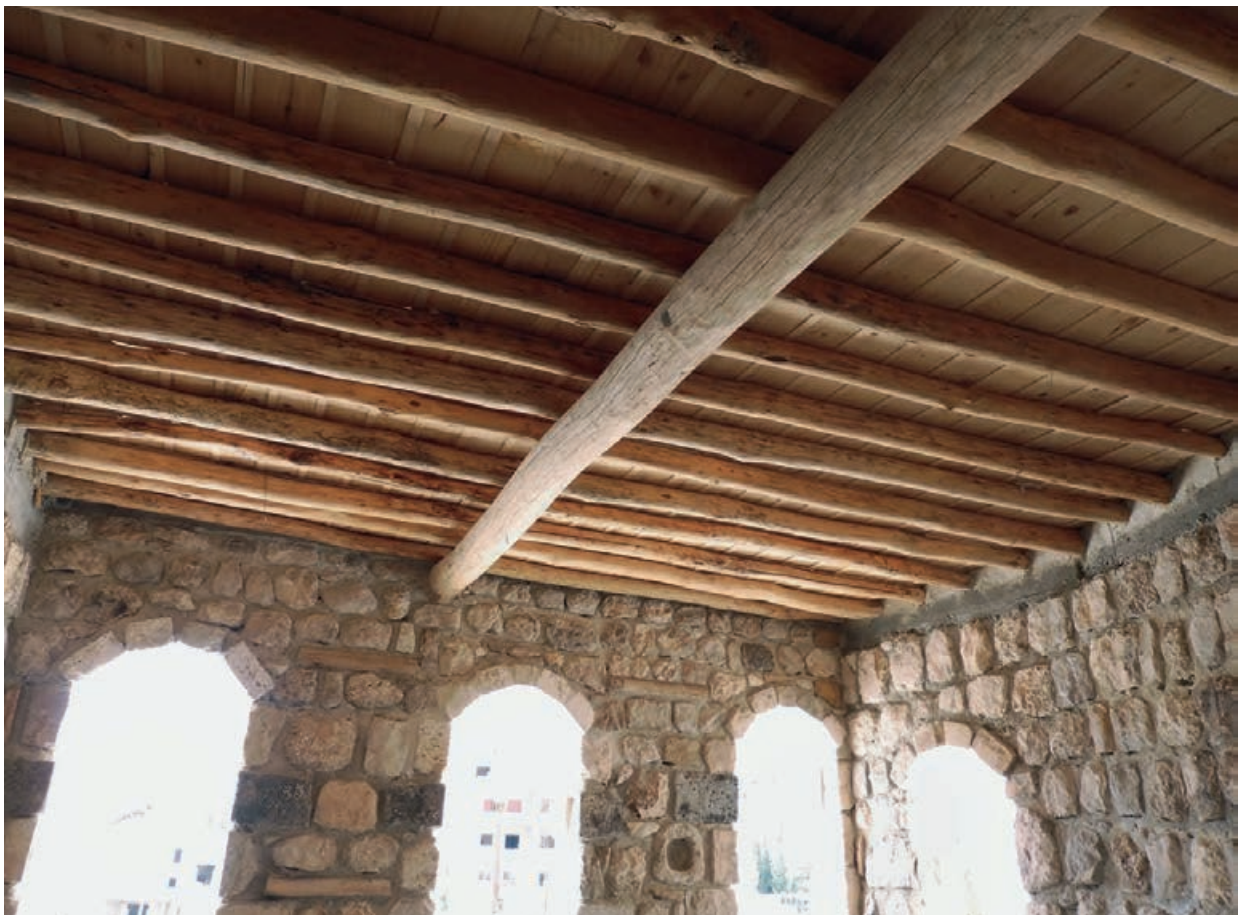
Fig. 12 Maaloula, Reconstruction of a vernacular house, 2018 (© S. Abdulac)
