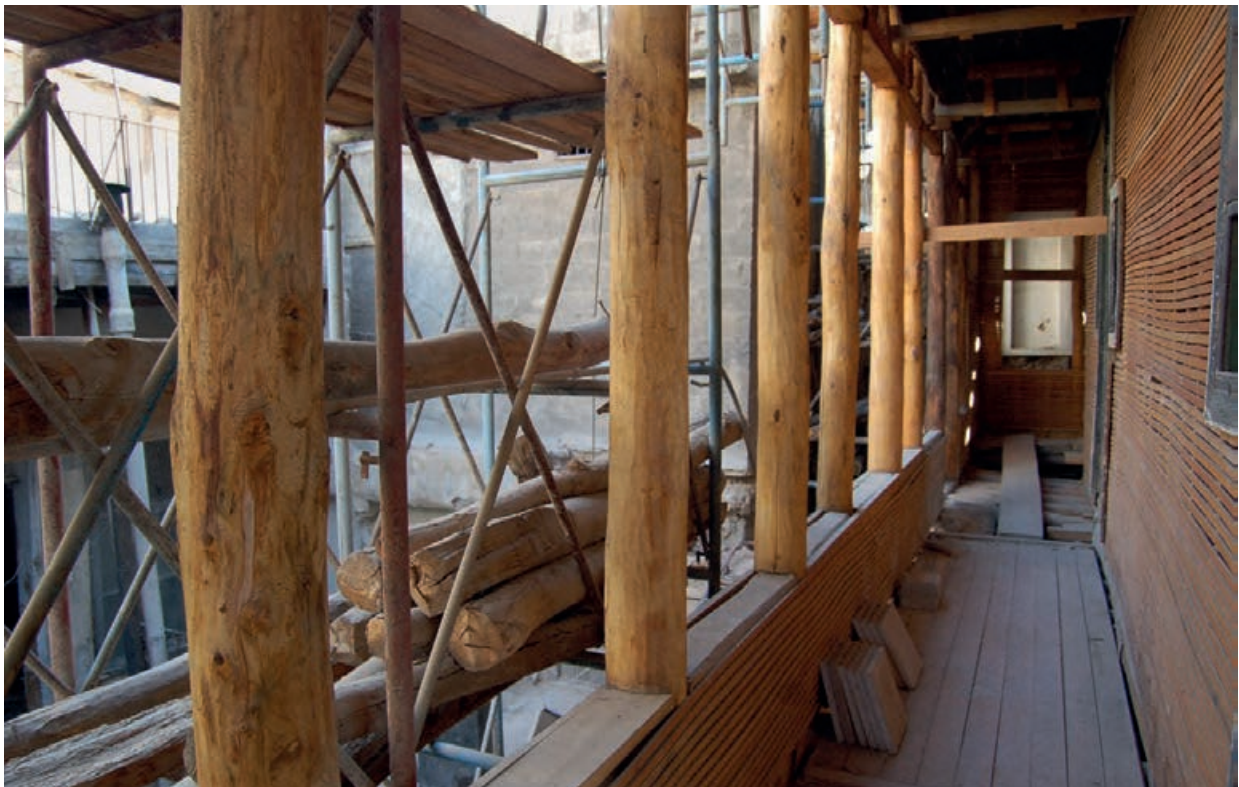
Fig. 8 Damascus, House under restoration, architect Y. al-Jabi, 2001 (© S. Abdulac)
