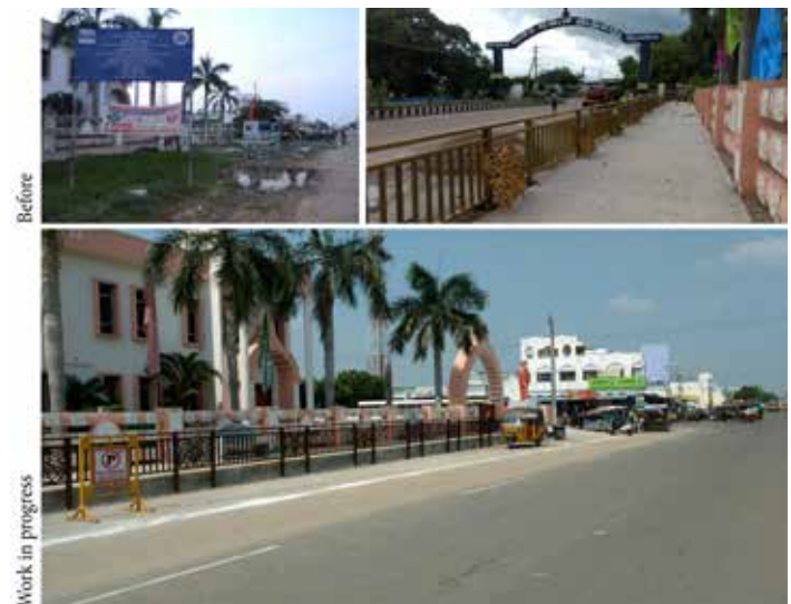
Work in progress as part of Heritage walkway in front of Amaravathi Heritage Centre
