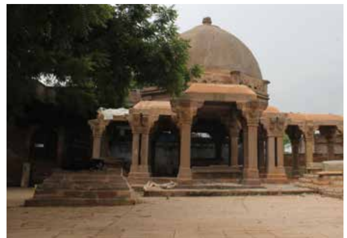
Bhattis Khamba- After Repair
