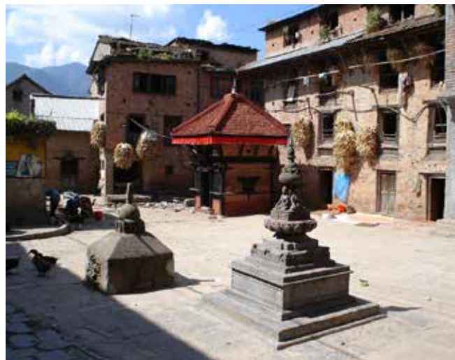
Figure 3 : Traditional interconnected courtyards in the historic town of Patan in Kathmandu valley, Nepal provide safe refuge to people during emergency situations.
