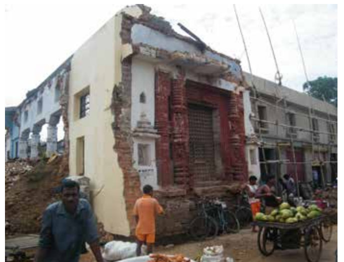
Demolished facade of Emar Matha
