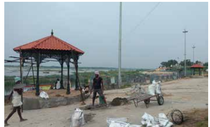
Street furniture under installation
