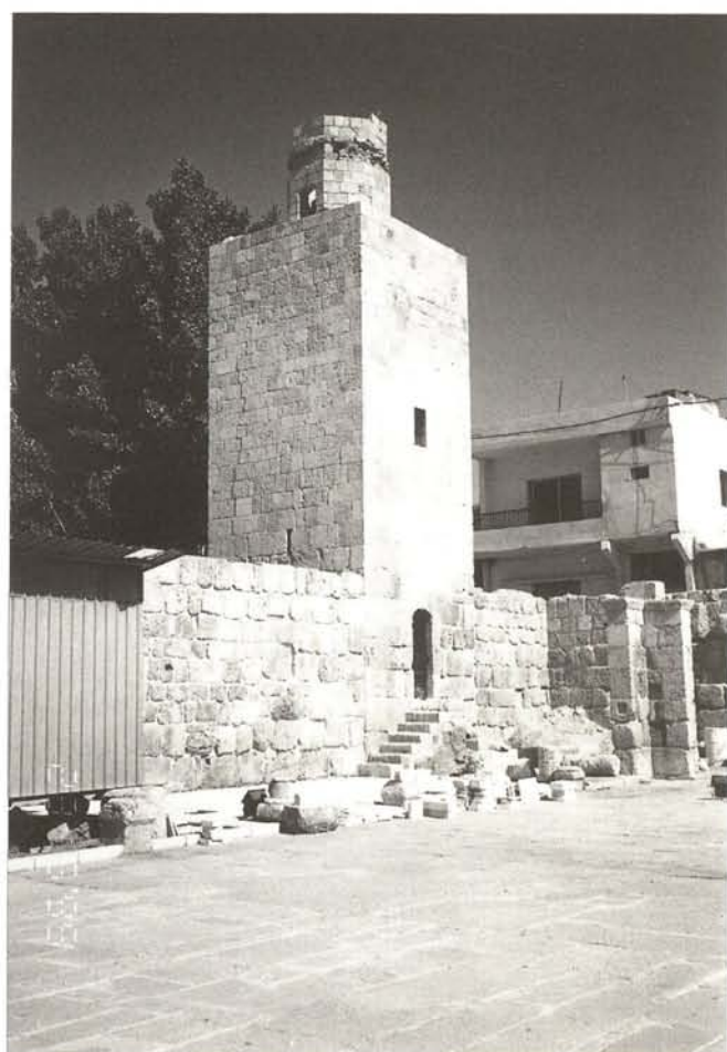
Baalbeck Great Mosque: minaret after restoration work
