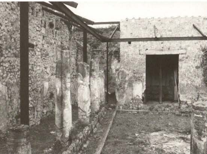
A gap in the protective roof. Ivy has come through and has already grown over the top of the wall.
