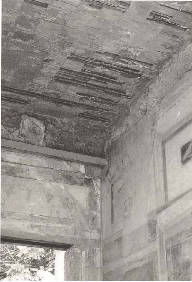
Decay of the modern ceiling construction (brick with iron reinforcements) above the original wall decoration which is already heavily damaged by pervading water (Casa Rebio Valente).
