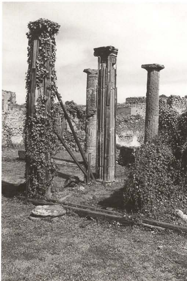
Scanty, temporary conservation measure bracing the columns of a peristyle house. After the earthquake of 1980 endangered houses and constructions were provisionally secured. After 20 years the temporary solutions are still in place, but have corroded or are slowly decaying, since the necessary measures have never been taken. Ivy growth is accelerating the process of decay.
