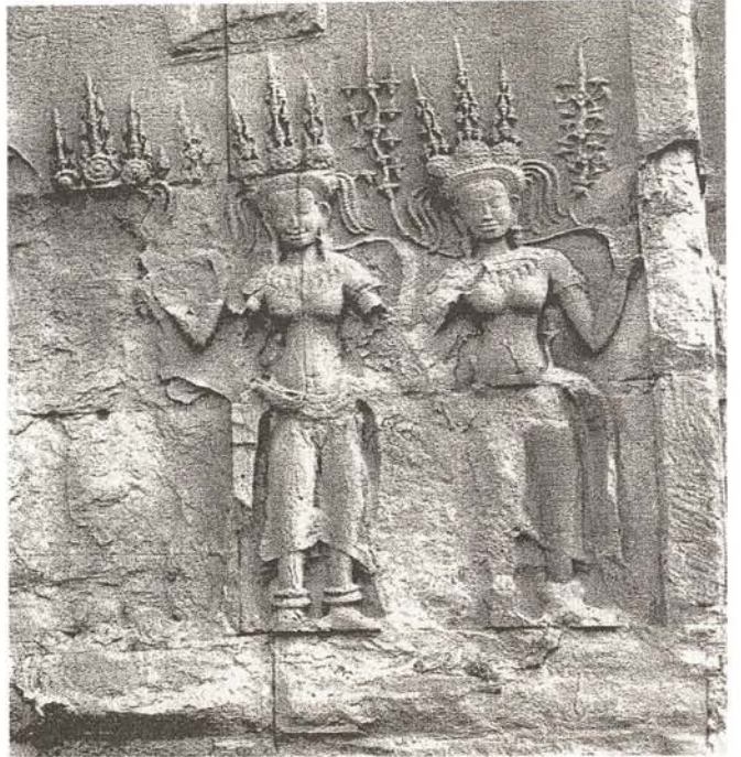
Increasing destruction of the temple reliefs: condition of a relief in 1965
