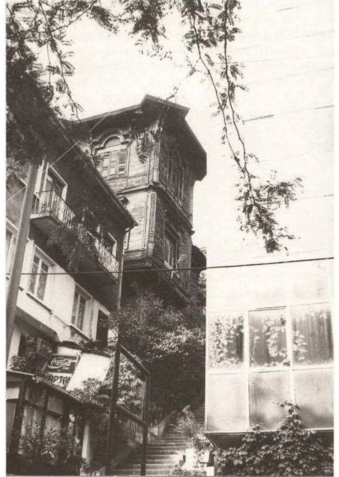
Timber House at Findıklı. The historic districts of Istanbul are destroyed by modern development. The property values are high in central business districts and this creates great pressure on historic buildings. The property developers try to demolish low buildings and build higher modern buildings instead. The timber house in the picture shows the contrast between the old and the new created by the change in scale.
