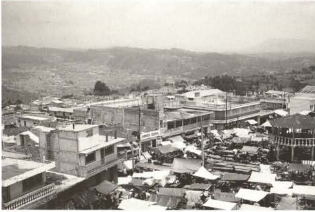
San Francisco El Alto, market place. Almost all the traditional houses have been replaced by new reinforced concrete buildings.
