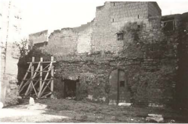
Cimitile, excavation area in the field of the Basilica nova , with masonry that is in danger of collapse and has partly been secured in emergency
