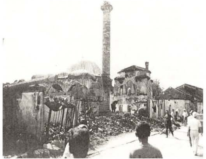
Djakovica, Kosovo – View of the Hadum Mosque, built 1594, amidst the burned – out ruins of the old bazaar historic district. The bazaar was destroyed and the mosque complex suffered extensive damage after being set on fire by Serbian police and paramilitaries in March 1999; the top of the minaret was shot off by Serbian troops using a shoulder-launched missile on May 8, 1999. (Photo: July 1999 by Xhavit Lokaj, Kosovo Cultural Heritage Project, Harvard University)
