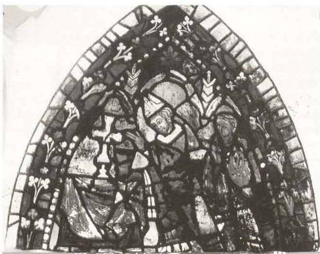
León (Spain), cathedral, exterior and interior view of a stained glass window: the seriously weathered glass surfaces reduce the transparency of the panes.
