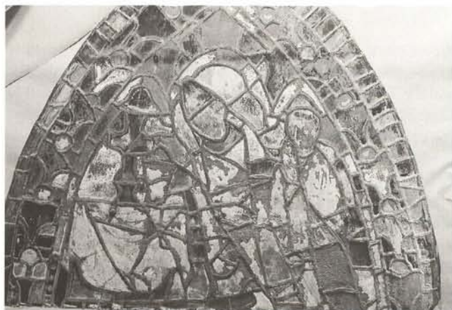
León (Spain), cathedral, exterior and interior view of a stained glass window: the seriously weathered glass surfaces reduce the transparency of the panes.
