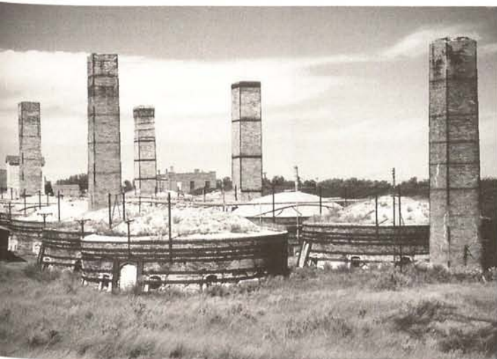
General view of 10 kilns and 5 stacks (1912–37), Claybank Brick Plant national historic site, Claybank, Saskatchewan
