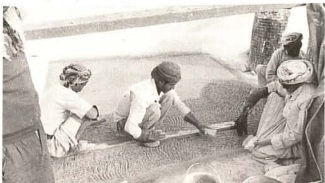
Pounding of a quadath layer
