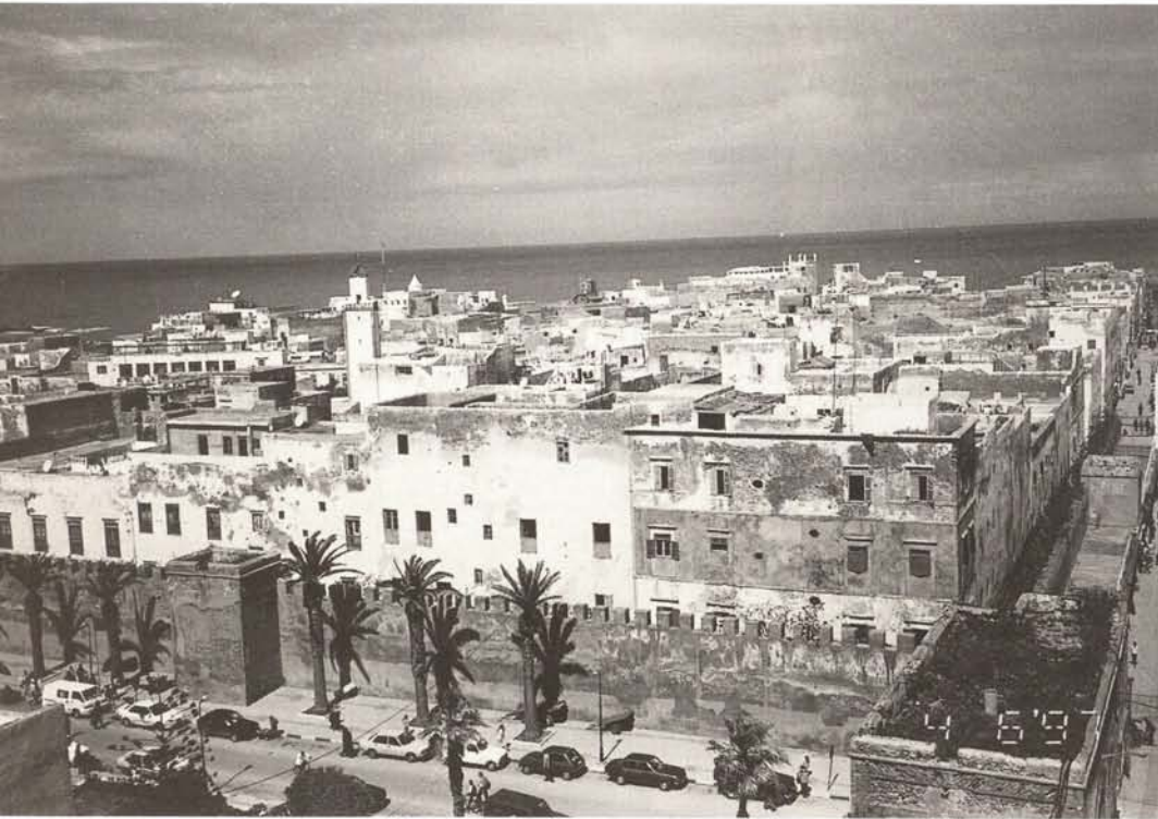
Essaouira (Mogador). Second east wall: rising damp due to surface water and rain water, causing stone surface erosion
