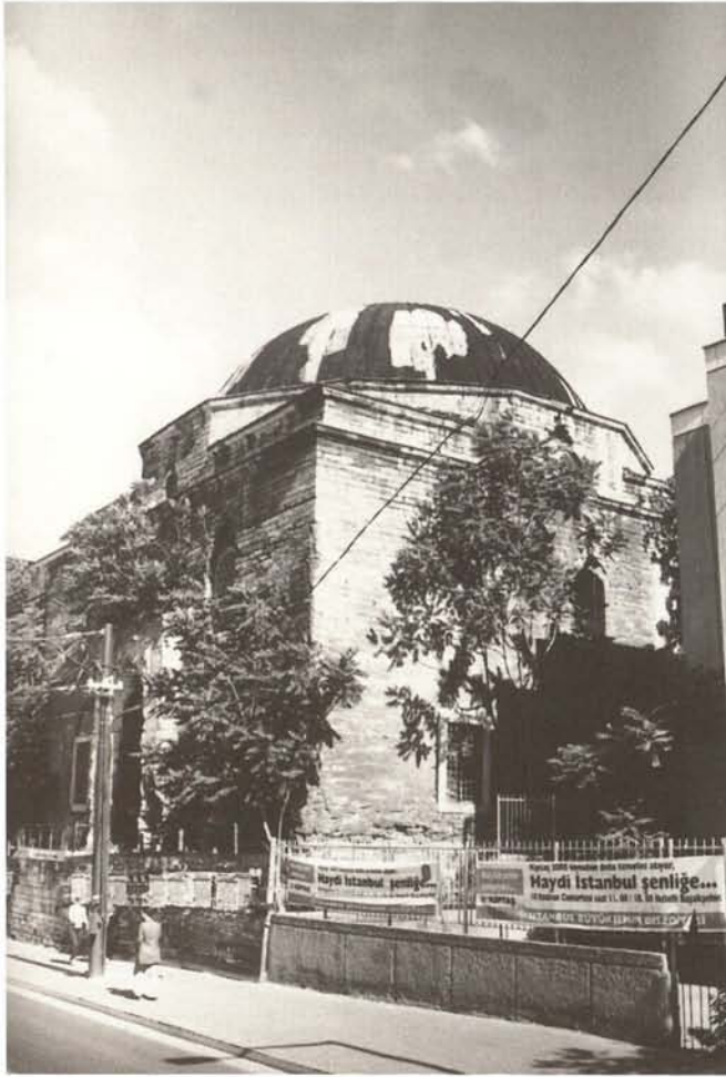
Bath of Bayezit is an early 16 th century building which has not been in use for many years. During the road-widening operation in the 1950's, the street level was changed and the foundations of the south wall were exposed. A crack which had developed earlier on the dome of the dressing hall was widened by the tremors in 1999.
