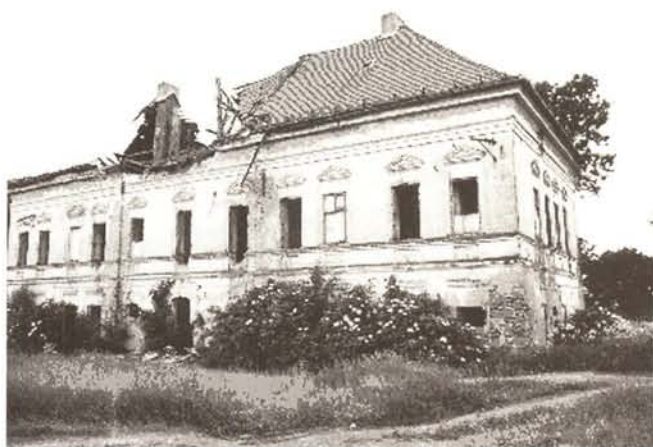
Žip, neo-classical manor house with collapsed roof
