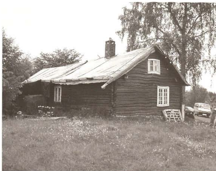
Example for an endangered farmstead, a blockhouse protected by a provisional roof
