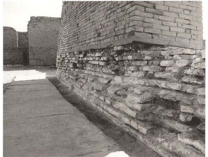
Moenjodaro, salt pater in a burnt brick wall, lower city
