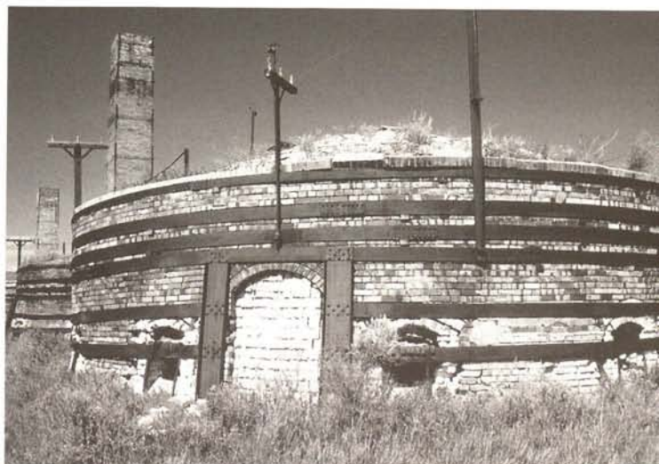
Typical deterioration, Kiln No 5, Claybank Brick Plant, national historic site, Claybank, Saskatchewan
