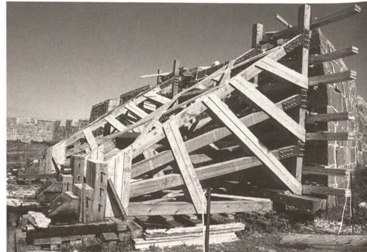
Shoring, Point of the North-West bastion, Fort Prince of Wales, Churchill, Manitoba
