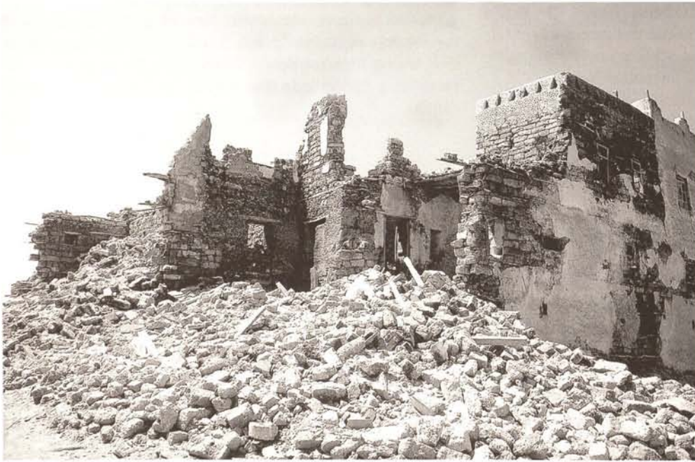
Mirbat, collapsed house
