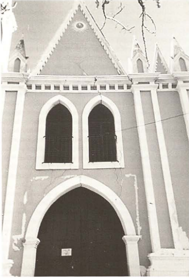
Coro, Iglesia de San Francisco, cracks and general damage due to movements of the earth
