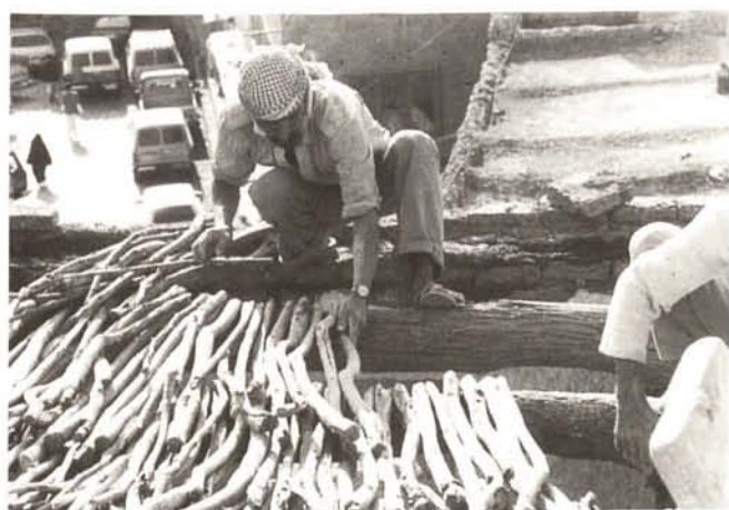
Installation of the brushwood layer for the ceiling
