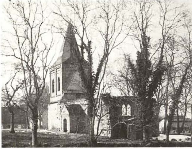
Ruinous village church in Zernin (Mecklenburg)
