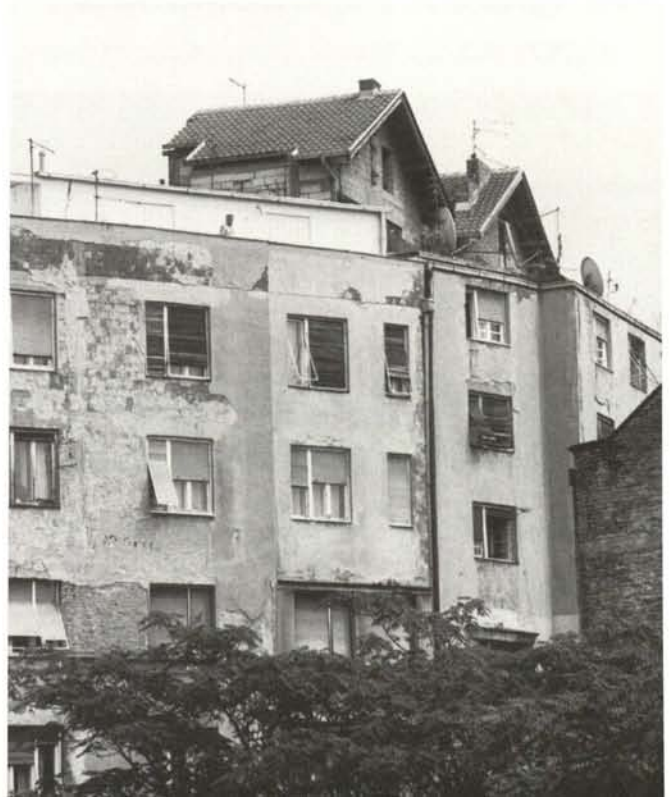
Belgrade, illegal construction in the historic centre
