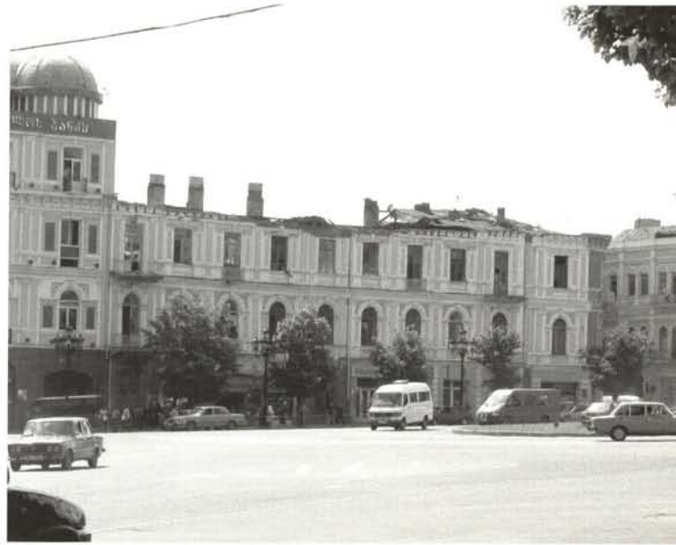
Damaged listed building on the Liberty Square destined for demolition by the city authorities
