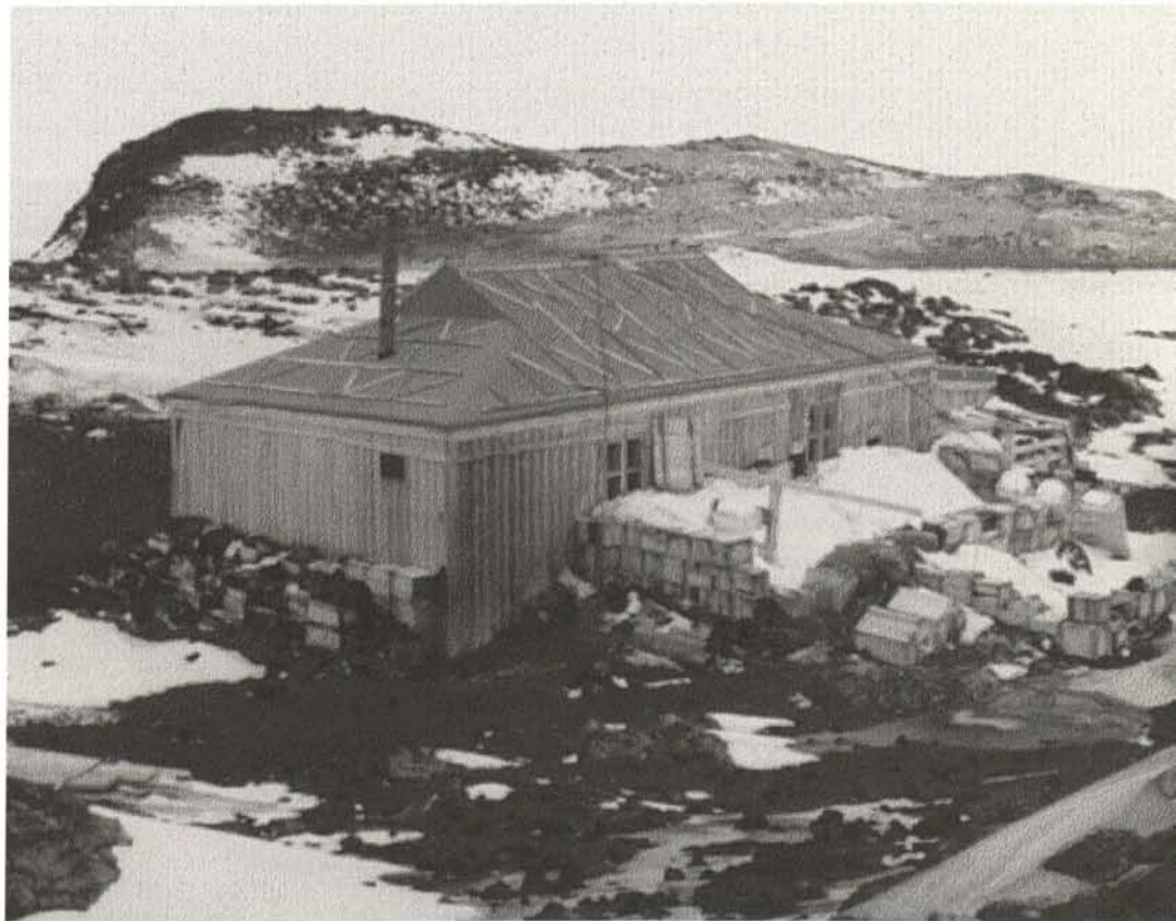
Insulation for this prefabricated building was improved by stacking boxes of supplies around the outside walls and filling the space between with volcanic scoria. Cape Royds, Antarctica. (Photo: P. Chaplin)
