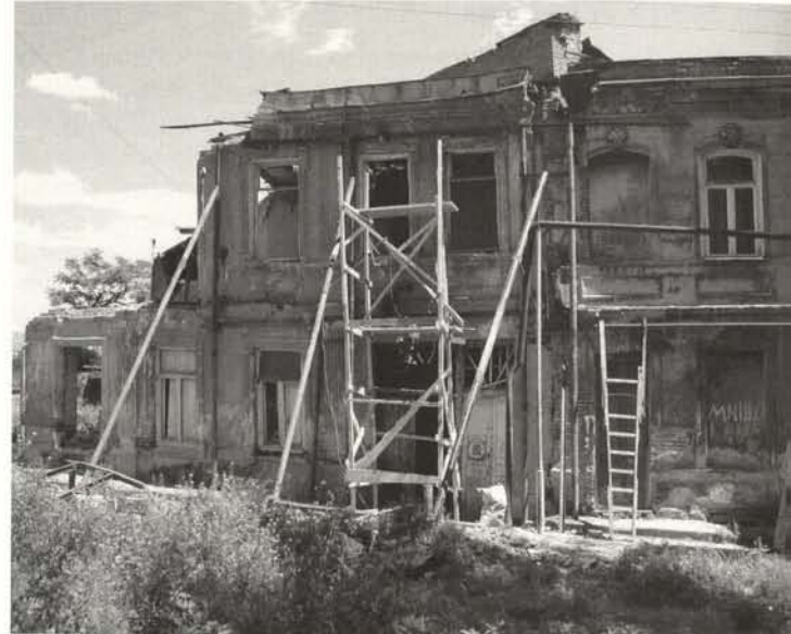
Residential house in Kvemo Kala micro-quarter. Emergency stabilisation after the earthquake
