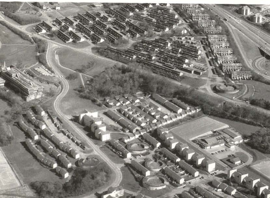
Byker Estate, Newcastle upon Tyne, 1970–81. A section of the main spine 'wall'.
