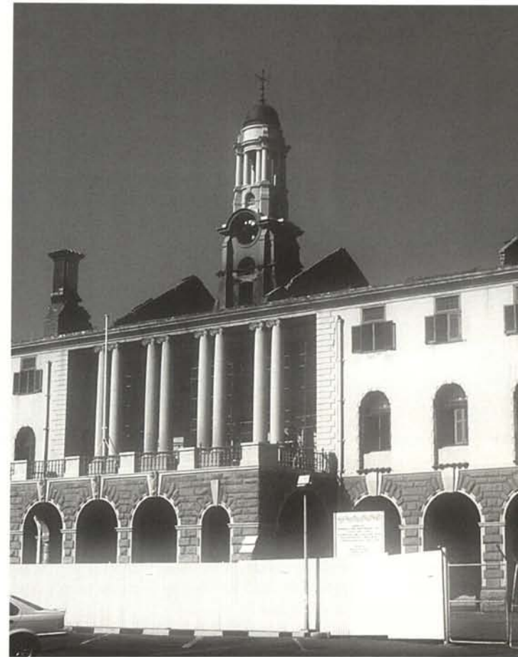
Pretoria's main railway station designed by Sir Herbert Baker and built in 1910–1912. This photograph was taken a few days after the destruction of the roof through fire on 19 February 2001. The fire was started by an angry mob of railway commuters who vented their frustration because of trains running late at evening rush hour. The building has since then been restored. (Photo: R.C. de Jong)
