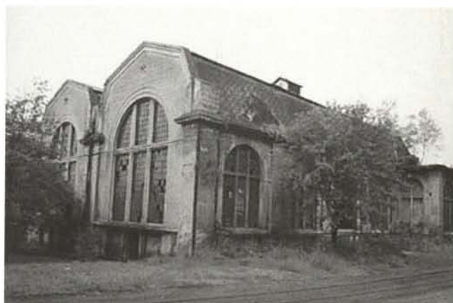
Operating buildings of the František Josef Mine Kladno – Dubí, Central Bohemian Region
