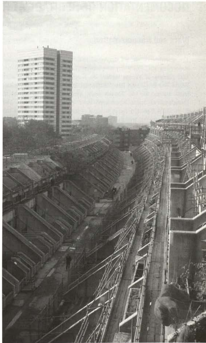
The Alexandra Road Housing Estate in London during the large-scale concrete repair programme in 1998. Attempts to rectify earlier poor repairs and address later problems were difficult to carry out without resulting in a blotchy looking building instead of the sleek, high quality concrete finish of the original concrete. (Photo: S. Macdonald)
