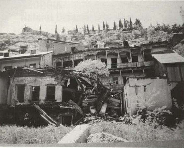
Residential buildings after the earthquake
