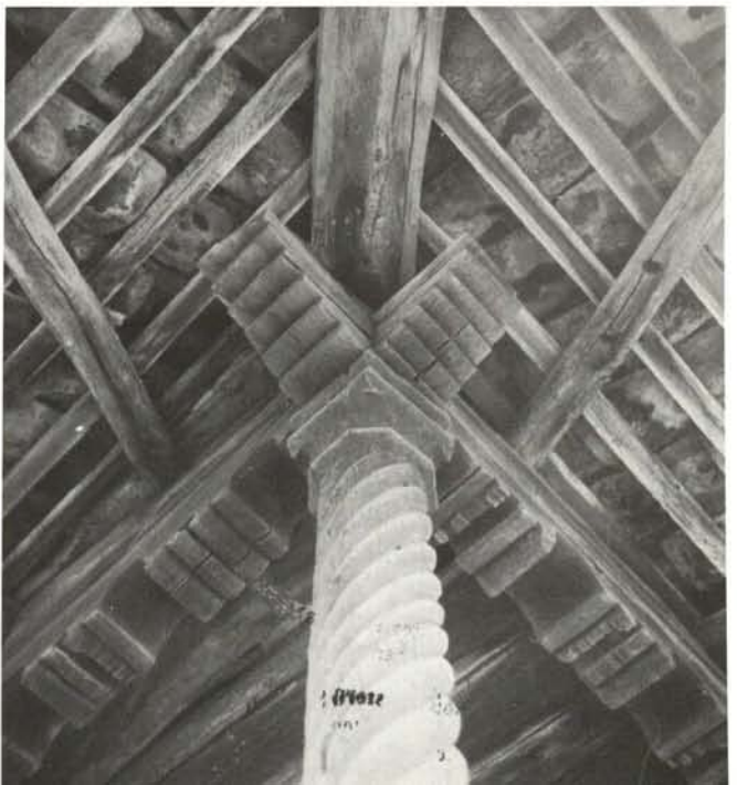
Village of Sičevo (Eastern Serbia), roof construction of the granary, detail
