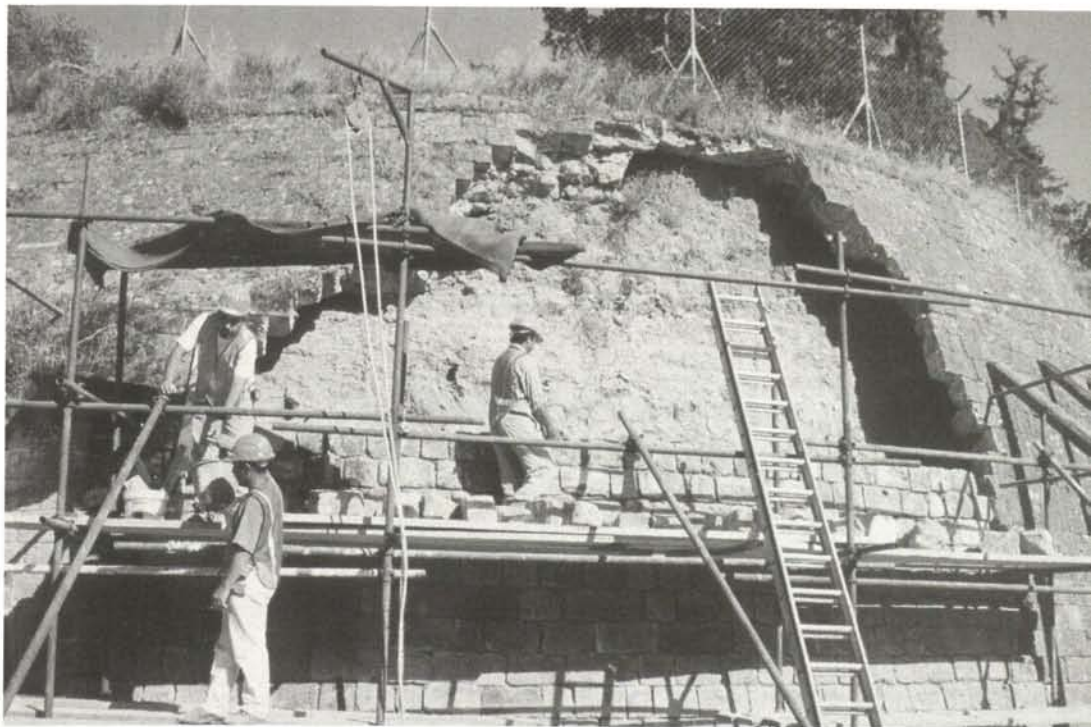
The Roccas bastion during conservation work
