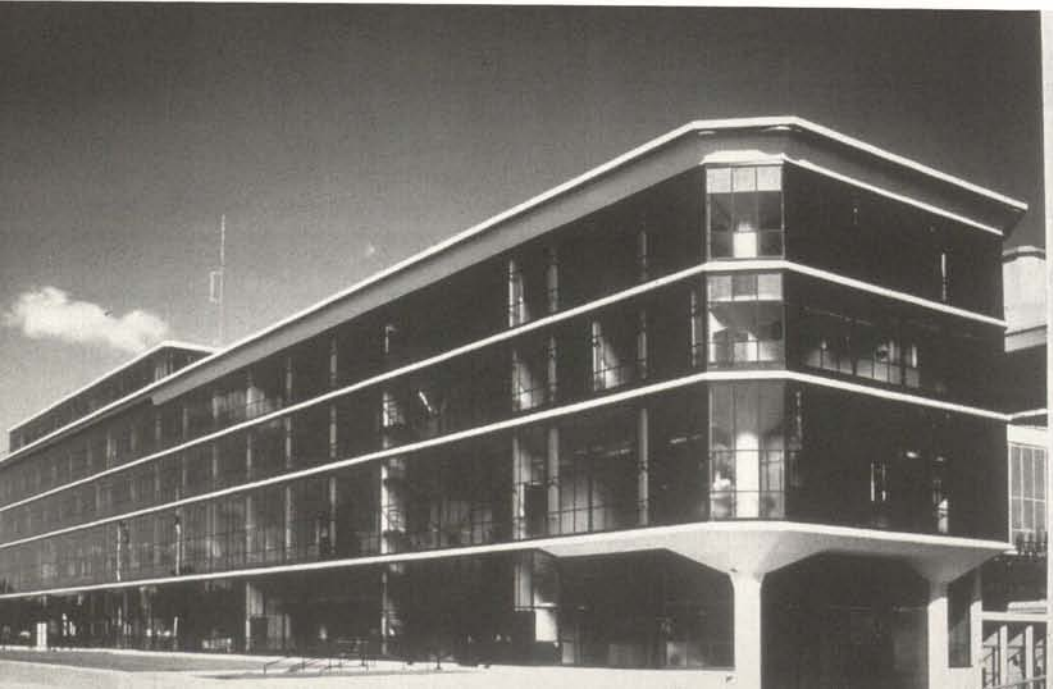
The D10 building of the Boots Factory in Nottingham, England, after major conservation works in the 1990s (Photo: S. Macdonald)
