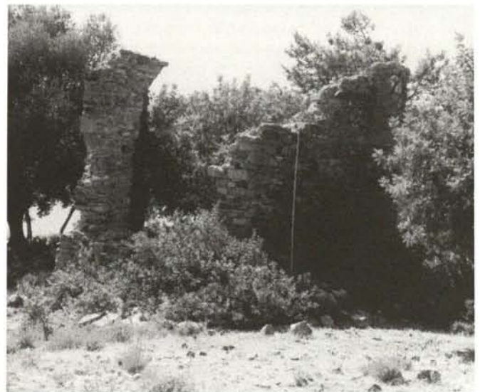
Ala Kilise II, basilica – polygonal apse, view from the east
