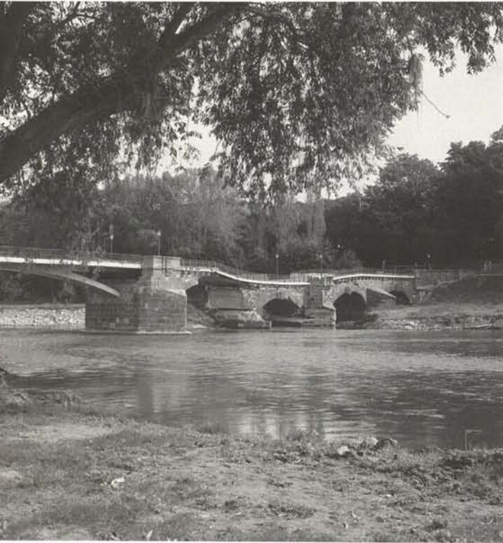
Grimma, damaged historic bridge
