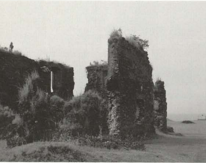
Castle of San Lorenzo. World Heritage (deterioration through lack of maintenance, Nov. 2002).
