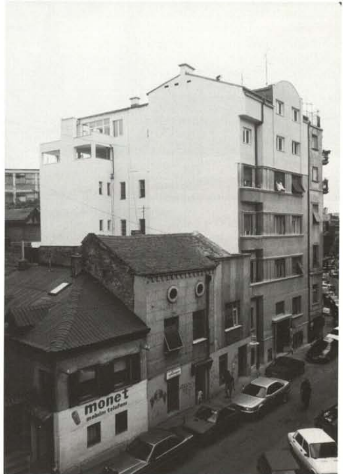
Belgrade, inappropriate addition in the historic centre
