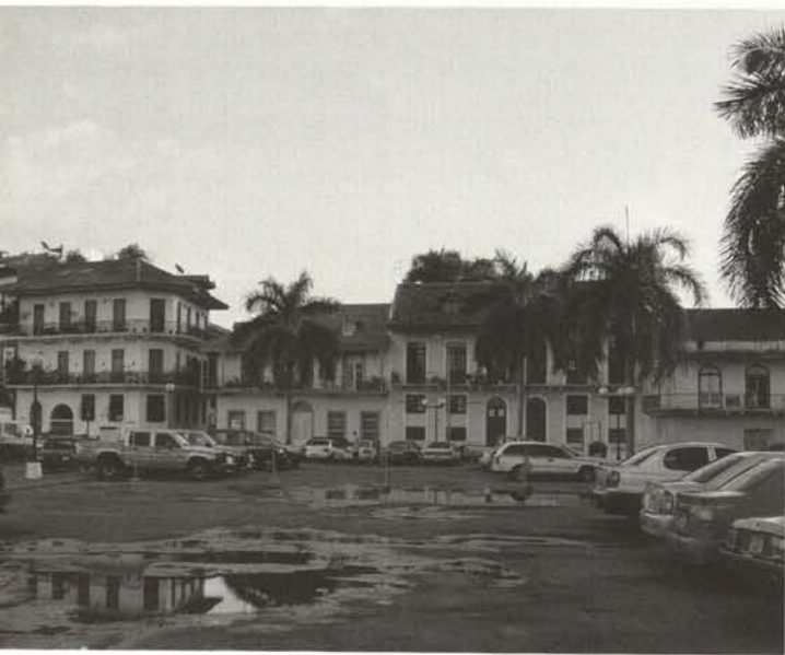
Restored houses, historic centre. World Heritage (successfully restored houses, Nov. 2002).
