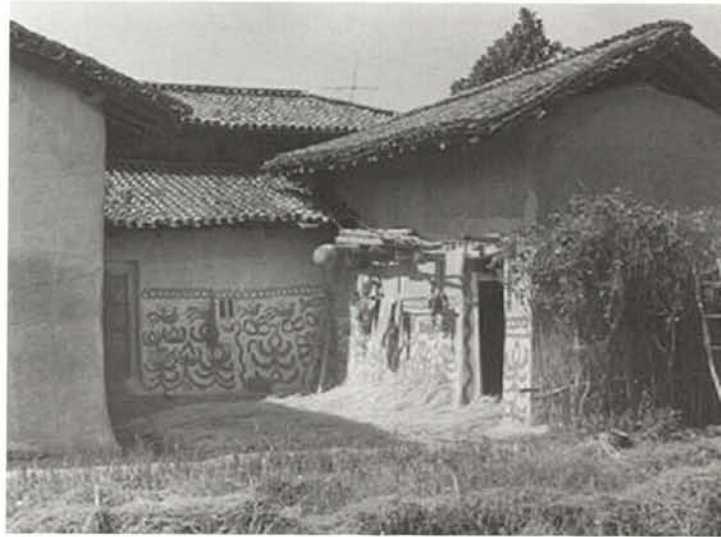
Vernacular architecture in the North Karanpura Valley
