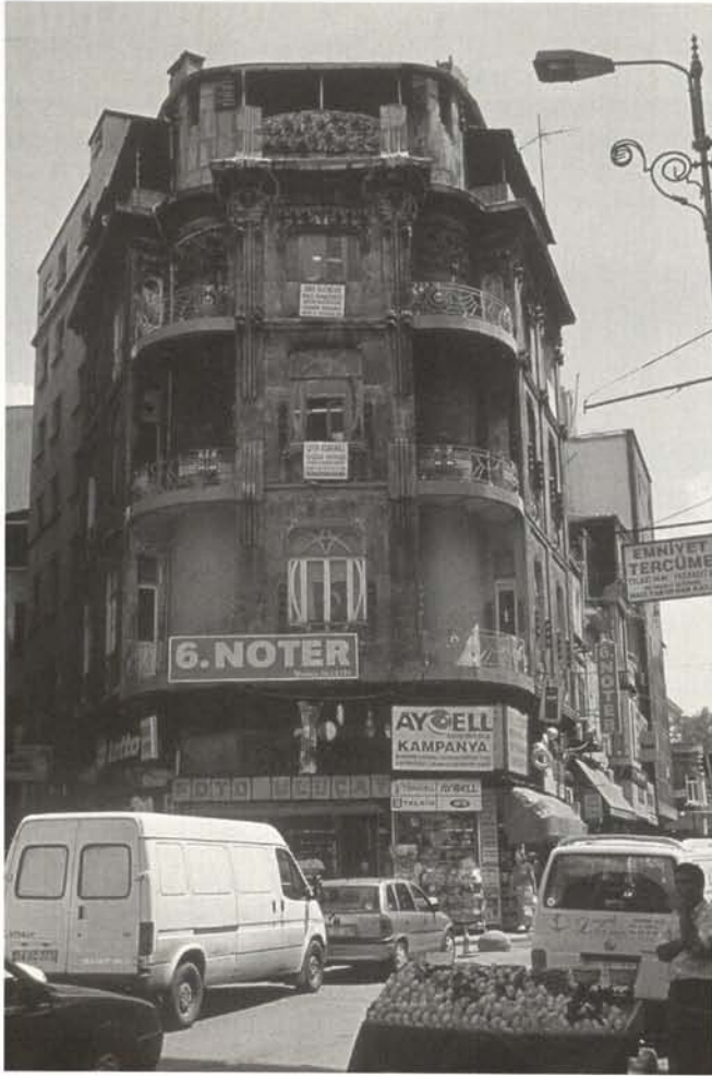
Vlora Han is a beautiful Art Nouveau office building at Sirkeci, within the commercial centre of historic Istanbul. The crowd of advertisements on the façades and alterations to the shopfronts make it difficult to appreciate the beauty of the building.
