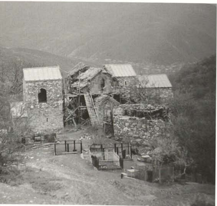
Kanchaeti Kabeni Church, general view after the earthquake
