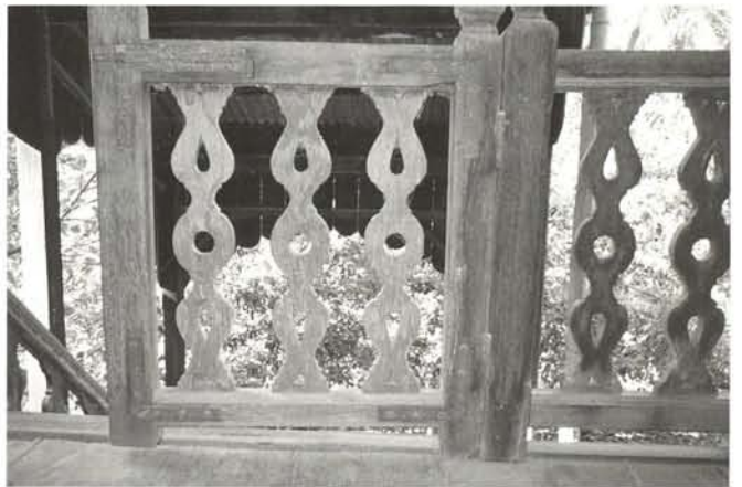
Guardrail, house in Battambang
