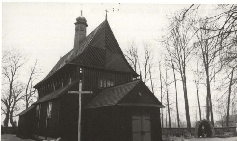
Długa Kościelna, the wooden church built at the beginning of the 17th century (before fire). Burnt in 2001, the fire was probably set deliberately.
