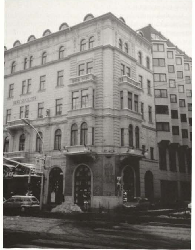
An accomplished façadism of a Budapest hotel
