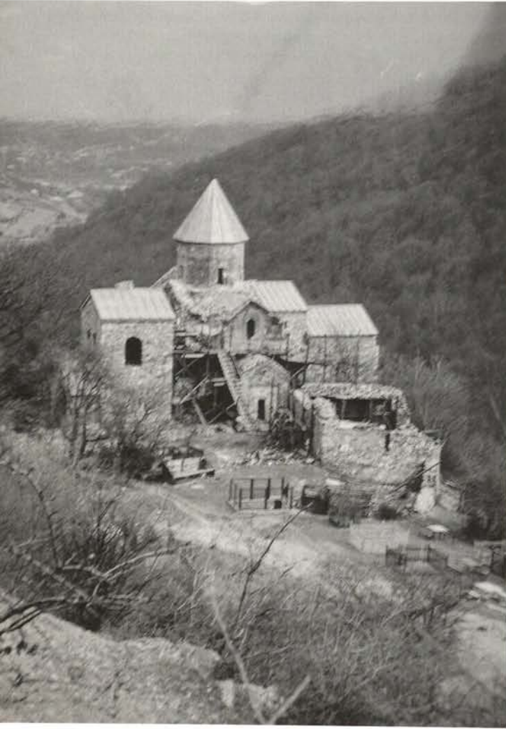
Kanchaeti Kabeni Church, general view before the earthquake
