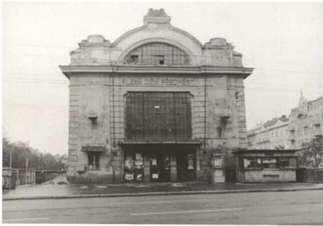
The main building of the railway stop, Plzeň – southern outskirts
