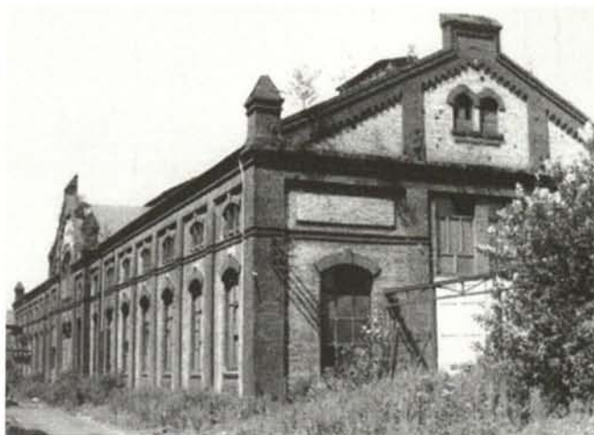
Workshop building of the coking plant Karolina, Ostrava, North Moravian Region
