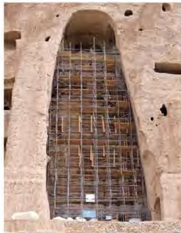
Niche of the Eastern Buddha with scaffolding (photo: B. Praxenthaler)
