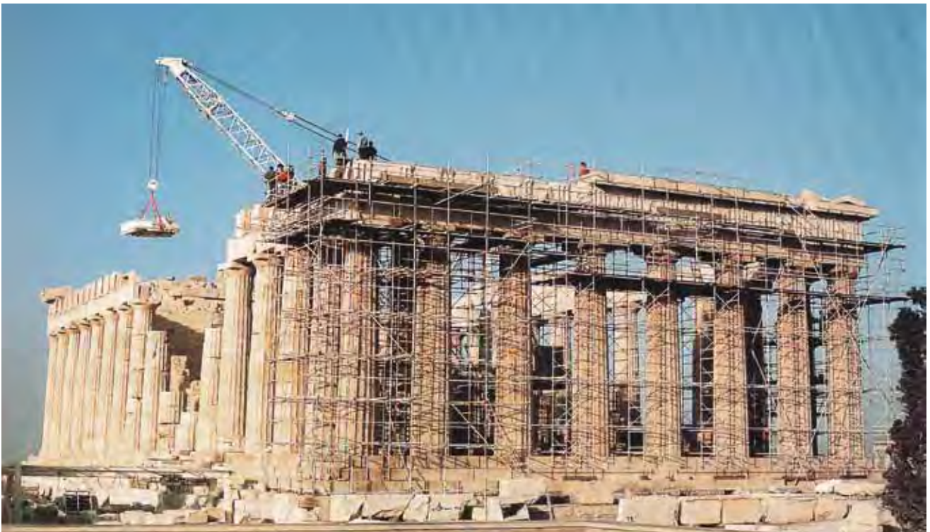
Parthenon, remantling the southeast corner of the cornice
