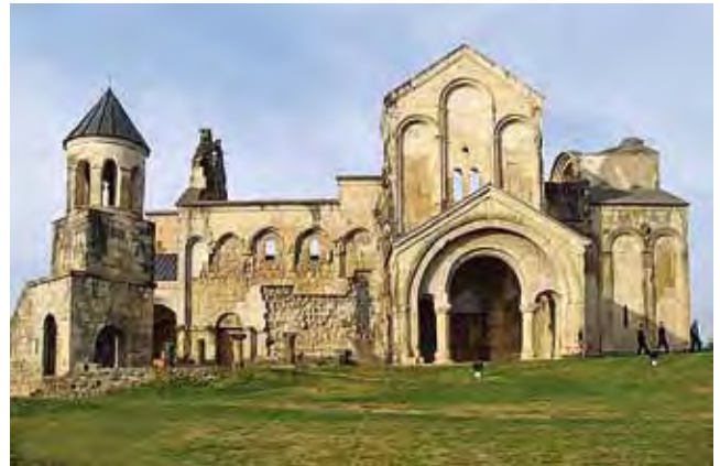
Bagrati Cathedral before the intervention
