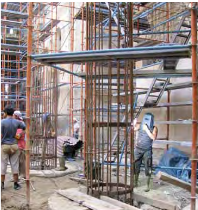
Bagrati Cathedral, the interior during reconstruction works, 2009
