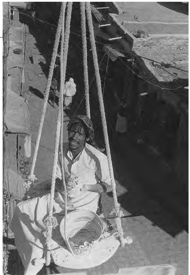
Plasterer on a hanging platform
