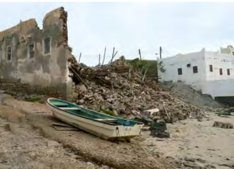
Mirbat (Oman), damage caused by a rainstorm, 2007
