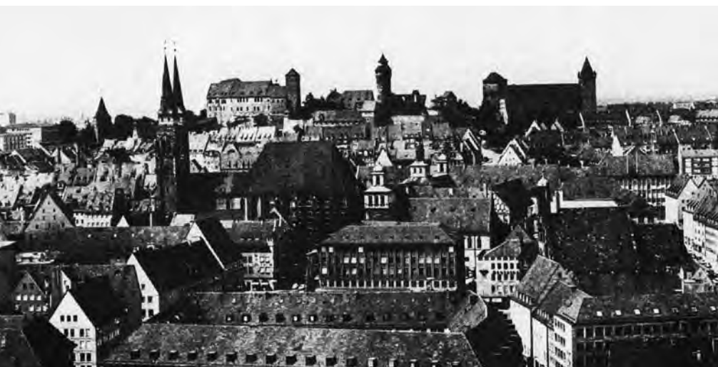
Old town with St. Sebaldus Church and Imperial Castle after rebuilding (below)
