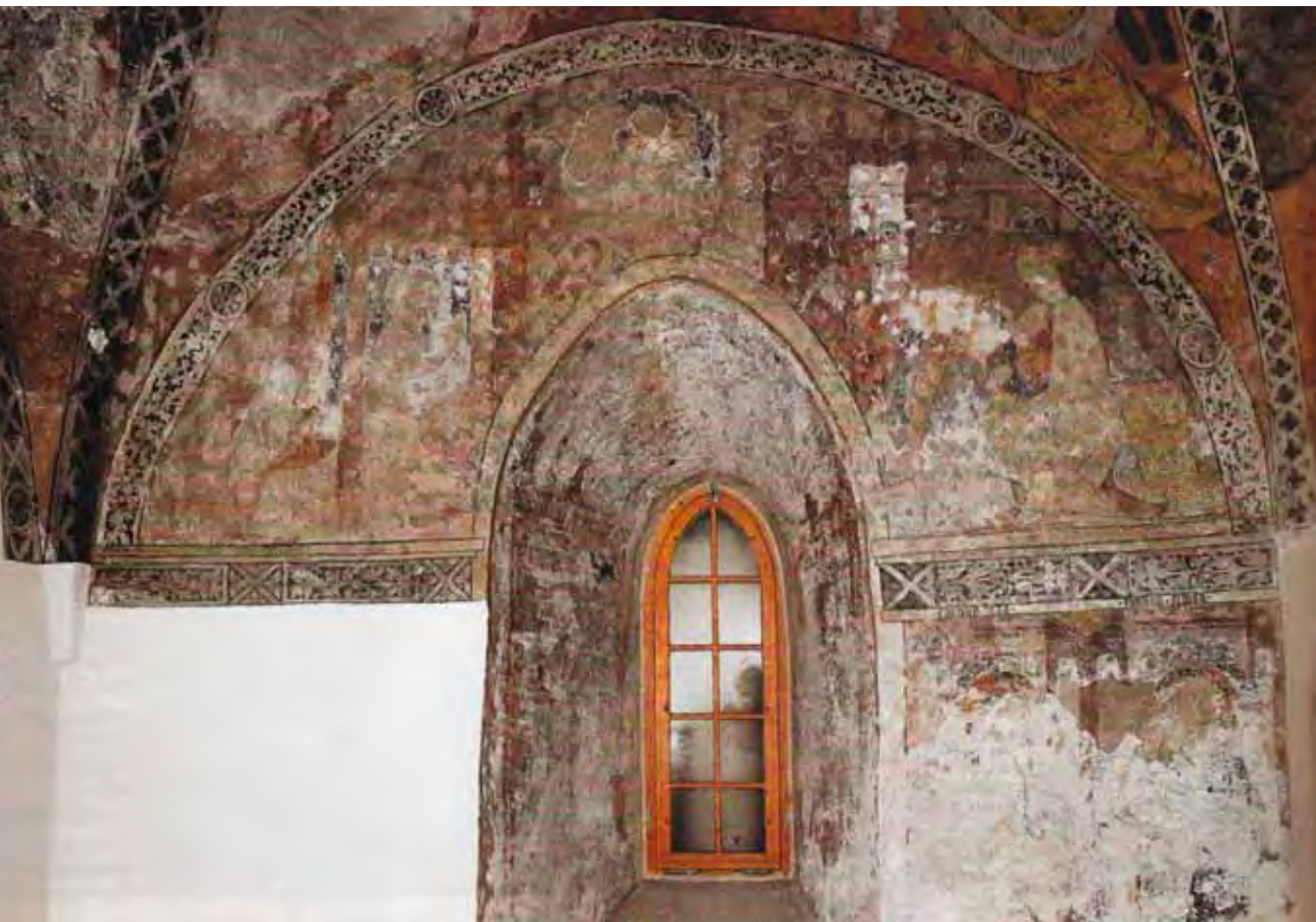
Masans, southwest wall in the chancel, precondition of the paintings discoloured by overpainting and burnt glue fixations (1996)
