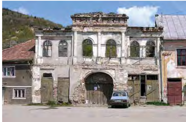
Roşia Montana (Romania), ruined façade in the small mining town that is intended to fall victim to a disastrous project of the Roşia Montana Gold Corporation (cf. "Hope for Roşia Montana?", in: Heritage at Risk 2006/07, pp. 128–130)
