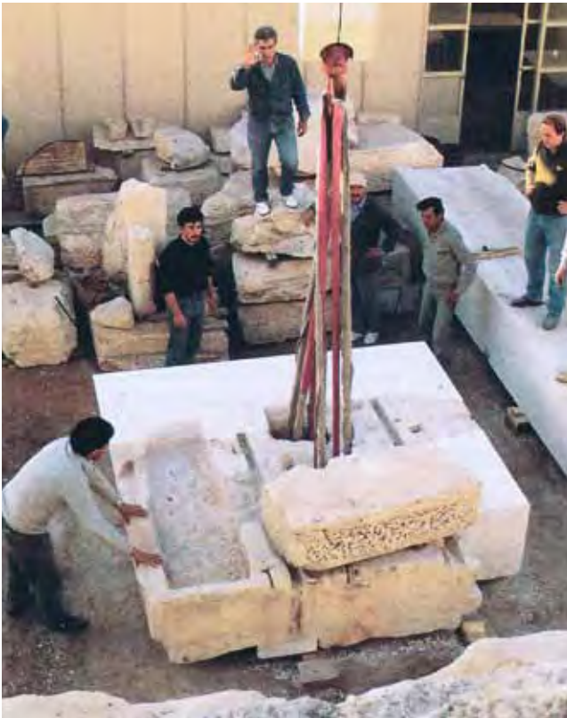
Parthenon (Athens), dismantling of a metope of the eastern façade
