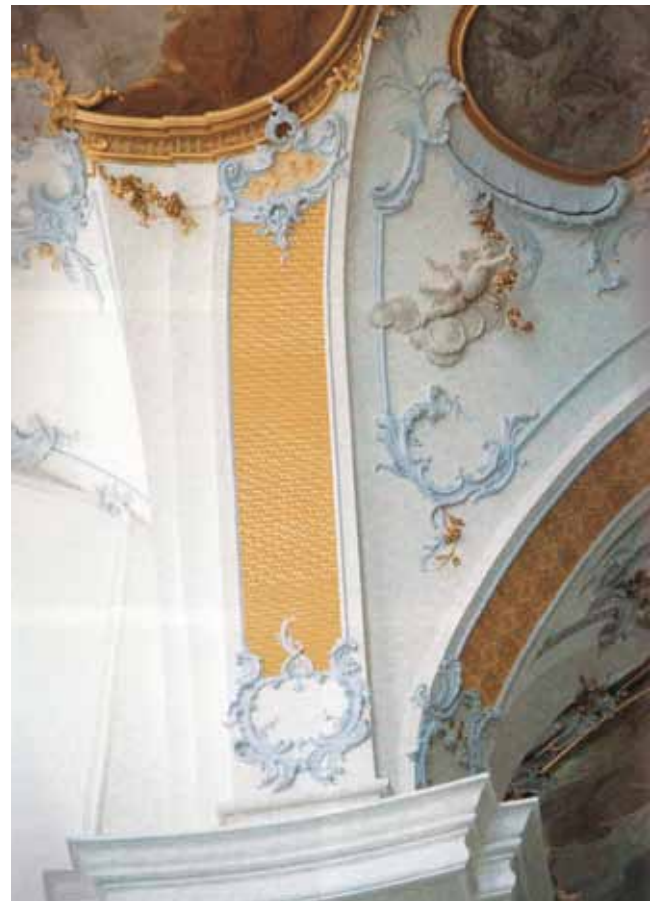
Vierzehnheiligen, colouring of the vaults, condition after the restoration
