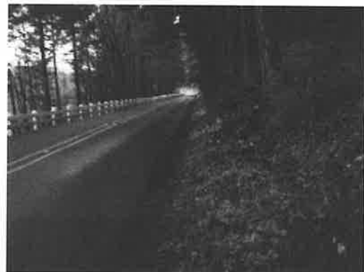
HCRH, Gutter Restoration
