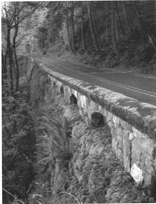
HCRH, Approaching Shepperd's Dell Bridge
