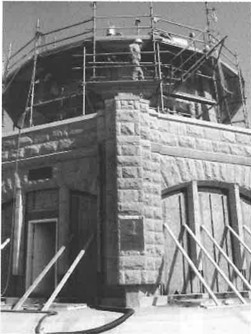
Vista House Restoration 1
