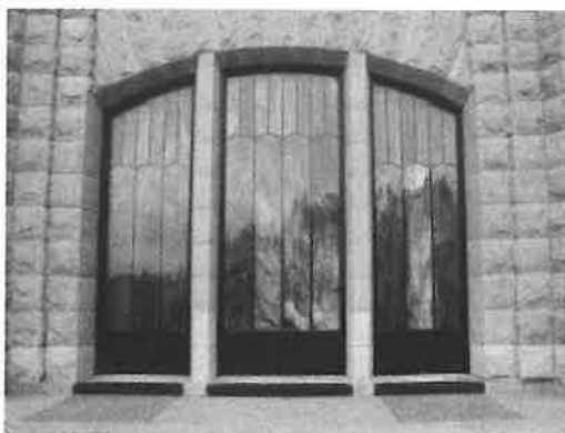
Vista House Restoration 4
