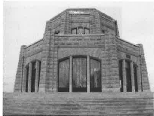
Vista House Restoration 3
