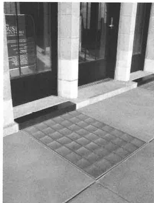
Vista House Restoration 2
