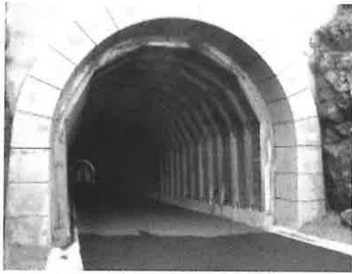
HCRH, Twin Tunnels 1
