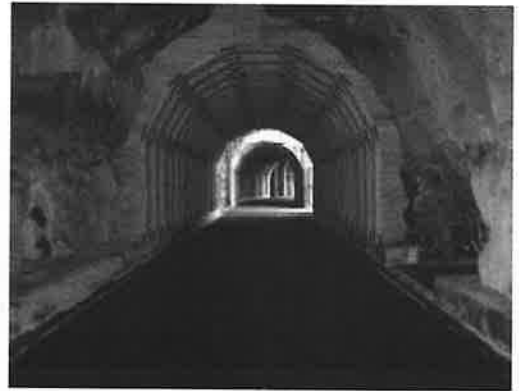
HCRH, Twin Tunnels 2
