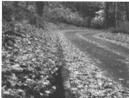
HCRH, Gutter Restoration, Figure Eights
