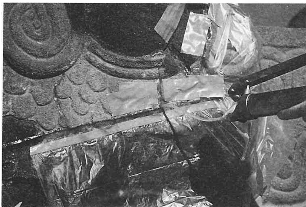
Fig. 8 Injecting epoxy resin into a opening of the relief stone.
