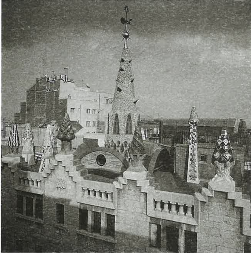
Fig. 1. Roof of the Palau Güell after the restoration
