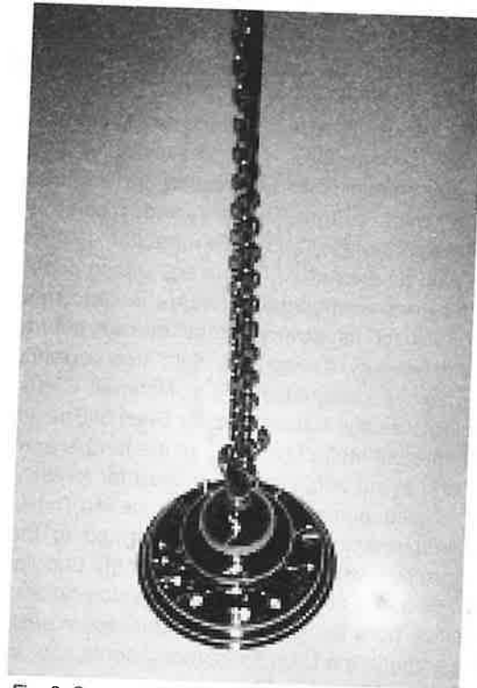
Fig. 2. Canopy of 17th century chandelier drilled to allow glass tails to lights paintings around a room
