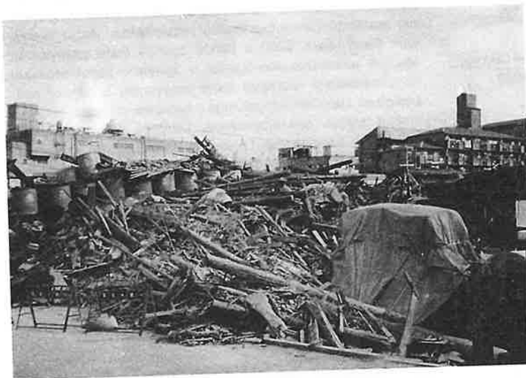
Fig.3 The collapsed warehouse of Fukuju Sake Brewery Inc.,in Higashinada-Ward, Kobe. wooden construction, late 19c. Ninety percent of brewery buildings of this kind collapsed. COPLAN PHOTO
