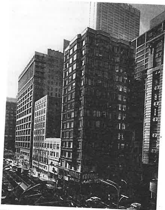
Fig. 17. The Reliance Building before Restoration: 1971
