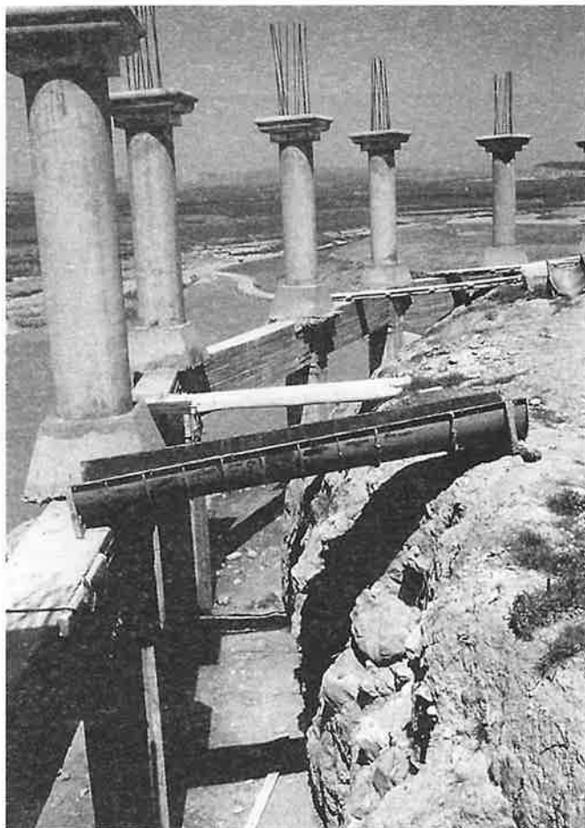
Fig. 9 Reinforced concrete columns which were connected each other
