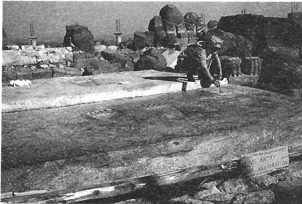
Fig. 11 Impregnating silicone resin in the footmark stone
