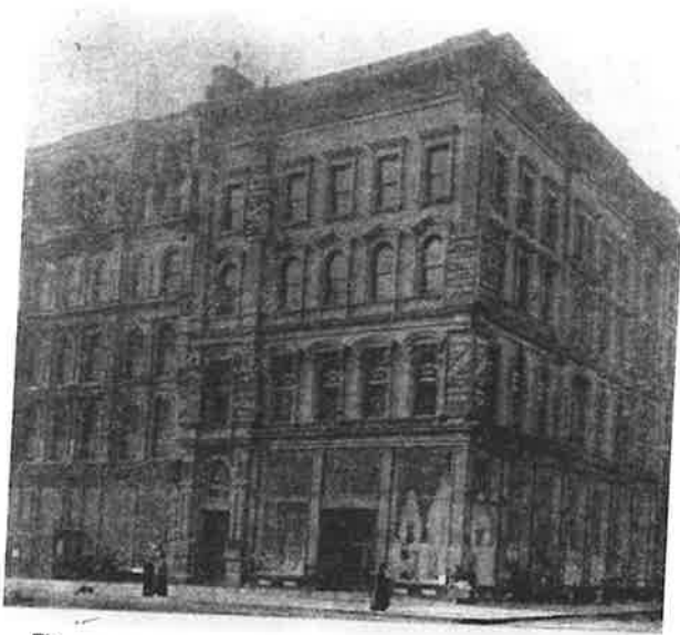
Fig. 15. The Reliance Building Masonry Structure on Top of New First Floor: 1891
