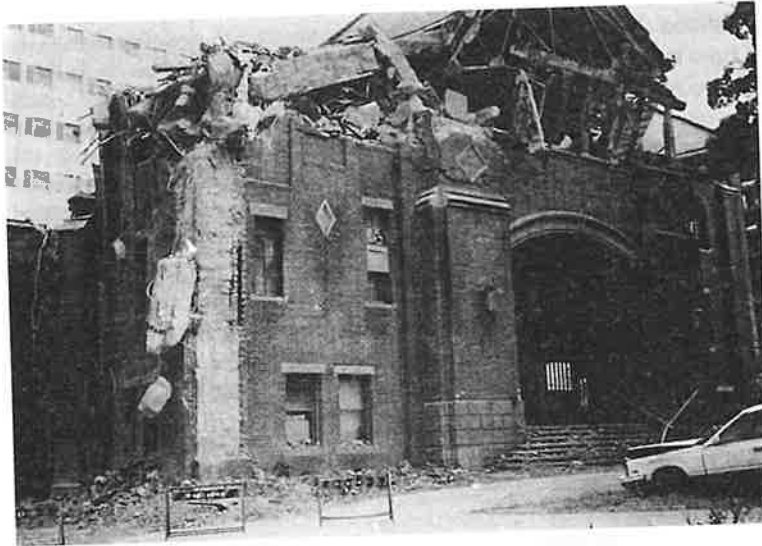
Fig.2 The remains of the Shimoyamate Catholic Church in Chuo-Ward, Kobe, built in 1910. Brick construction. The remains were cleared shortly after the earthquake. COPLAN PHOTO
