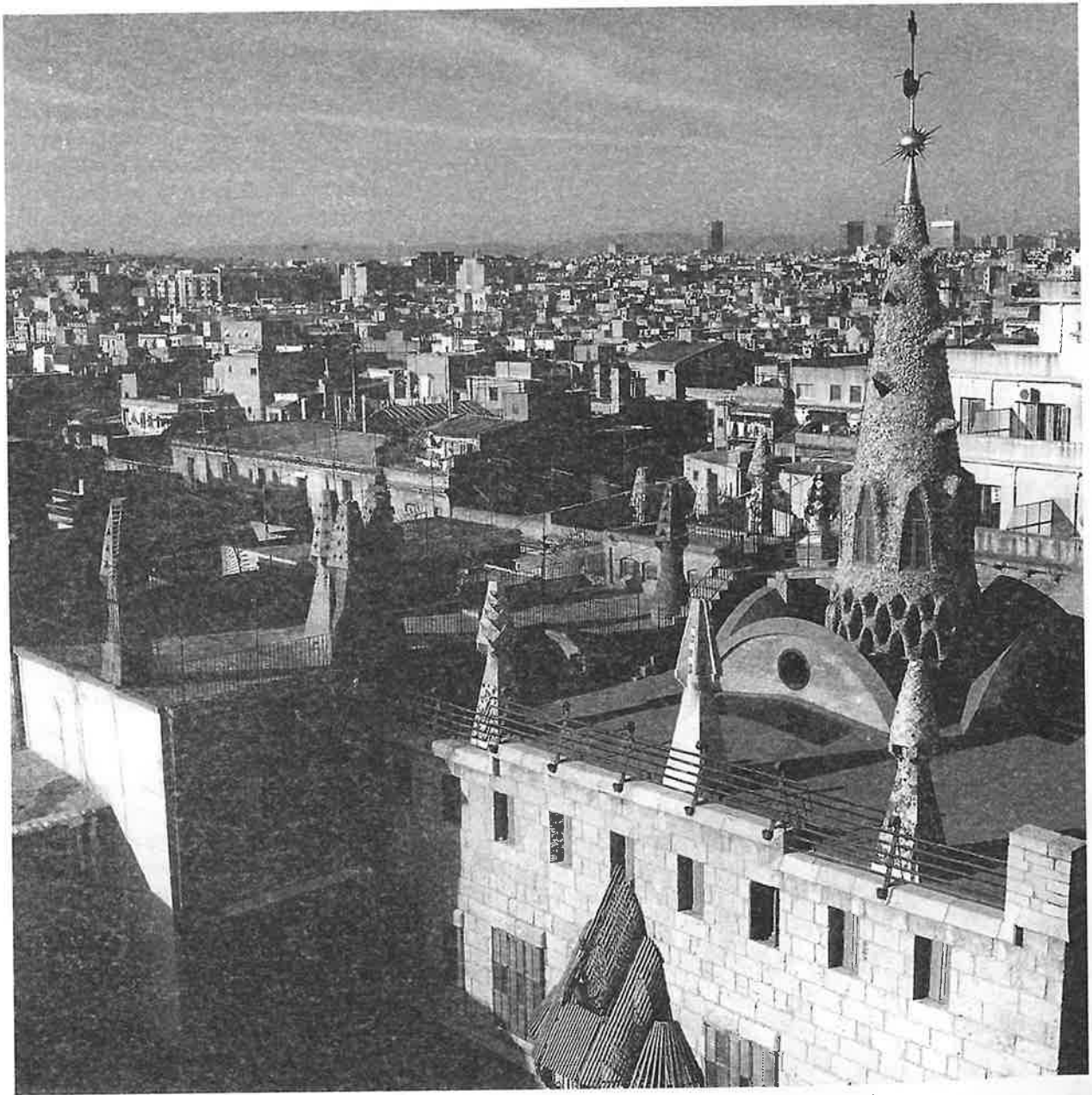
Fig. 3. Roof of the Palau Guell after the restoration. General view from the east
