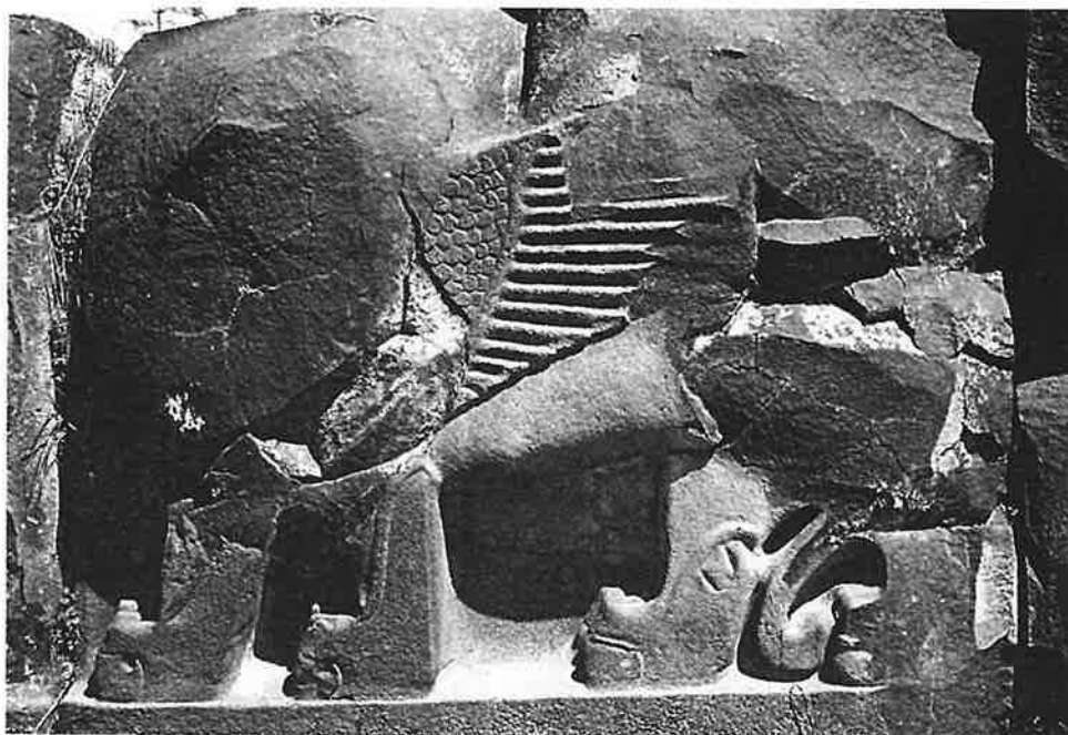
Fig. 5 Deterioration in progress appeared on the relief stone
