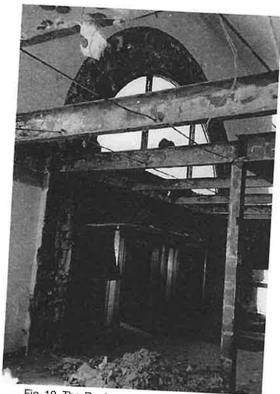
Fig. 10. The Rookery La Salle Street Lobby under Demolition: 1989
