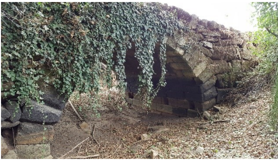
Fig. 87 S. Lourenço Bridge, in Chaves (source: photo of the author).
