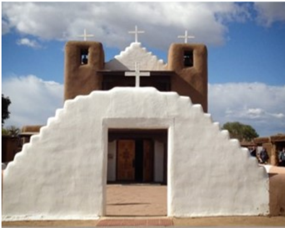
Fig. 16 Example of melding of indigenous and Hispanic adobe architecture, Taos, New Mexico, USA
