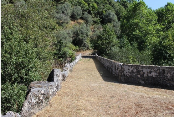
Fig. 85 Mediaeval Bridge, in Vieira do Minho (source: photo of the author).
