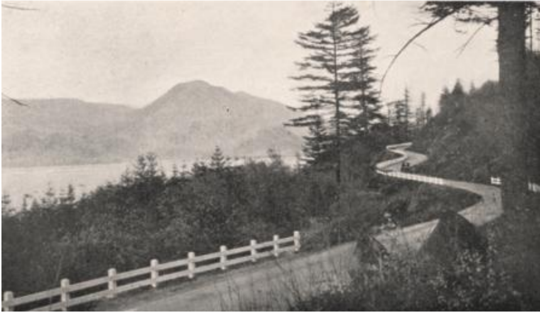
Fig. 1 A portion of the Columbia River Highway, east of Cascade Locks in Hood River (William Calder 1924 - National Library of Australia)
