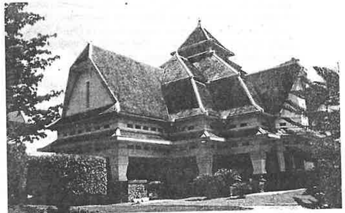
A house in the Darmo area, Surabaya, built in 1923 by Job & Sprij Architecture Bureau Surabaya. The roof form reminds us to roof forms of Indonesian traditional architecture. Terrace around the house providing shadows and holes on the buildings facade for cross ventilation become special features of the Dutch colonial architecture in Surabaya.
