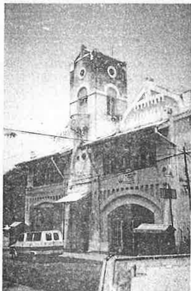
Two examples of colonial heritage buildings at the Harbor of Cirebon
