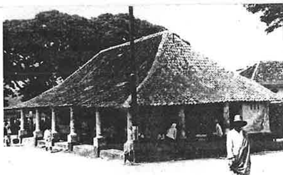
The Arya Jipang House at Palmerah, Jakarta in 1949. The building has since disappeared.
