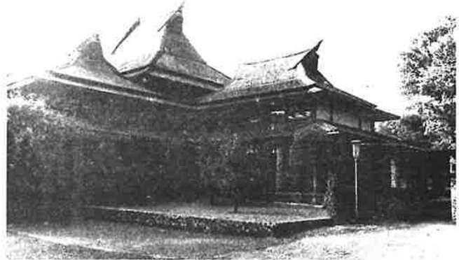
Aula Barat (West Hall) in Bandung Institute of Technology campus, built around 1920 by Maclaine Pont
