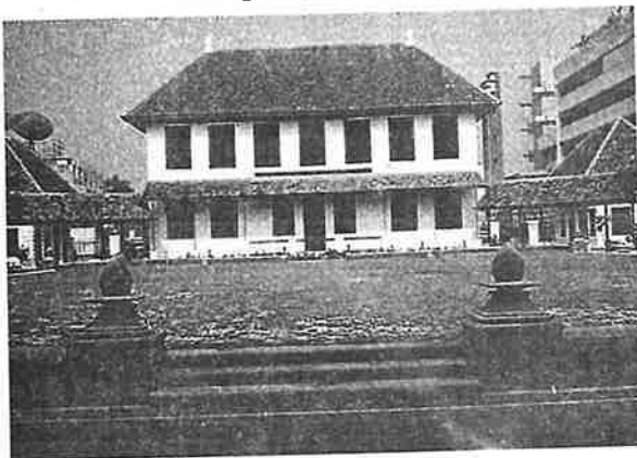
Gedung Arsip Nasional after the renovation
