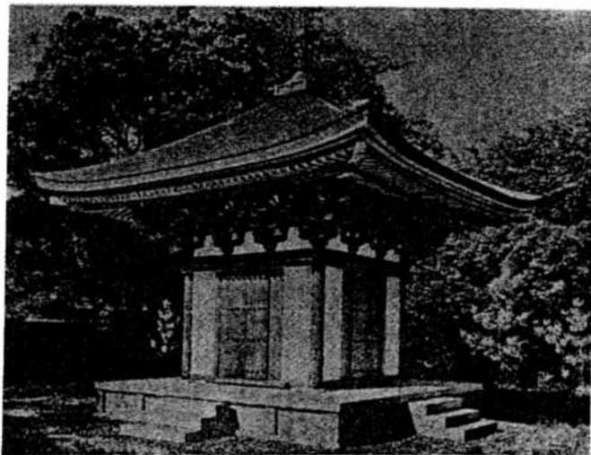
Fig. 5. Hall of Rakando of the Horyuji Temple (after restoration)
