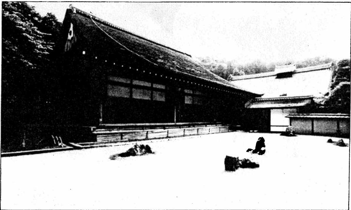
16. RYOAN-JI GARDEN AND HONDO, originally an aristocratic villa, turned into a Zen temple in 1488. Hondo was rebuilt in 1797 reusing another temple's structure of 1606.
