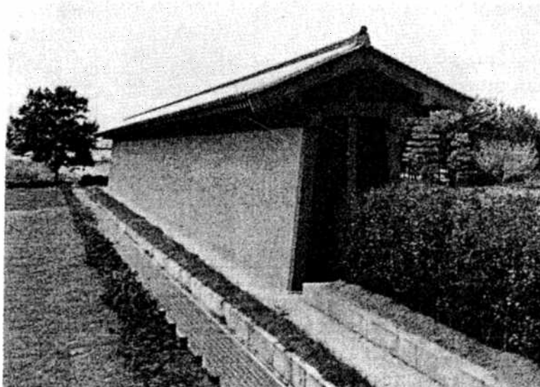
Fig. 6. Reconstruction of a portion of the Great Wall surrounding Nara Palace. The Great Wall was 2.7 m thick and probably more than 6m high.
