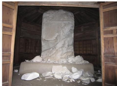
Figure 2.37 Damaged Kodokan stone monument due to the earthquake
