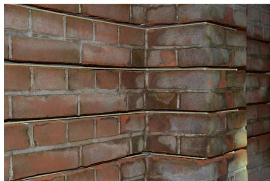
Figure 2.6 Mortar joints of the brickwork were removed to insert aramid fiber for reinforcement
