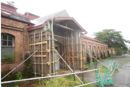
Figure 2.26 Damage to the brick counterfort and its emergency treatment
