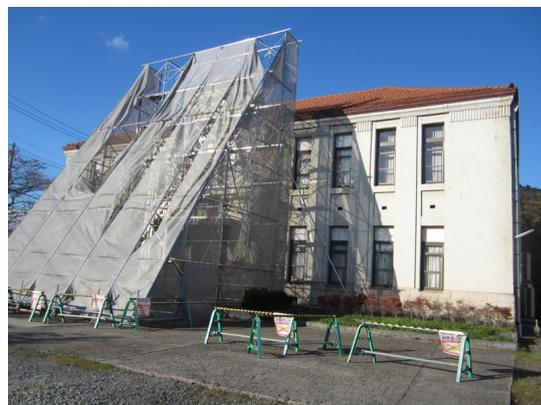
Figure 2.21 Temporary scaffoldings were erected to prevent further fall of the pediment
