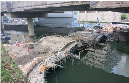
Figure 2.29 Dismantling of the bridge
