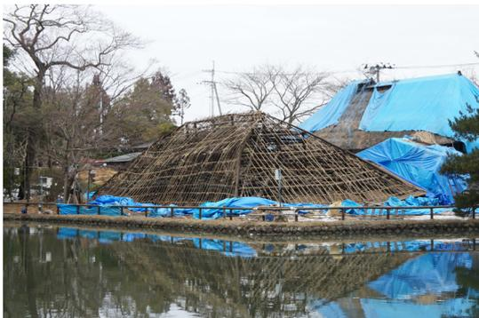
Figure 2.7 Dismantlement of the roof
