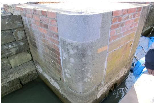
Figure 2.33 Repairs on bricks and stone blocks
