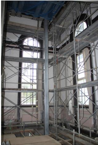
Figure 2.4 Interior steel frame reinforcement of the Assembly Hall: Steel columns of 200-millimeter square were installed in the four corners
