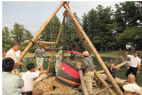
Figure 4.2 Hoisting the standing rock
