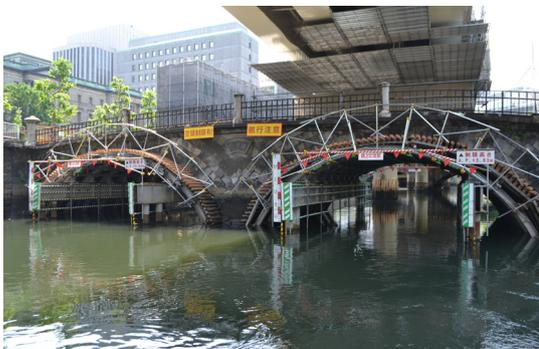
Figure 2.28 Construction of the temporary timbering
