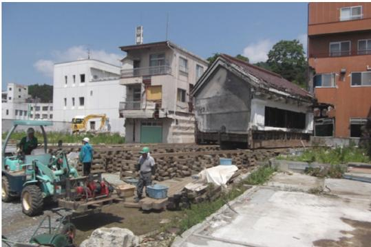
Figure 2.14 Kadoboshi Store was pulled back to its original location, employing a traditional relocation method
