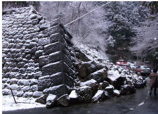
Figure 2.34 The northeastern wall of principal compound, immediately after the earthquake (taken on 2011/3/11)
