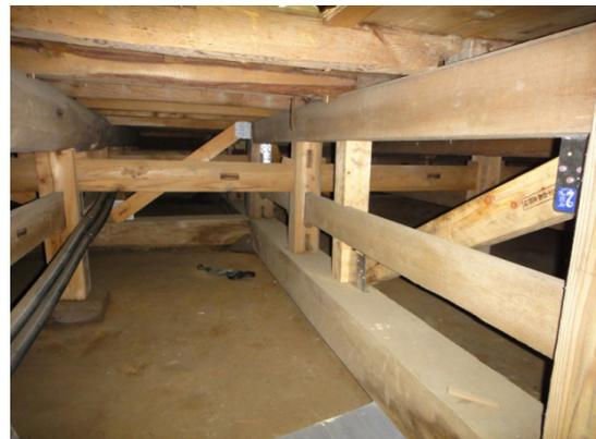
Figure 2.2 Braces were introduced for reinforcement into the extant floor structure of buildings in the left photo
