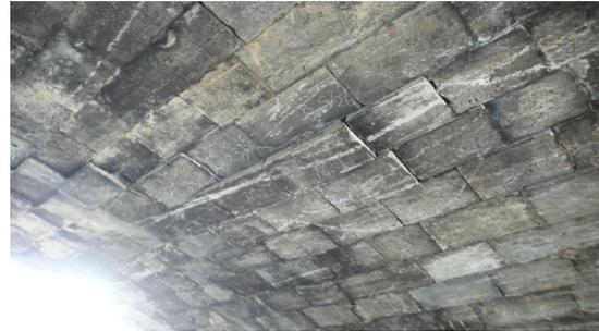
Figure 2.30 Bulging of the arch stones
