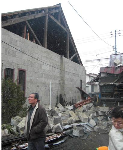
Figure 2.22 The collapse of the stone wall caused by the earthquake
