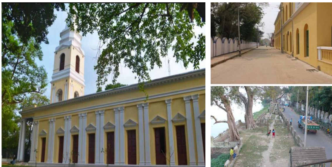
Fig.1. (Left) St. Olav's Church, restored; (Right Top) Citizen's view of the restored heritage precinct; (Right Bottom) The restored riverfront is now a recreational area frequented by locals.
