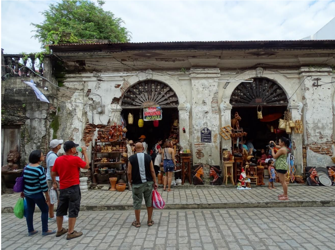
Fig.2: Many of the old houses in Vigan are in poor condition and are rented out for souvenir shops
