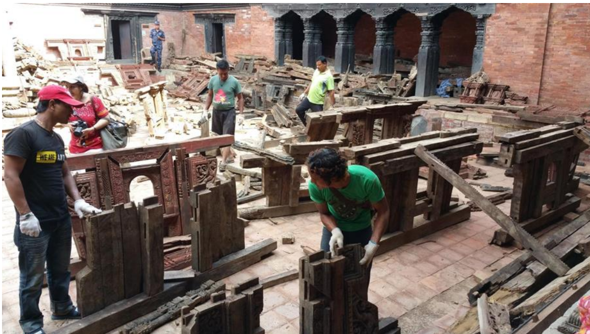
Fig.4: Engaging local craftsmen in post disaster recovery, Kathmandu
