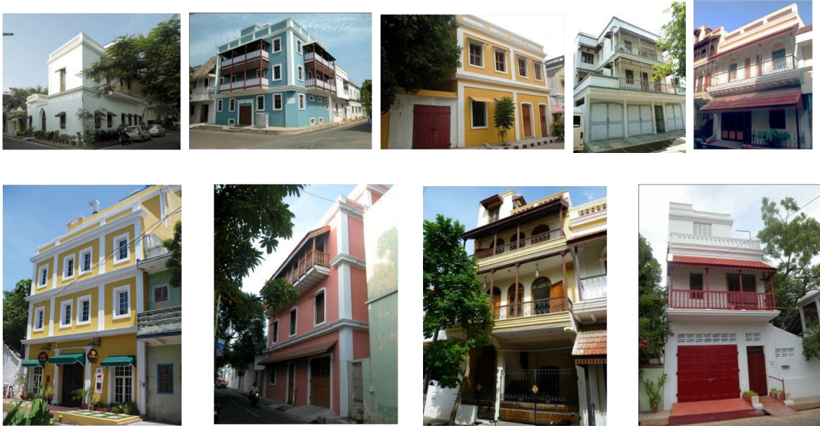
Fig.3: Façade Control became acceptable after many received grants during Vysial Street Façade Restoration project. Courtesy: INTACH, Pondicherry chapter, and PONDYCAN
