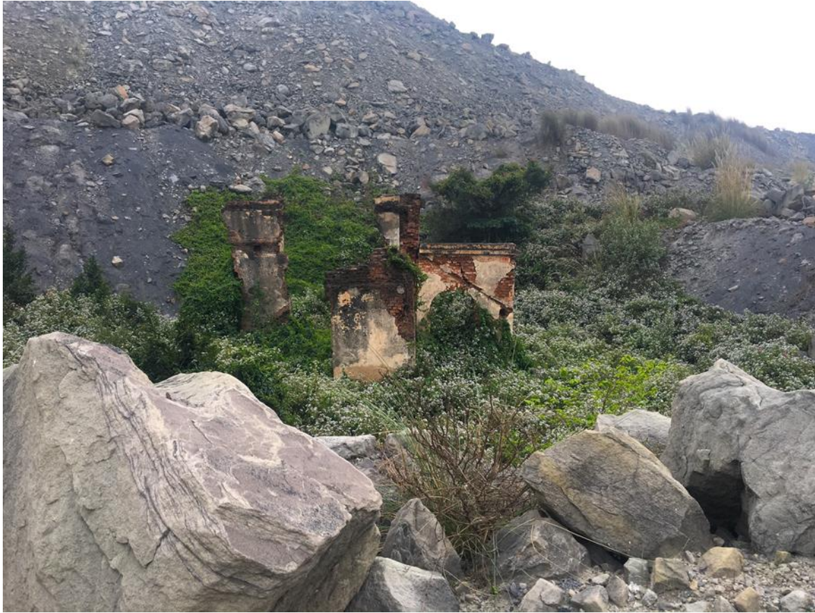
Fig.4: Remains of Tagore Bungalow at Narankoori, engulfed by a mining pit except the three walls, which are saved by the efforts of the local villagers (2020). Courtesy: Kamalika Bose.
