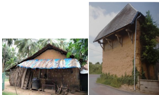
Fig. 4. Large overhangs built with local materials: [a] Goa – India (2019) [b] Normandy – France (Source: Patte, Architectures En Terre )
