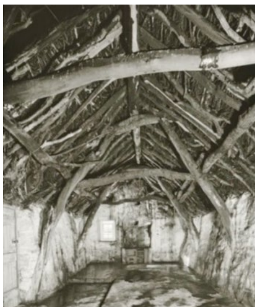
Fig. 3. Cruck framed roofs ensured the stability of roofs, Dumfriesshire – Scotland (Source: Walker, McGregor, Conservation of Vernacular Buildings)
