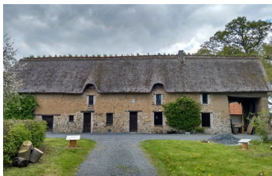
Fig. 5. Plants on roof ridge protected buildings from water damage, Maison des Marais in Normandy – France (2015)
