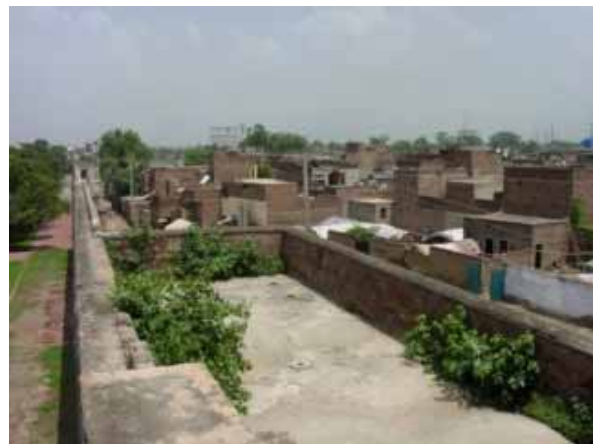
Fig 14. Modern constructions close to the wall of Shalamar.
