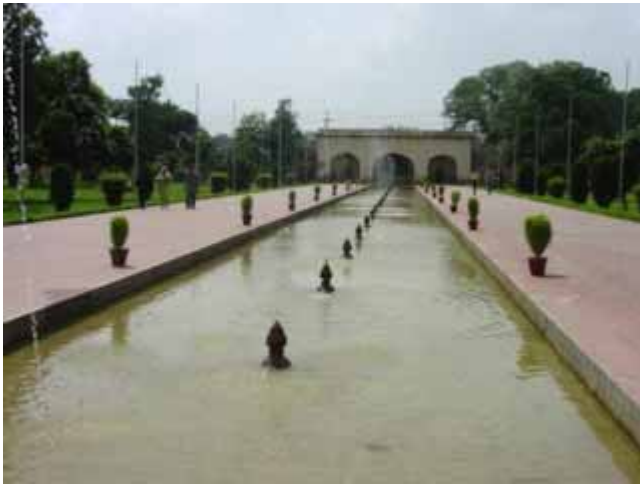
FIGURE 07. Shalamar. The central canal with fountains at the third terrace.
